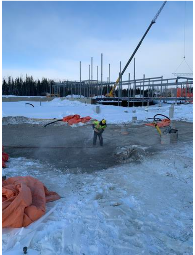
C2- Spreading water over backfilled area
