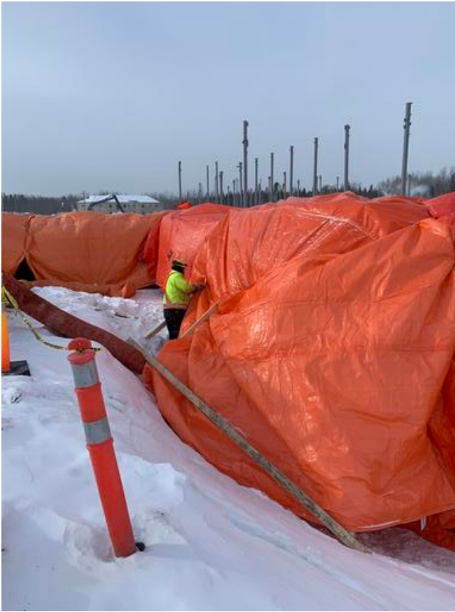
Modifying Hoarding for grade Beam (A2)
