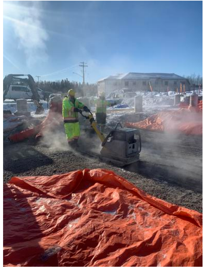
C2- Compacting backfill lift Arshdeep Grewal Feb 14, 2021 10:36 AM
