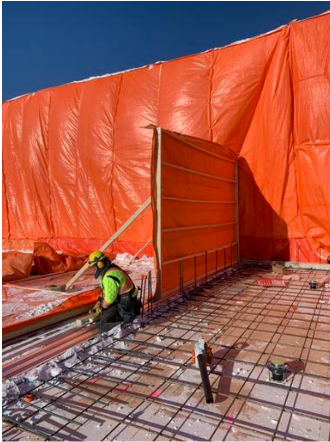
A1- Building hoarding for structural slab Arshdeep Grewal Feb 11, 2021 9:36 AM
