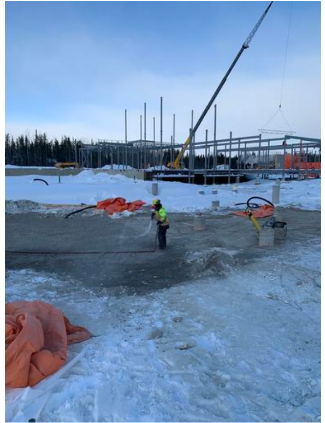
C2- Spreading water over backfilled area Arshdeep Grewal Feb 13, 2021 11:04 AM
