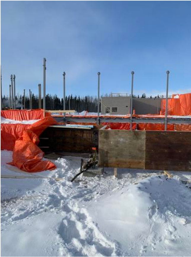
A2- Grade beam formwork Arshdeep Grewal Feb 13, 2021 11:04 AM
