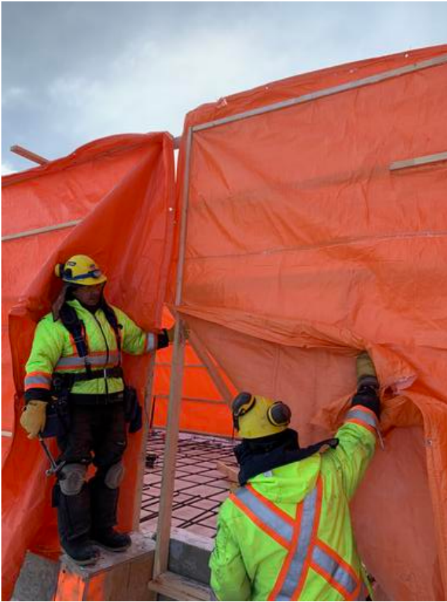
A1- Building hoarding for structural slab Arshdeep Grewal Feb 13, 2021 11:04 AM
