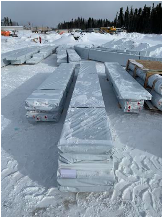
Glulam unloaded on-site Arshdeep Grewal Feb 9, 2021 3:08 PM
