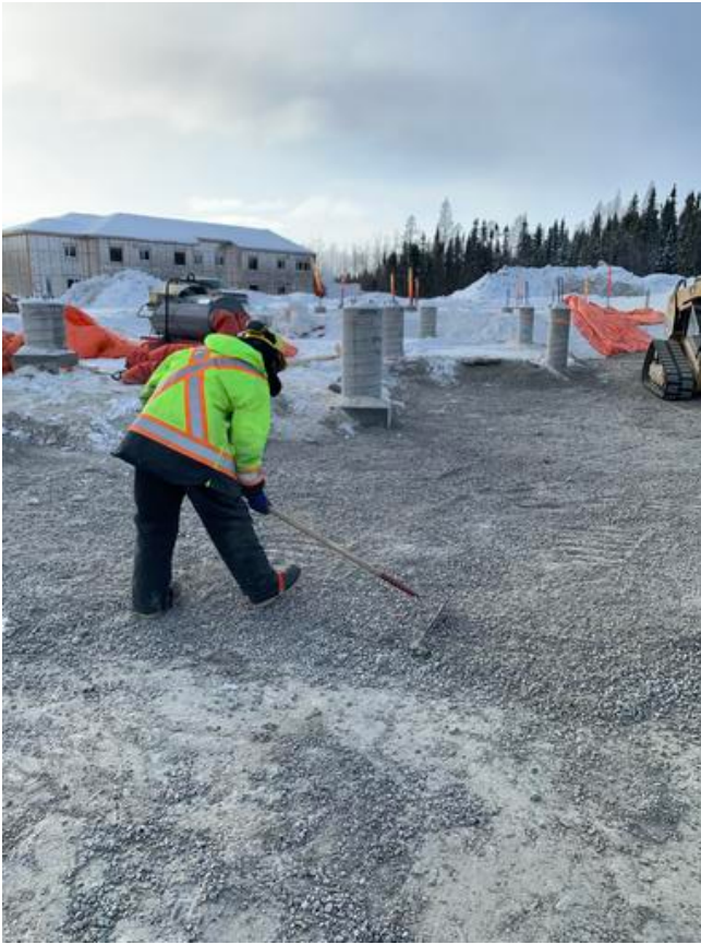
C2- Spreading backfill material Arshdeep Grewal Feb 13, 2021 11:04 AM
