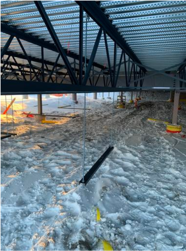
B1-Hangers installation under Q-Deck Arshdeep Grewal Feb 11, 2021 9:36 AM
