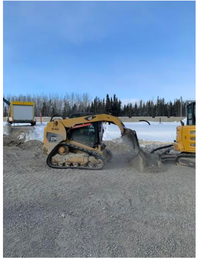
C2- Skidsteer placing backfill material Arshdeep Grewal Feb 13, 2021 11:04 AM
