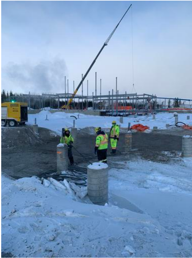
C2- Placing glycol loops over backfill lift Arshdeep Grewal Feb 13, 2021 11:04 AM
