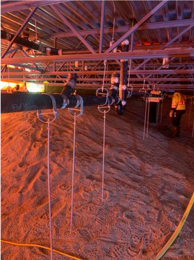
A1- Installing additional hangers near connection
