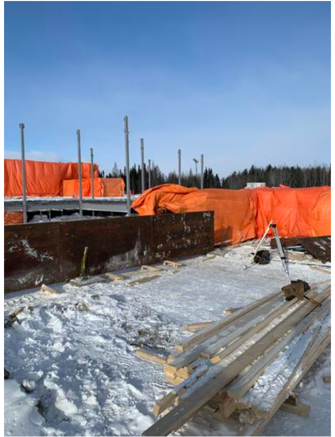
A2- Grade beam formwork Arshdeep Grewal Feb 13, 2021 11:04 AM
