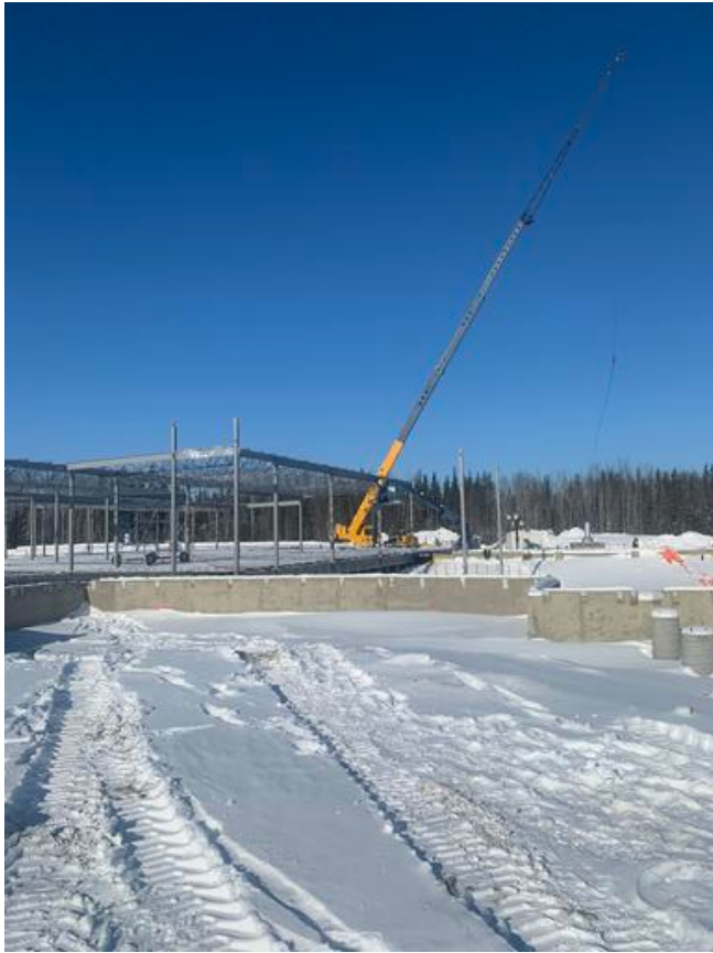
B1- Erection of roof structure
