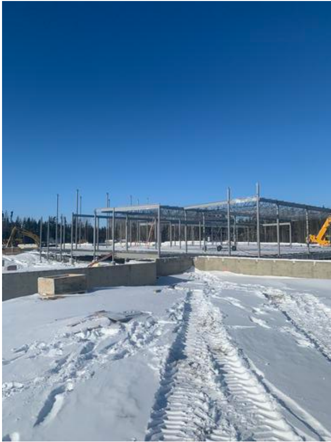
B1- Erection of roof structure Arshdeep Grewal Feb 14, 2021 10:36 AM
