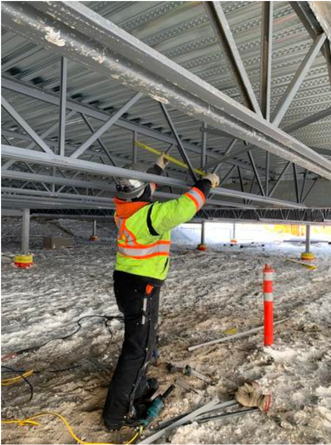
B1- Cross-bridging steel joist Arshdeep Grewal Feb 13, 2021 11:04 AM
