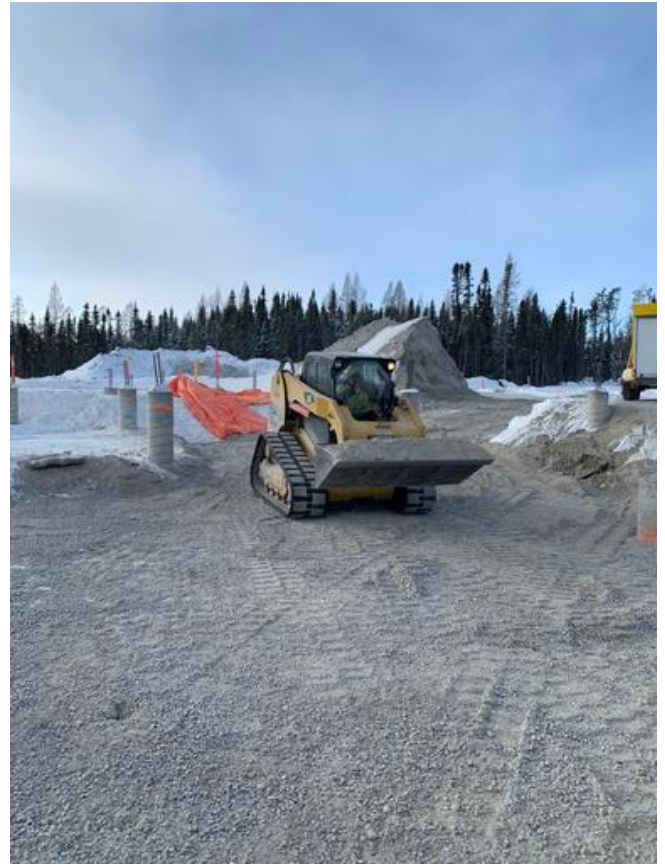
C2- Hauling backfill material from stockpile Arshdeep Grewal Feb 13, 2021 11:04 AM
