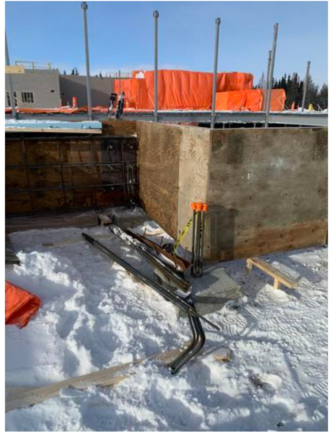
A2- Placing rebar for Grade Beam Arshdeep Grewal Feb 13, 2021 11:04 AM
