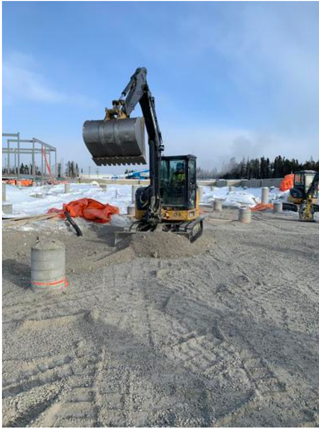
C2- Spreading backfill material by Mini Excavator Arshdeep Grewal Feb 13, 2021 11:04 AM
