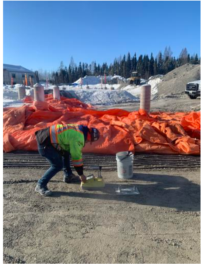
C2- M.Block testing backfill lift Arshdeep Grewal Feb 14, 2021 10:36 AM
