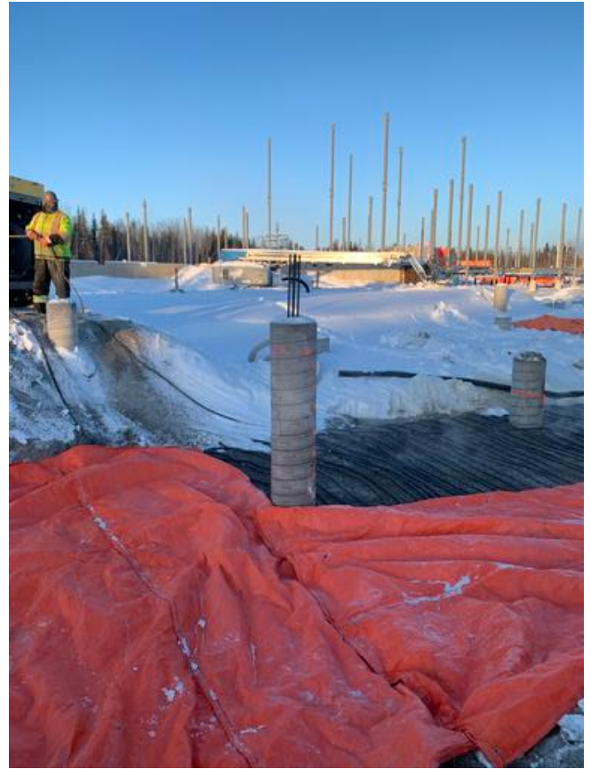
C2- Placing tarps over glycol loops Arshdeep Grewal Feb 11, 2021 9:36 AM
