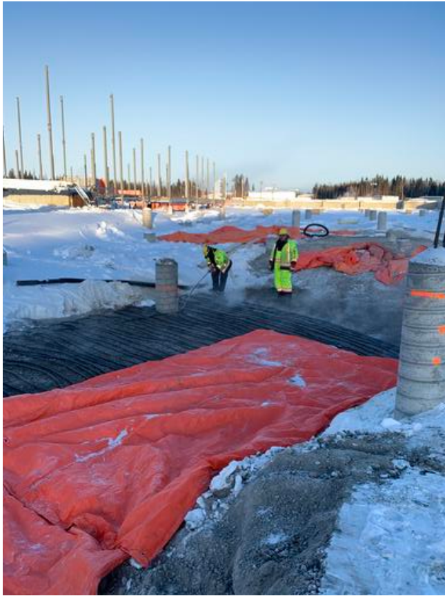
C2- Placing glycol loops for heating backfill Arshdeep Grewal Feb 11, 2021 9:36 AM
