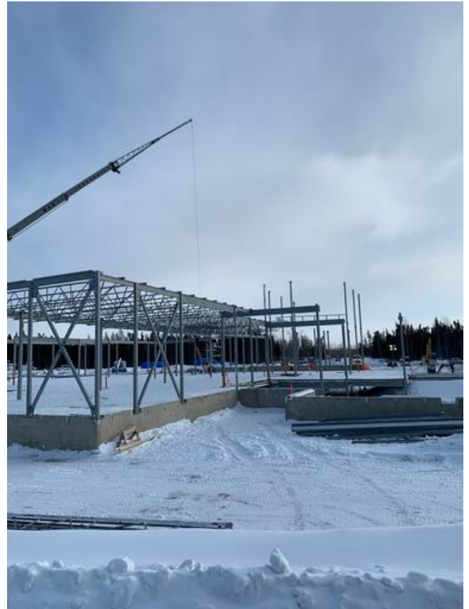
B1- Erection of roof structure Arshdeep Grewal Feb 13, 2021 11:04 AM
