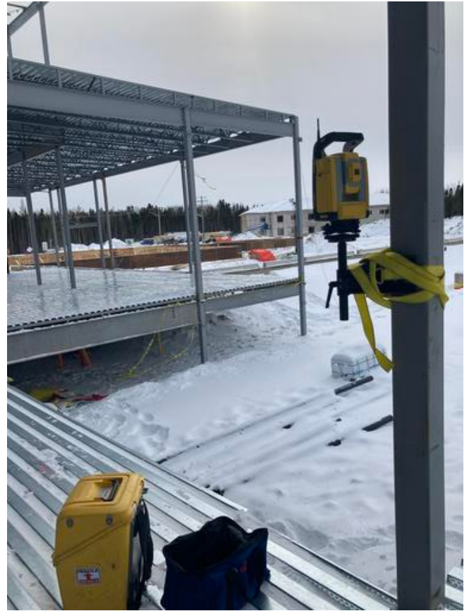
surveying for layout of sleeves and hangers B1 Anmol Kang Mar 1, 2021 4:10 PM
