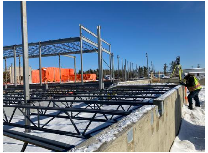
Laying out new control points Anmol Kang Mar 4, 2021 4:55 PM
