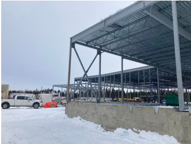
Q deck B1 roof level
