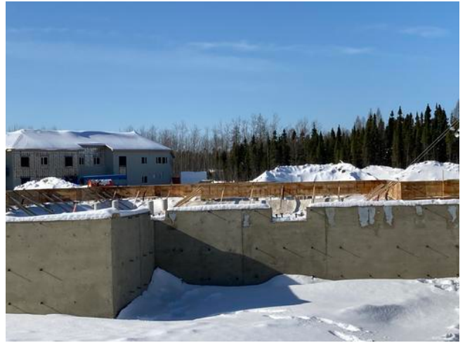
Grade beam C2 form work
