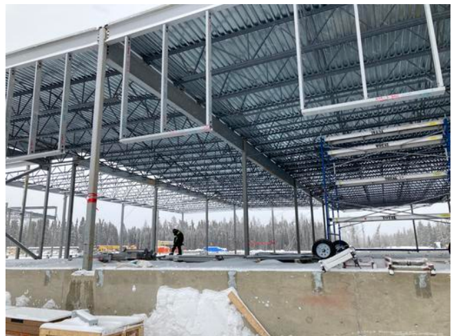
Q deck B1 roof level
