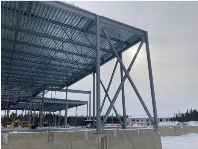
Q deck B1 roof level Anmol Kang Mar 1, 2021 4:11 PM
