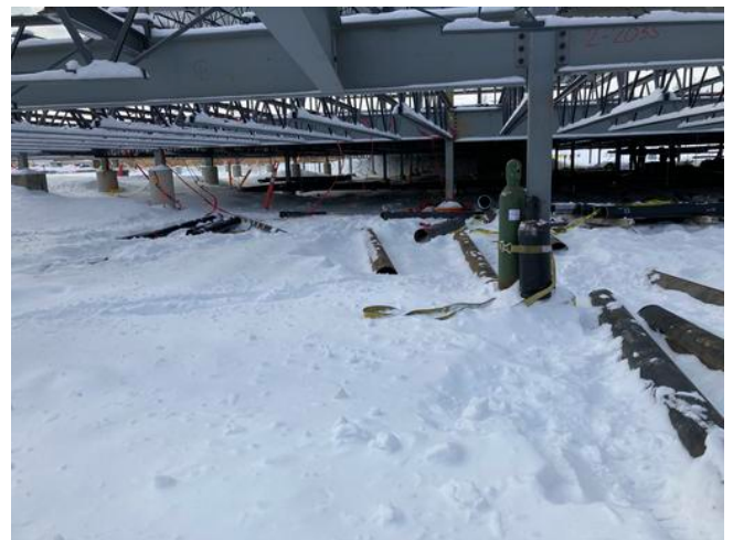
Preparation for B1 piping in crawl space
