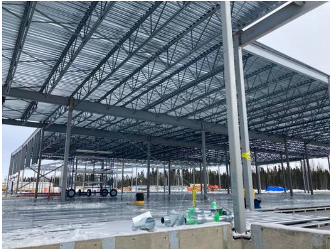
Q deck B1 roof level Anmol Kang Mar 1, 2021 3:44 PM
