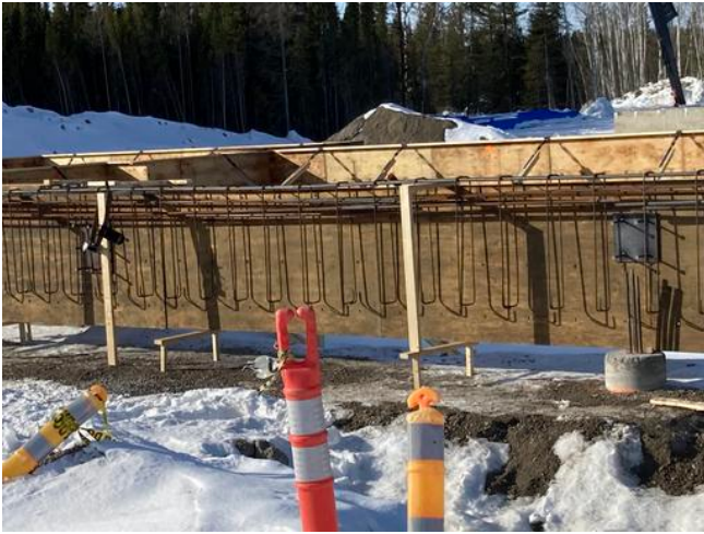
Rebaring grade beam Anmol Kang Mar 5, 2021 4:28 PM
