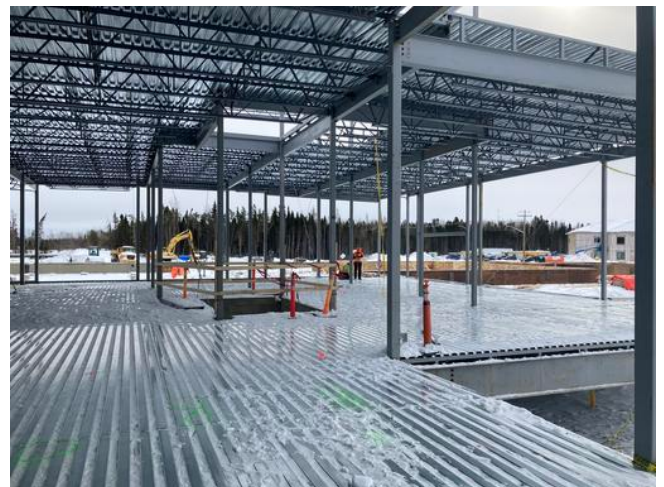
Q deck B1 Roof level and floor level
