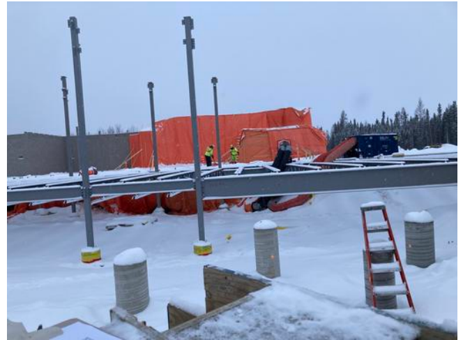
Heating and hoarding over masonry A1
