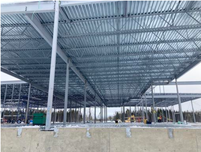
Q deck B1 roof level
