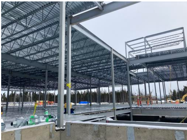
Penthouse steel structure Anmol Kang Mar 1, 2021 3:43 PM
