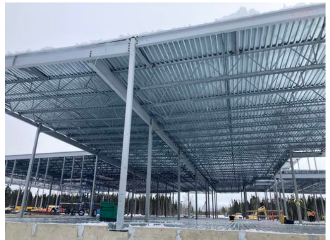
Q deck B1 roof level Anmol Kang Mar 1, 2021 3:43 PM
