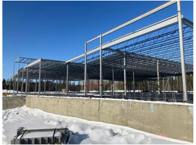
Steel Structure B1 and A3
