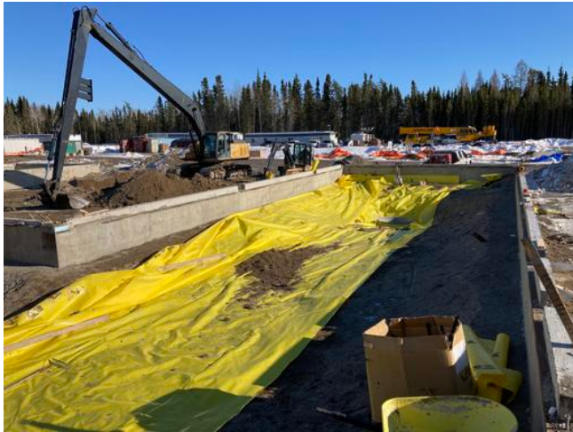
A2- Placing poly membrane Anmol Kang Mar 13, 2021 5:38 PM
