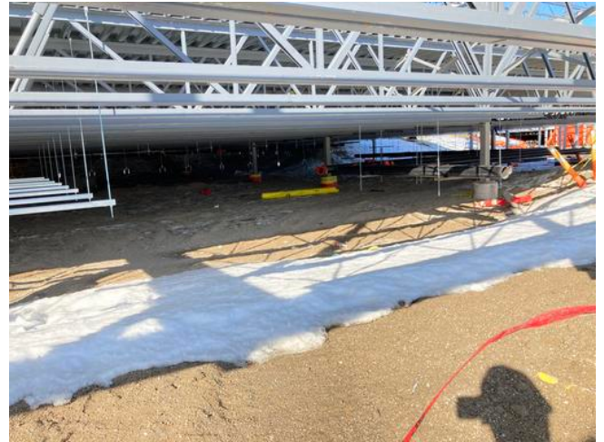
B1- Installing hangers / pipes in crawlspace
