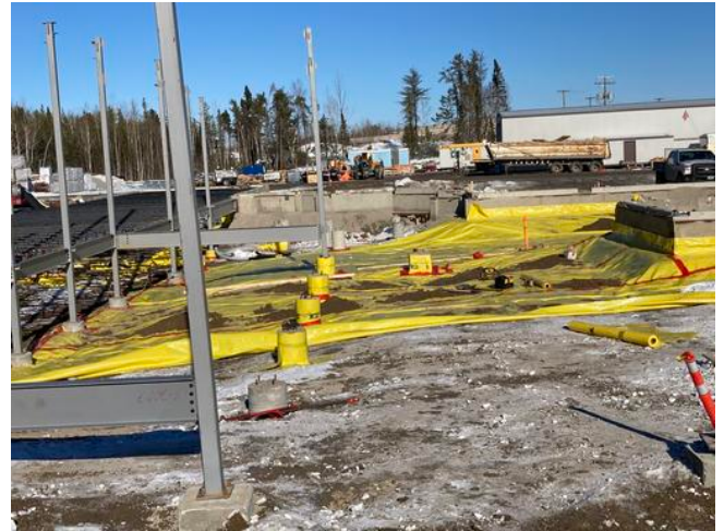
Laying sand over poly in A2
