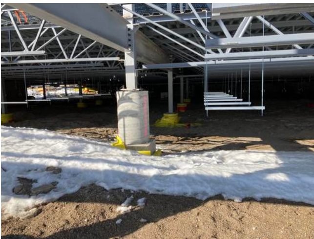
B1- Installing hangers in crawlspace
