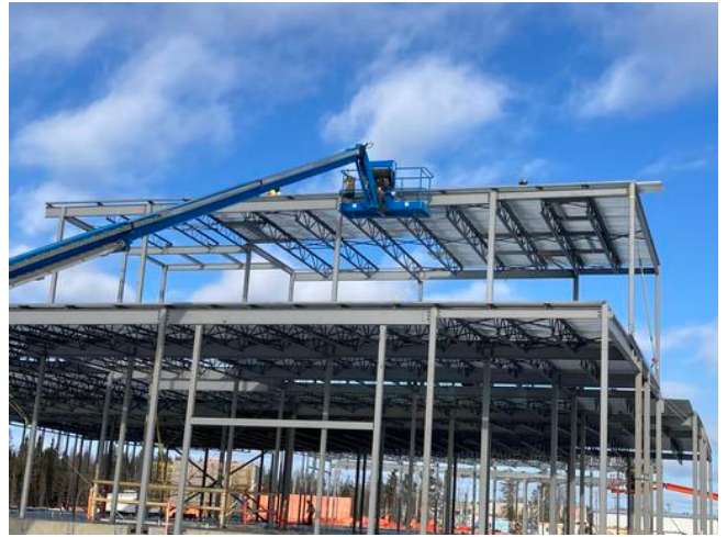
Penthouse Qdeck work in progress
