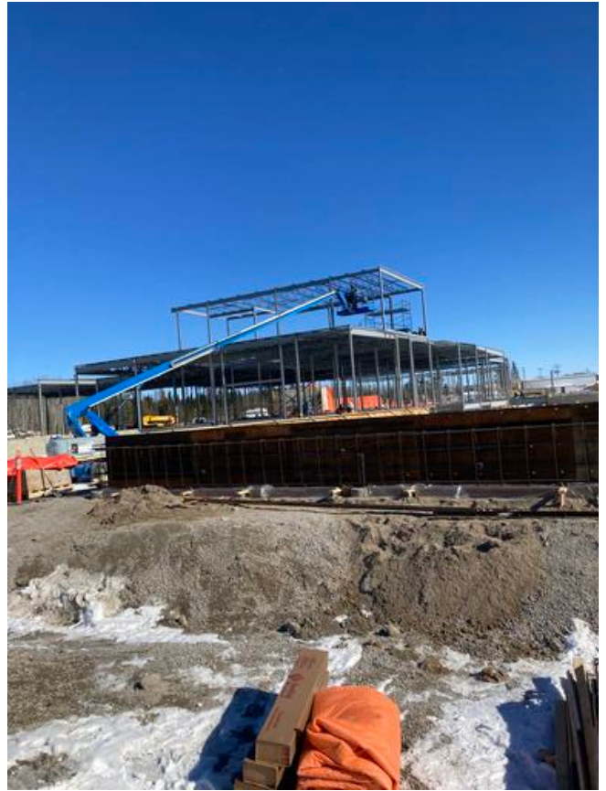
C2 grade beam work in progress
