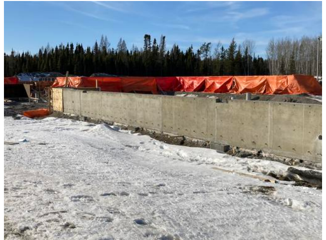
C2- Building hoarding for grade beam
