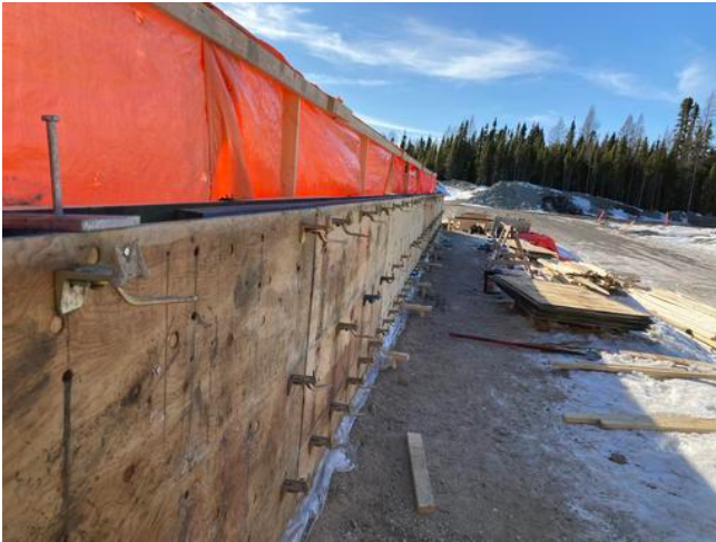
C2- Buttoning up grade beam
