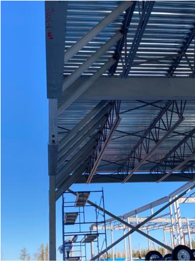
B1- Hangers installation with diagonal bracing
