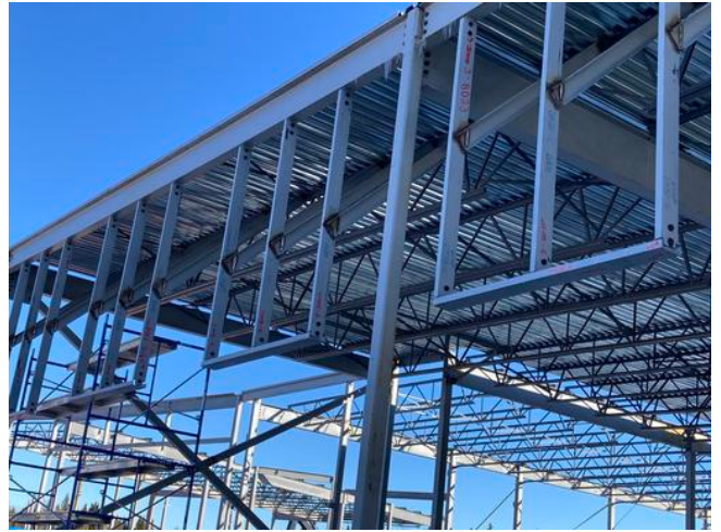
B1- Hangers installation with diagonal bracing
