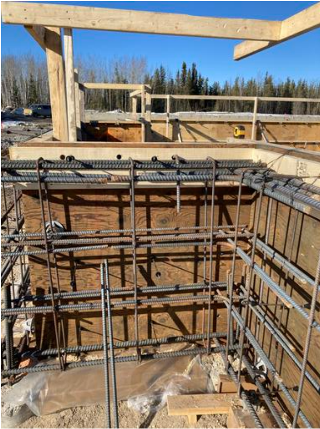
C2- Grade beam rebar
