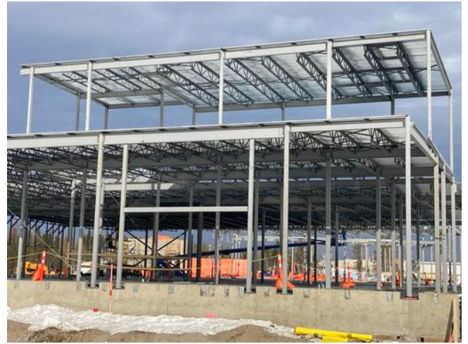
Qdeck work complete for penthouse over B1 Anmol Kang Mar 12, 2021 5:43 PM
