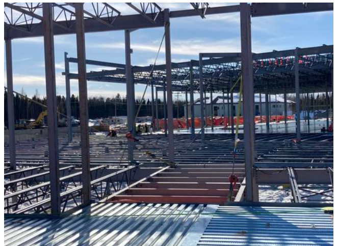
A3- Straightening structural steel
