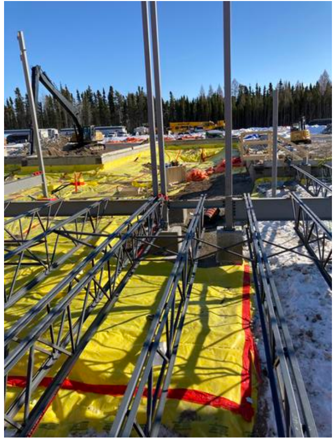
A2- Placing sand over poly membrane
