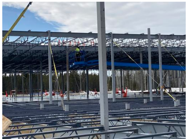
Installing supports for glulam in A3 Anmol Kang Mar 12, 2021 5:43 PM
