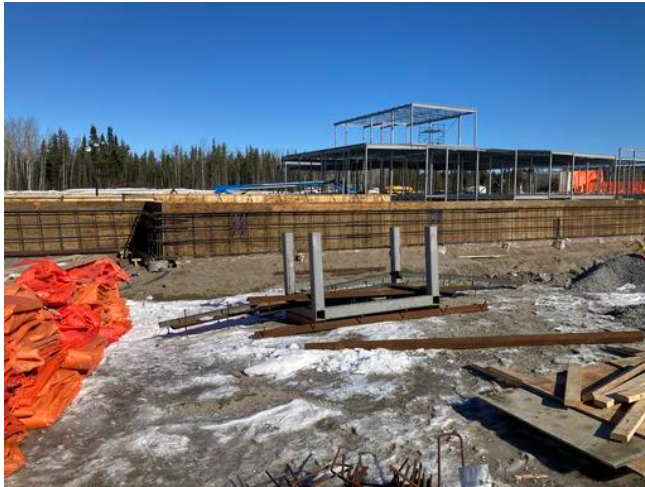
C2 grade beam work in progress
