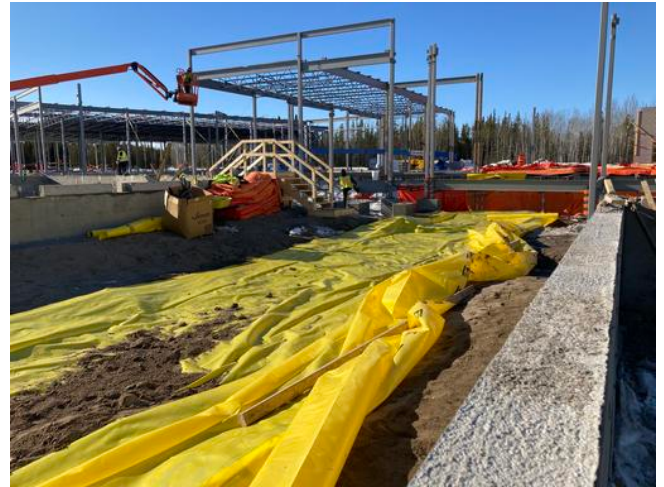
A2- Placing poly membrane
