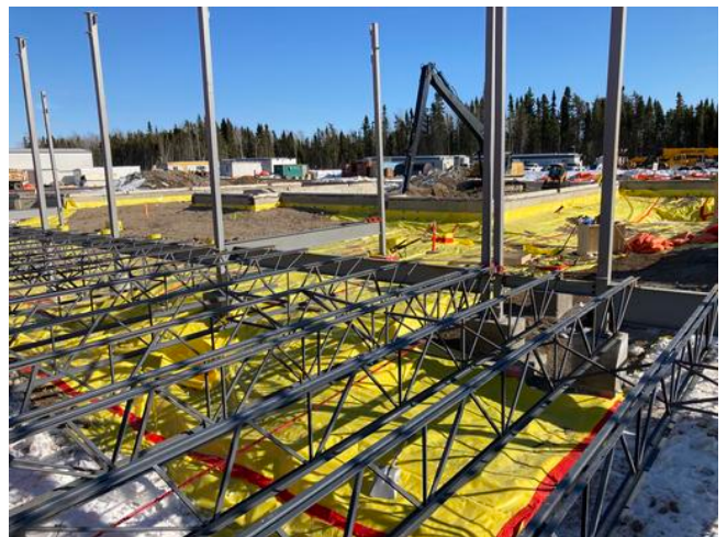
A2- Placing sand over poly membrane
