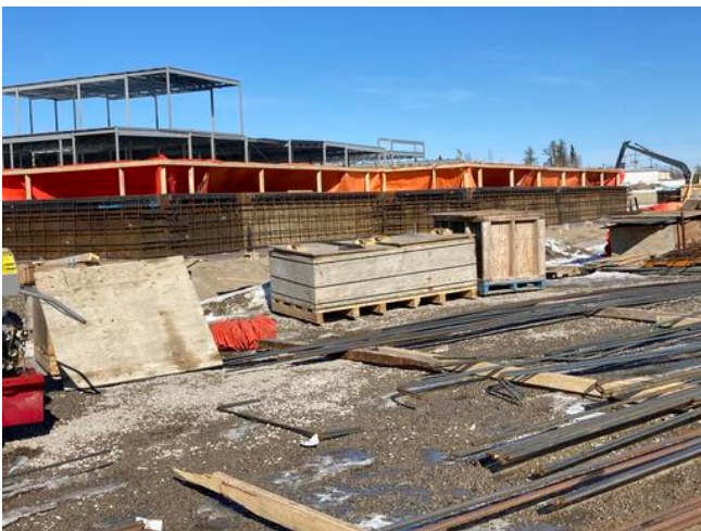
C2- Placing rebar for grade beam
