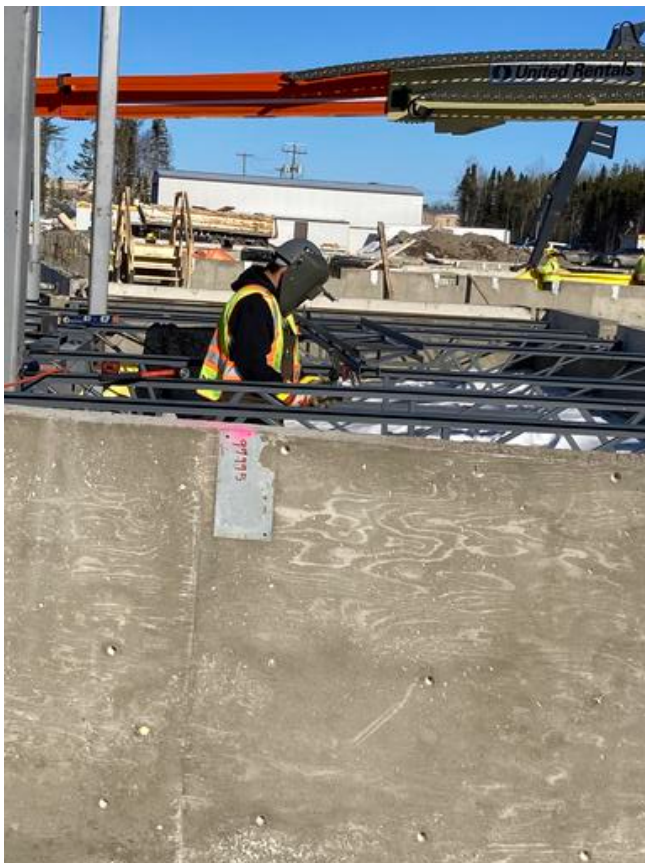
A3- Joist installation
