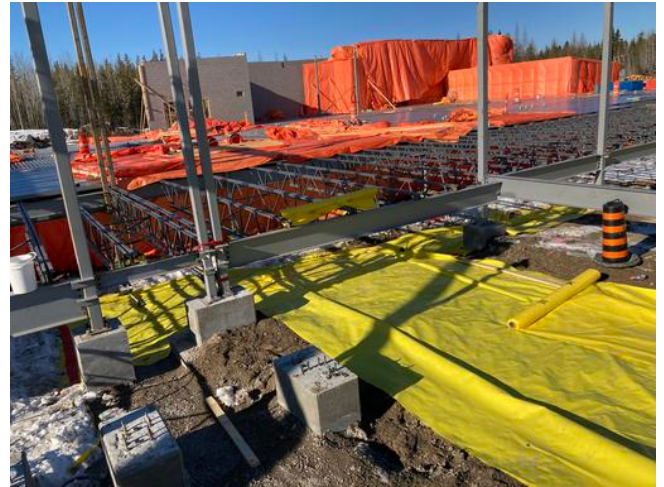
A2- Placing poly membrane
