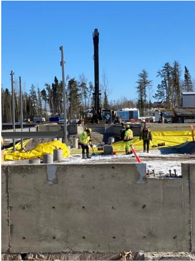
shoveling snow before laying poly in A2
