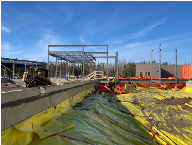
A2- Placing sand over poly membrane
