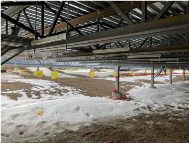
Installing hangers A1 crawlspace
