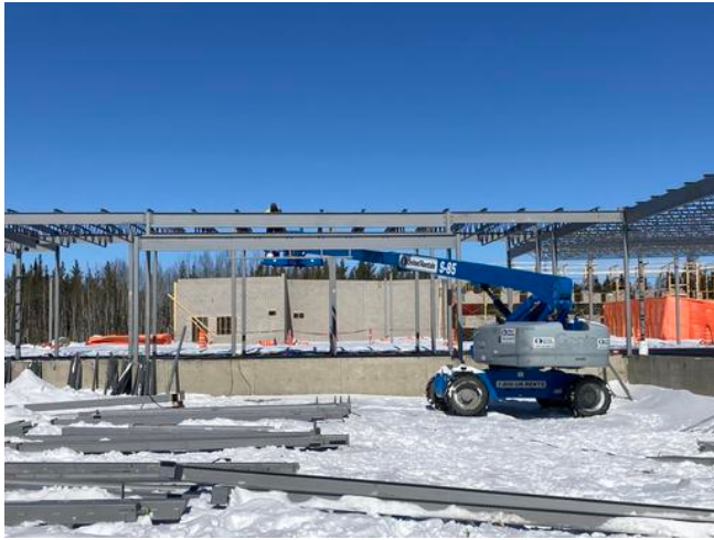
Straightening and torquing in A2
