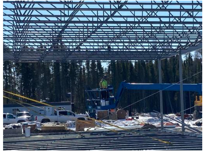
A2 cross bracing work in progress
