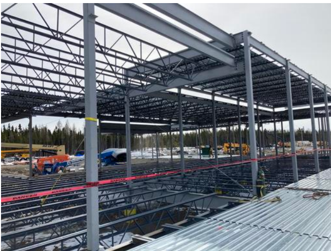
Laying sheets A2 roof level
