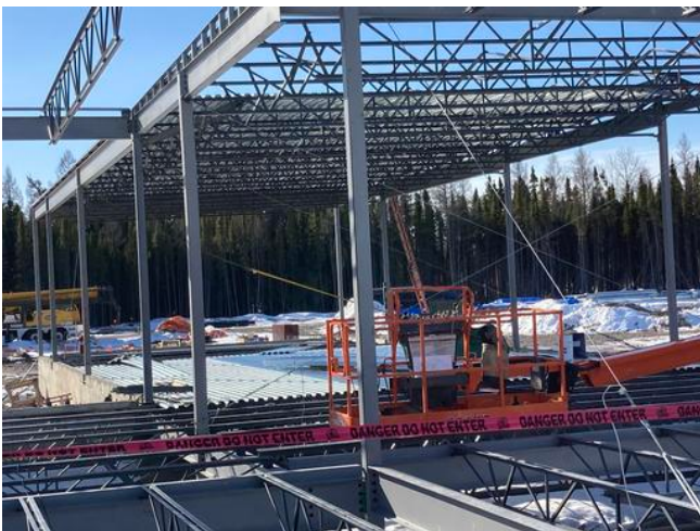
Straightening & Torqueing Steel structure A2
