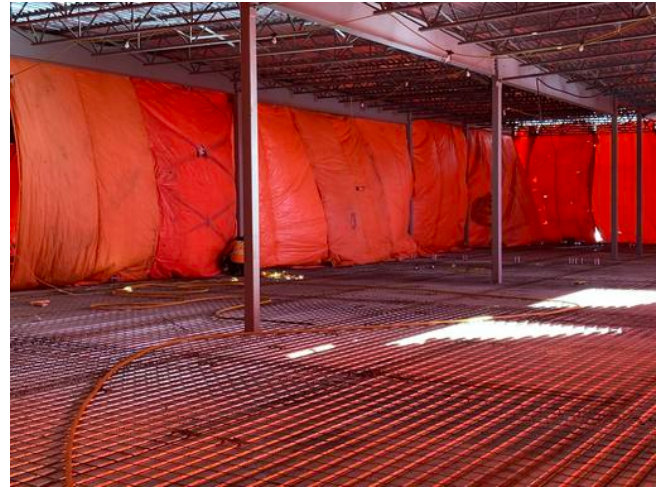
B1-2 mesh on Q deck
