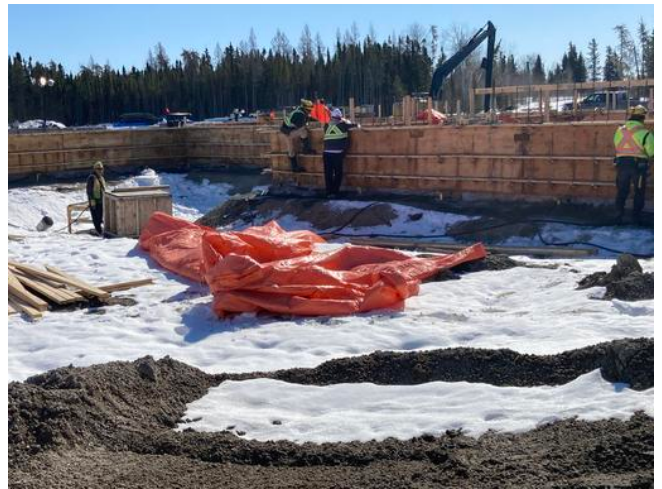
Formwork removal C2 grade beam
