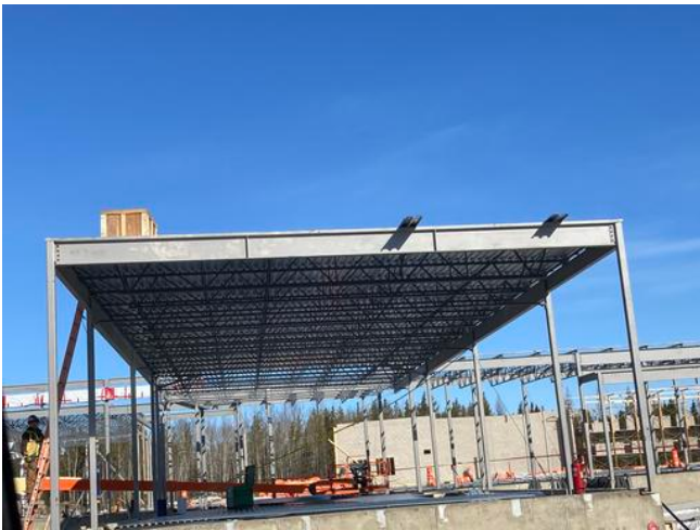
Laying deck sheets A2 roof level
