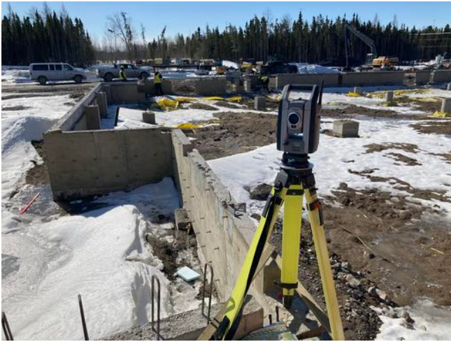
Setting up new control points
