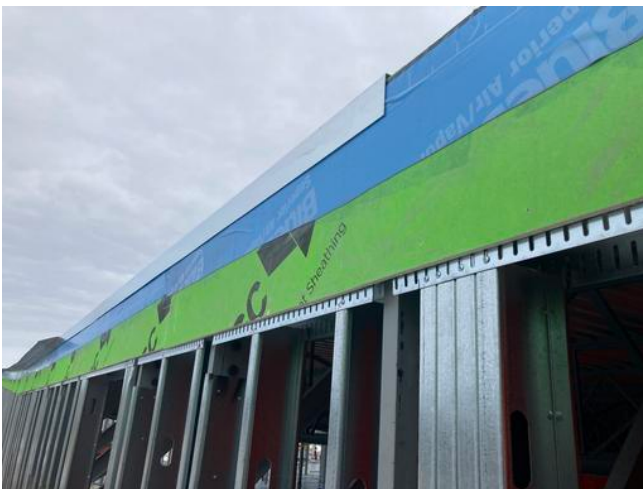
B1- Installing flashing & blue skin along wall Anmol Kang
