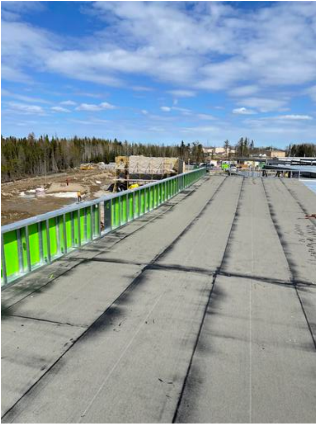
B1- Stud framing for parapet walls Arshdeep Grewal Apr 17, 2021 7:52 AM
