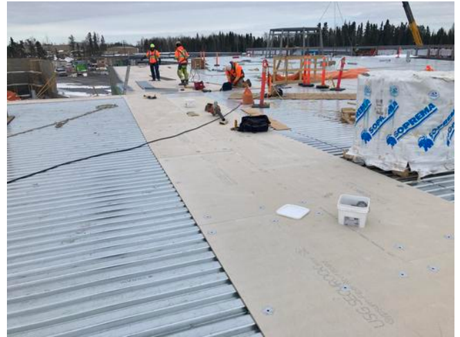
B1- Installing roof boards Anmol Kang
