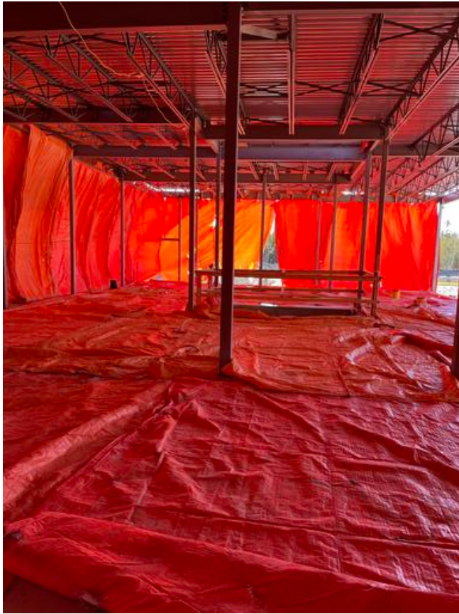
B1-2 - Tarps over poured concrete slab
