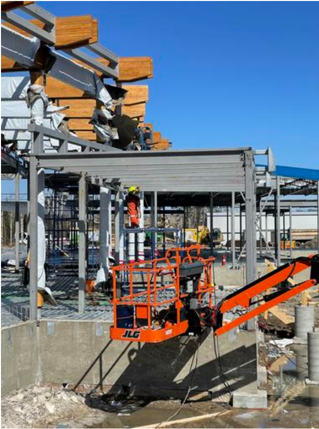
A3- Erection of Glulam Structure Arshdeep Grewal Apr 18, 2021 4:29 PM
