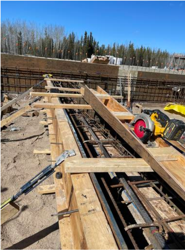
C2 - Building formwork & rebarring for Grade Beam Arshdeep Grewal Apr 18, 2021 4:29 PM
