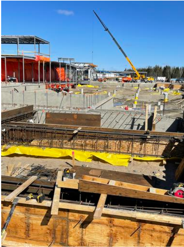
C2 - Placing rebar for Grade Beam Arshdeep Grewal Apr 18, 2021 4:29 PM
