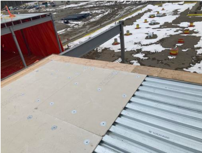
B1- Installed roof boards and plywood along edge Anmol Kang
