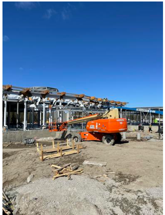
A3- Erection of Glulam Structure
