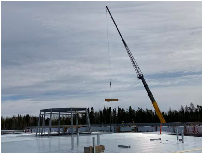
A3- Crane lifting Glulam piece
