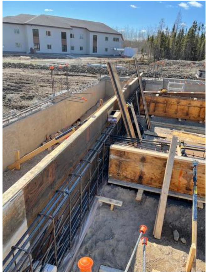
C2 - Formwork & rebar for Grade Beam Arshdeep Grewal Apr 18, 2021 4:29 PM
