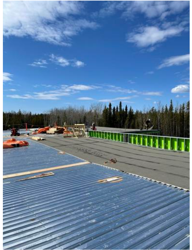
B1- Vapor barrier installed over dens deck
