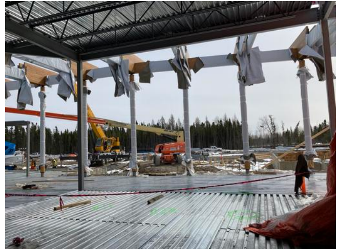
A3- Glulam Erection Anmol Kang Apr 15, 2021 4:54 PM
