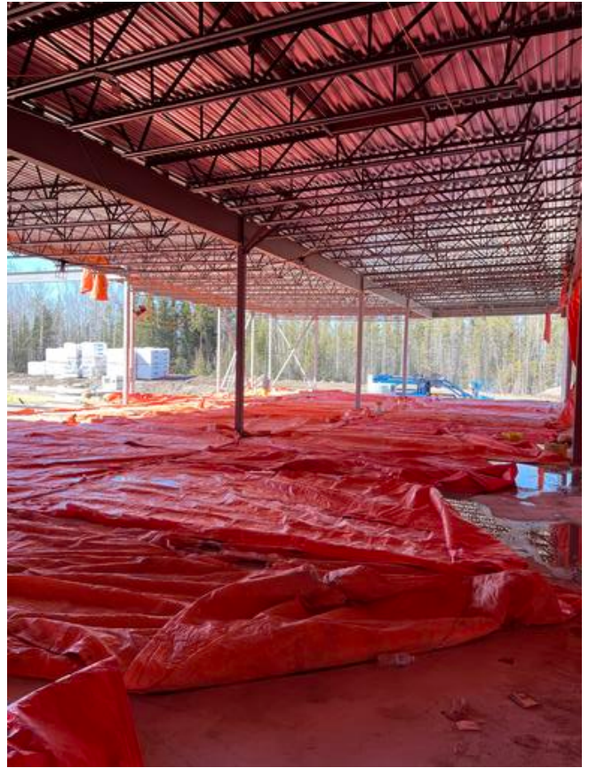
B1-2 - Placed tarps over concrete slab
