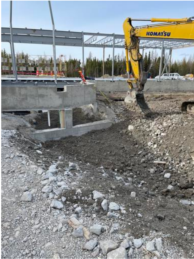
A2- Placing material over water main connection
