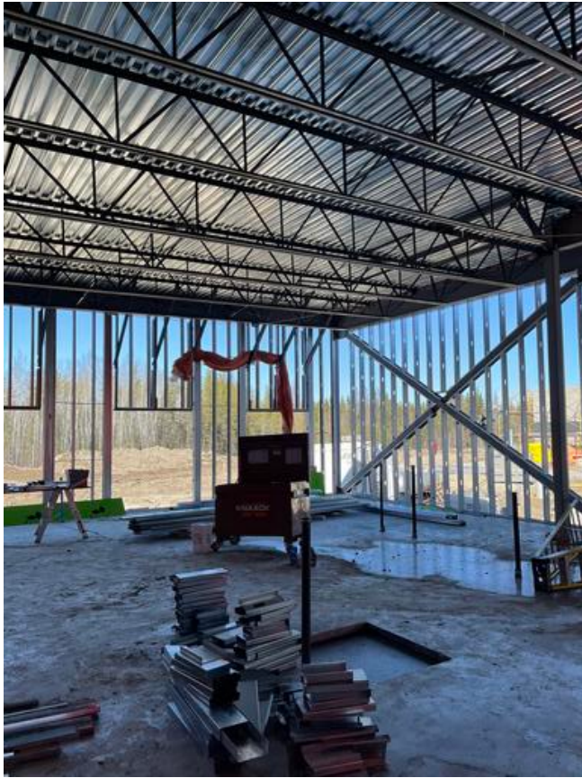
B1- Exterior steel stud framing Arshdeep Grewal Apr 18, 2021 4:29 PM
