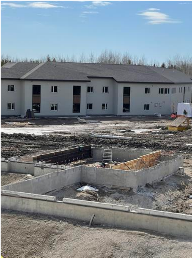
C2 Ambulances Garage - Building formwork for GB
