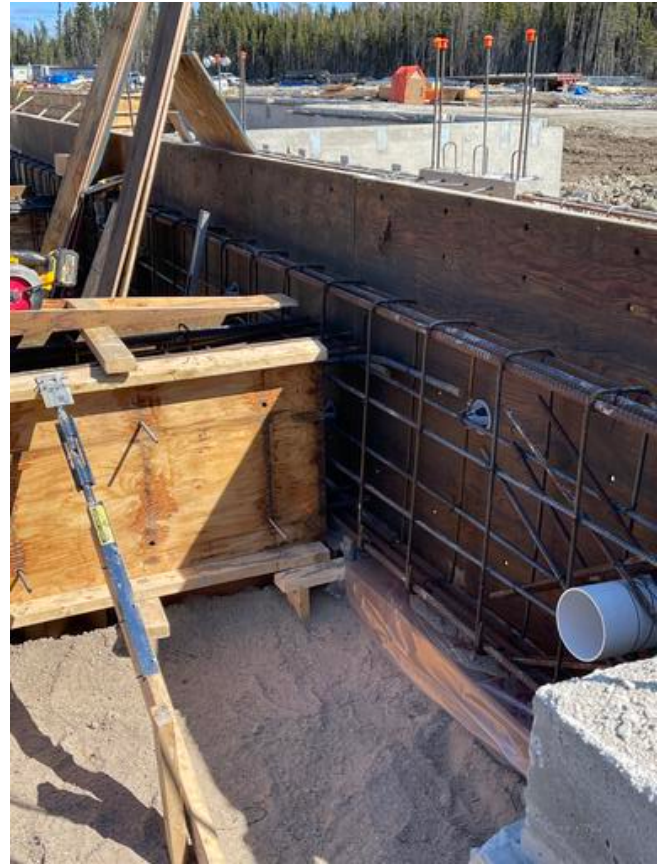
C2 - Rebar for Grade Beam Arshdeep Grewal Apr 18, 2021 4:29 PM
