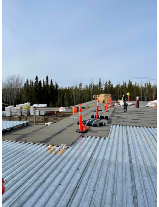
B1- Vapor barrier installed over deck
