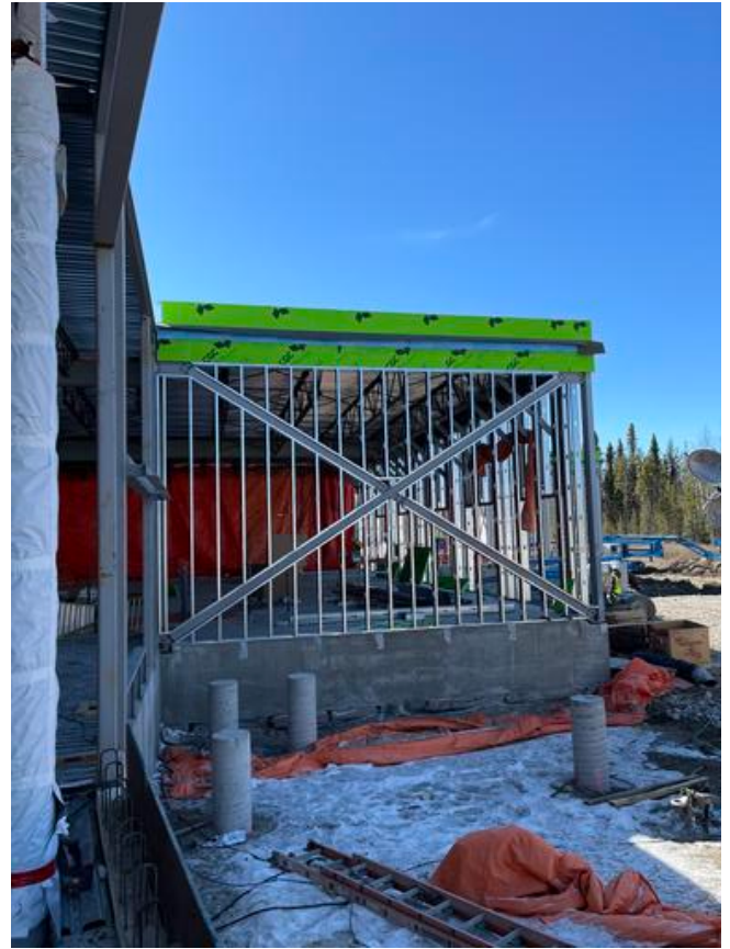
B1- Stud framing around cross bracing Arshdeep Grewal Apr 18, 2021 4:29 PM
