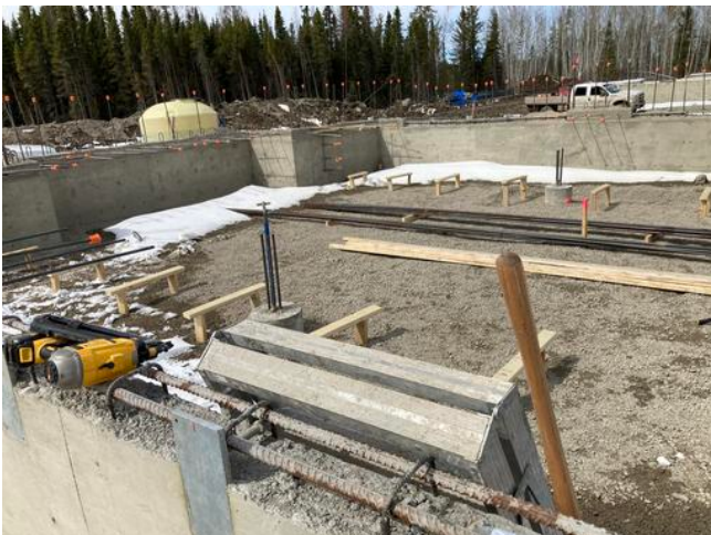
C2- Layout for grade beam Anmol Kang Apr 15, 2021 4:54 PM
