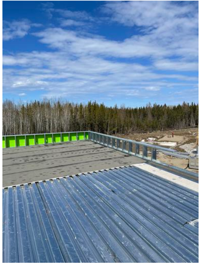
B1- Stud framing for parapet walls Arshdeep Grewal Apr 17, 2021 7:52 AM
