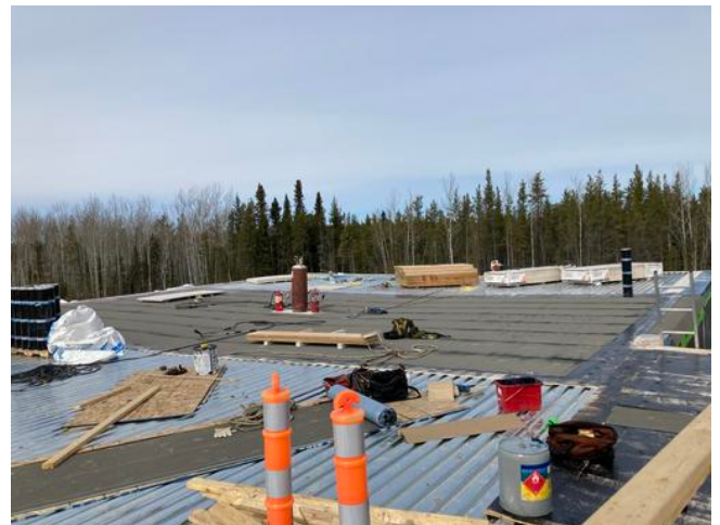
B1- Installing dens deck and vapor barrier Anmol Kang Apr 15, 2021 4:54 PM
