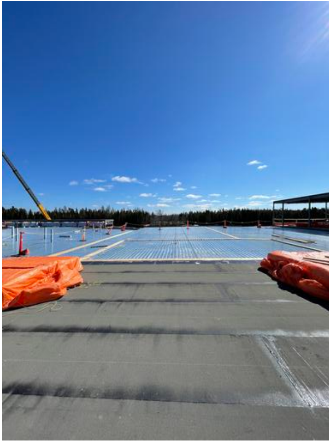
B1- Installing dens deck and vapor barrier Arshdeep Grewal Apr 18, 2021 4:29 PM
