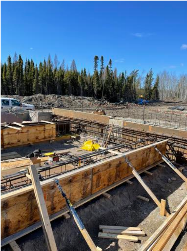
C2 - Formwork & rebar for Grade Beam Arshdeep Grewal Apr 18, 2021 4:29 PM
