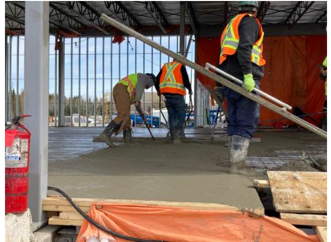
B1-2 - Placing concrete over Q-Deck
