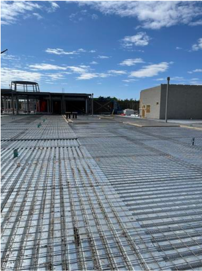
A1- Wire mesh over Q-deck Arshdeep Grewal Apr 17, 2021 7:52 AM
