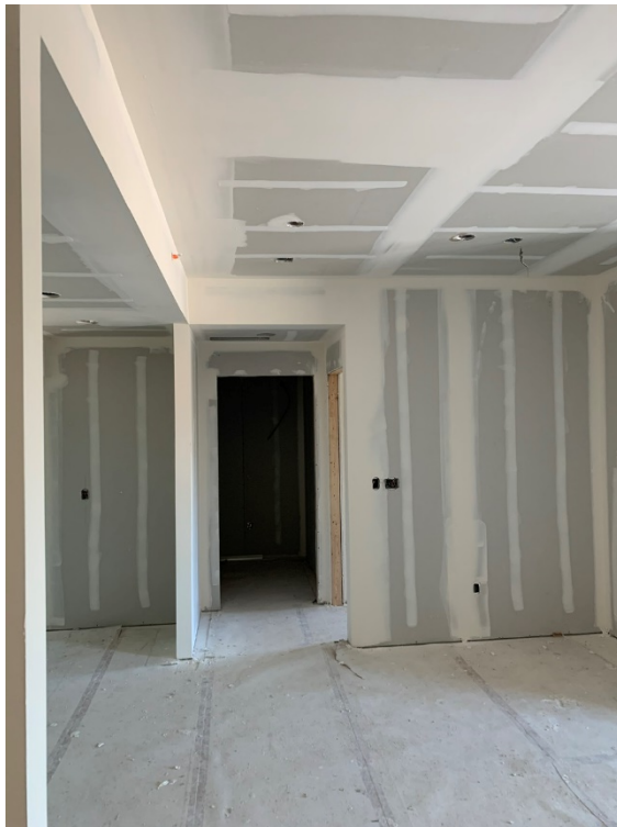
Wall/Ceiling Taping – LVL 2 East Wing
