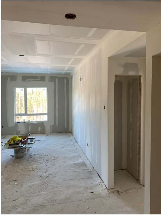
Taping Progress – LVL 2 East Wing
