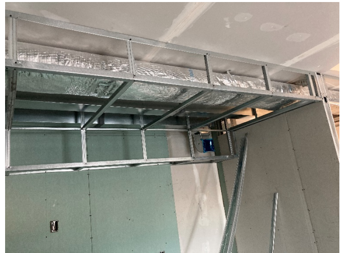
Bulkhead Framing – LVL 1
