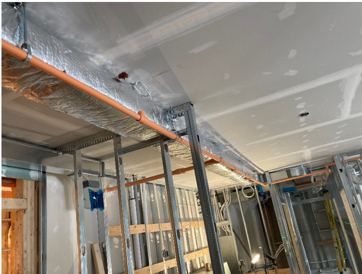
HVAC Installation – LVL 1
