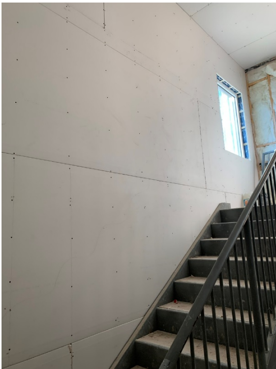
Gypsum Board – Stair # 2
