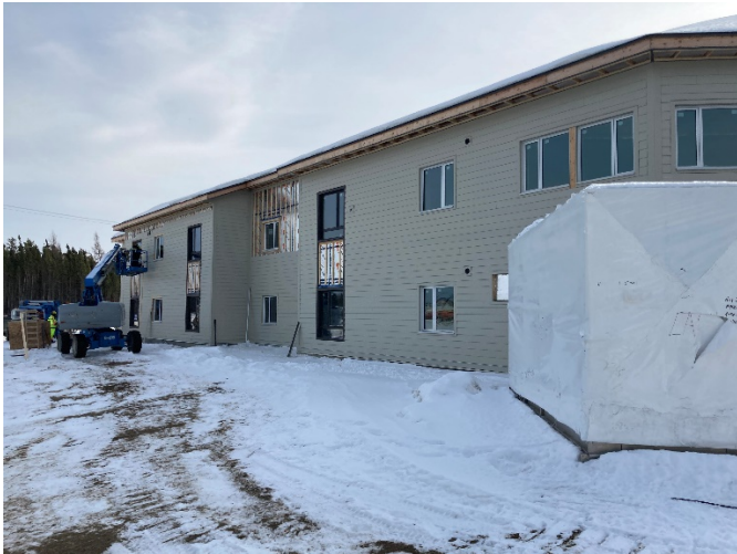
Fiber Cement Siding Install – North East
