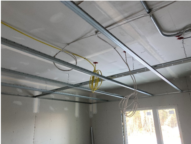
Suspended Ceiling – LVL 1
