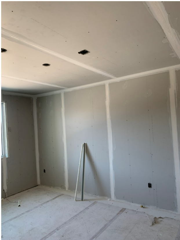
Taping Progress – LVL 2 West Wing
