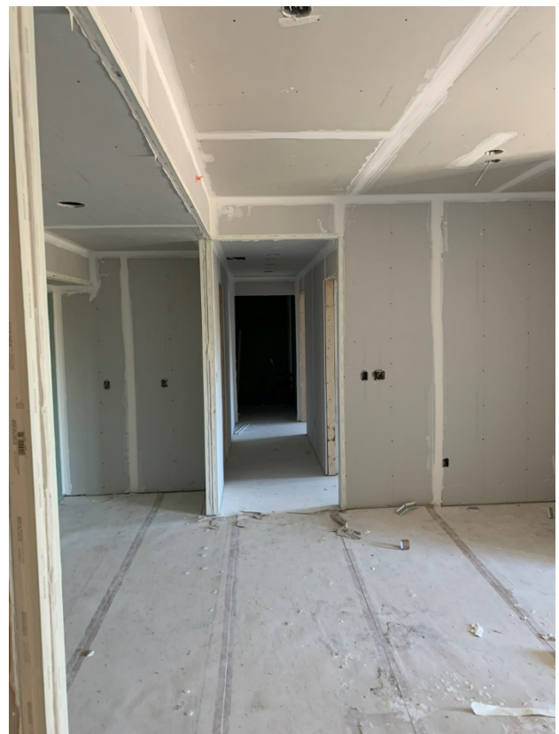
Taping Progress – LVL 2 West Wing
