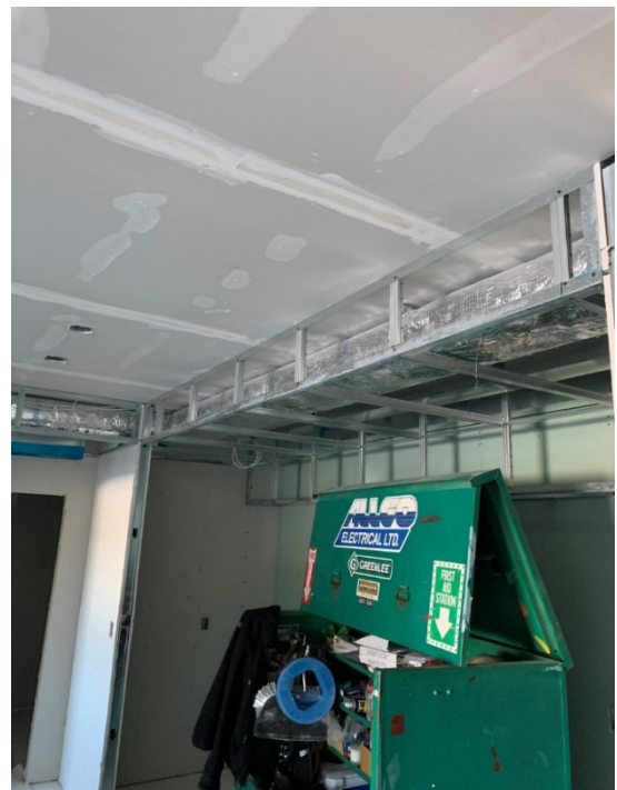
Ceiling Framing - LVL 1 East Wing
