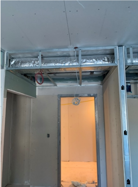
Ceiling Framing – LVL 1 East Wing
