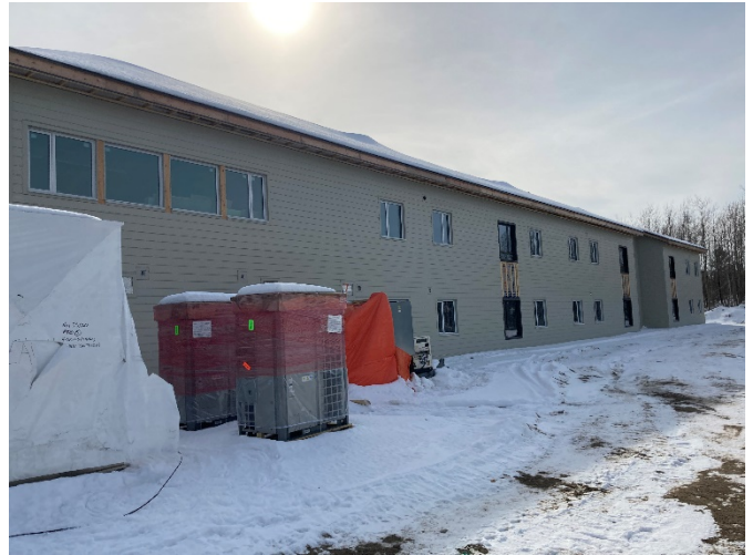
Fiber Cement Siding Install – North West
