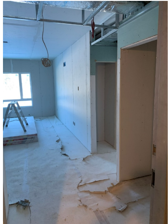
Gypsum Board/Ceiling Framing – LVL 1 East Wing
