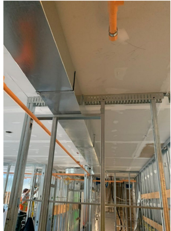
Duct Installation – LVL 1 West Wing
