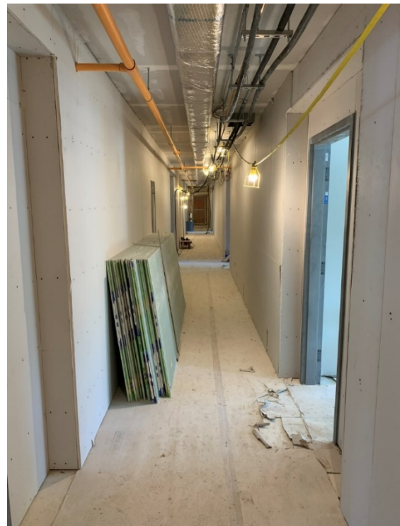
Hallway Progress – LVL 2
