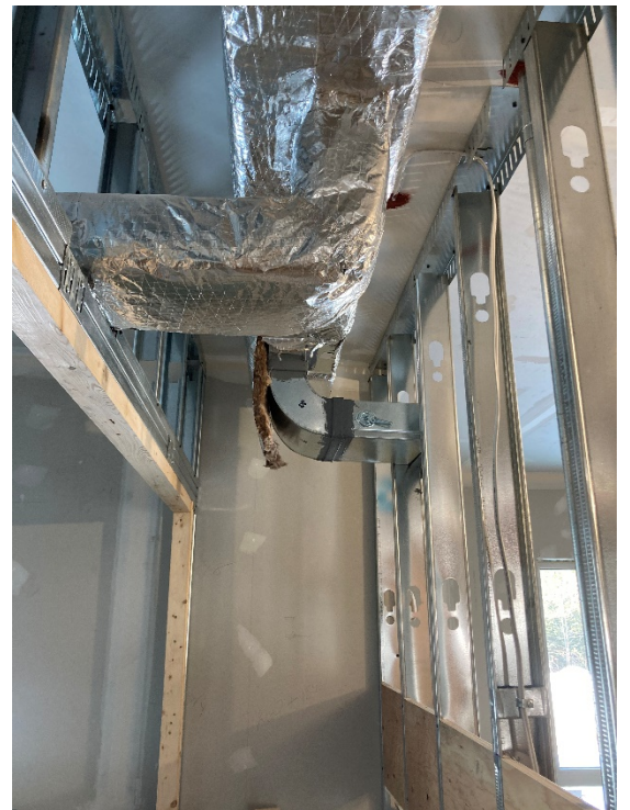
HVAC Installation – LVL 1
