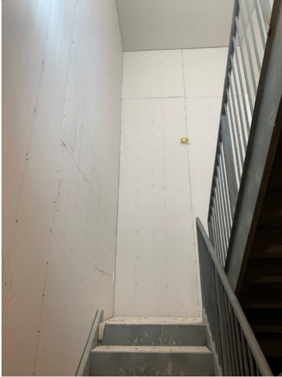
Gypsum Board – Stair # 3
