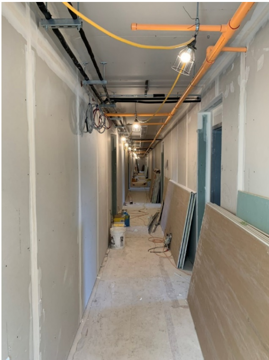
Hallway Progress – LVL 2
