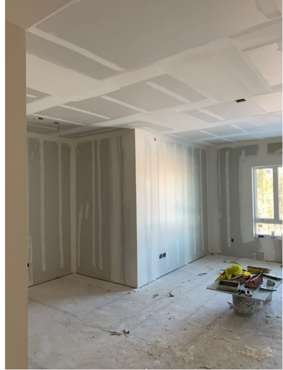
Taping Progress – LVL 2 East Wing
