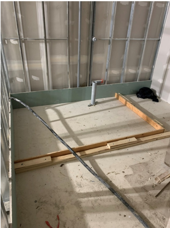
Laundry Room Housekeeping Pad Formwork
