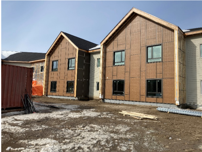
EZ Trim Install – South
