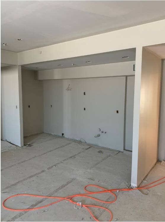
Prime/Paint Progress – LVL 2
