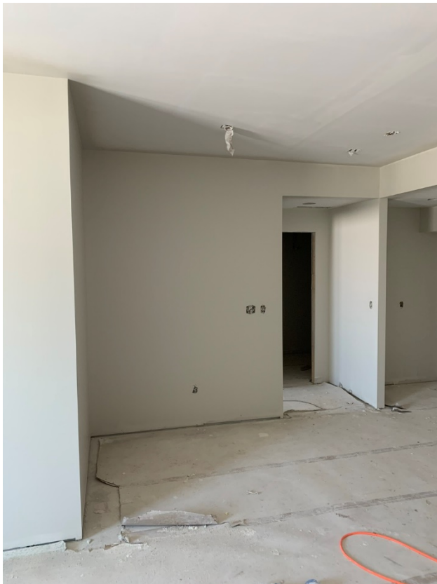
Prime/Paint Progress – LVL 2
