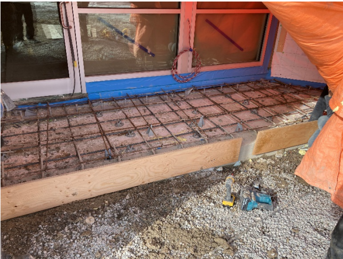
Front Entrance Rebar Install
