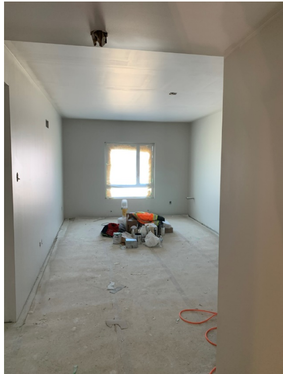
Prime/Paint Progress – LVL 2
