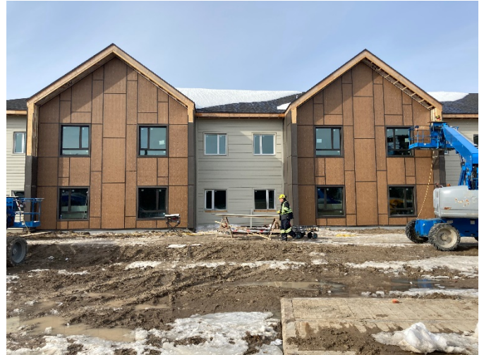
EZ Trim Install – South
