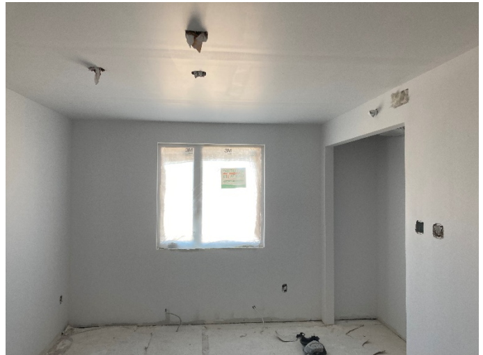
Prime/Paint Progress – LVL 2
