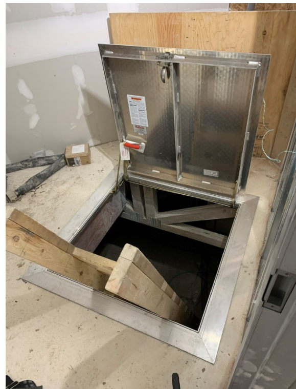
Crawlspace Access Hatch Installed
