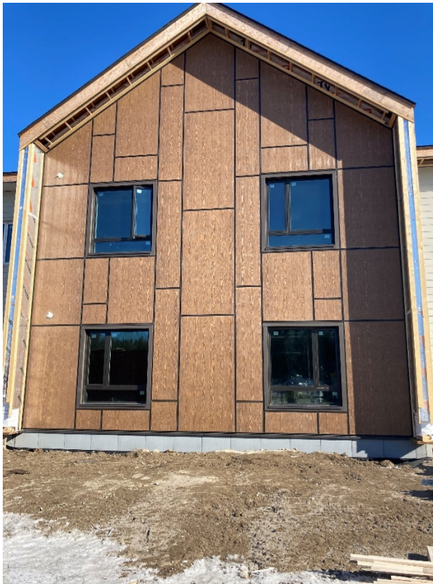
EZ Trim Install – South
