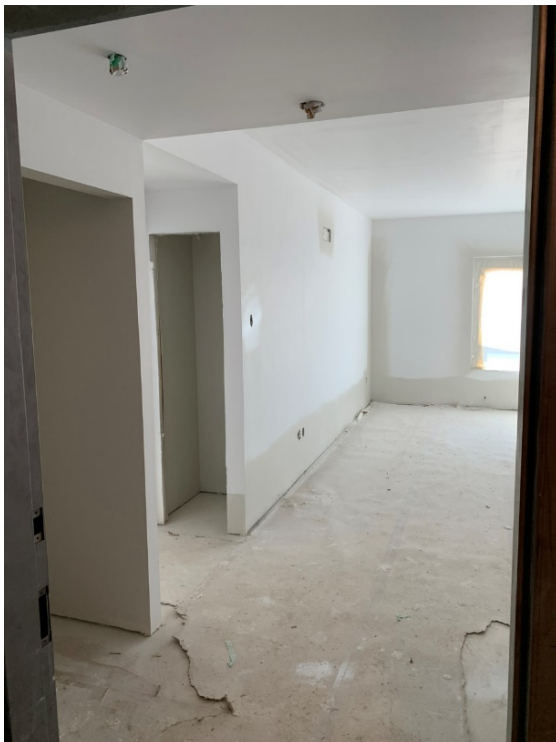
Prime/Paint Progress – LVL 2
