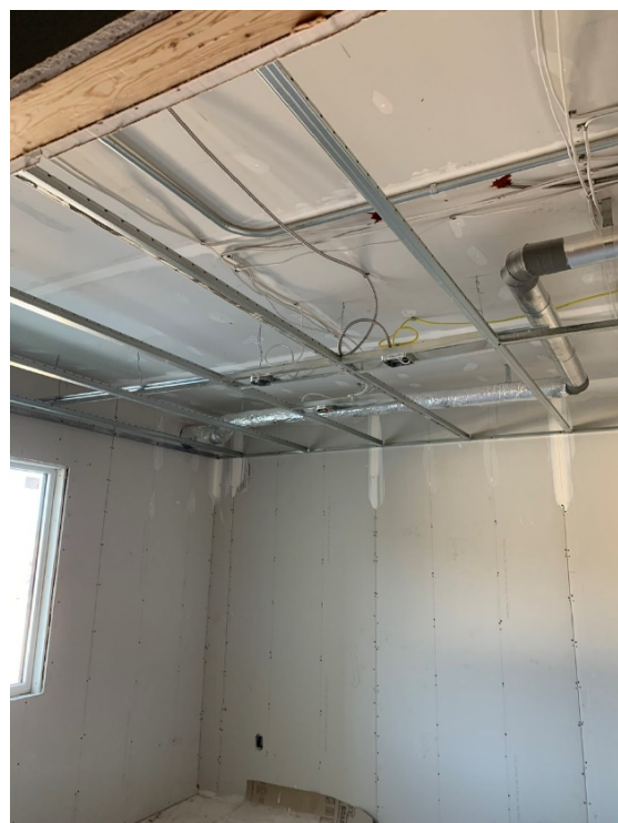
Suspended Ceiling Framing – LVL 1
