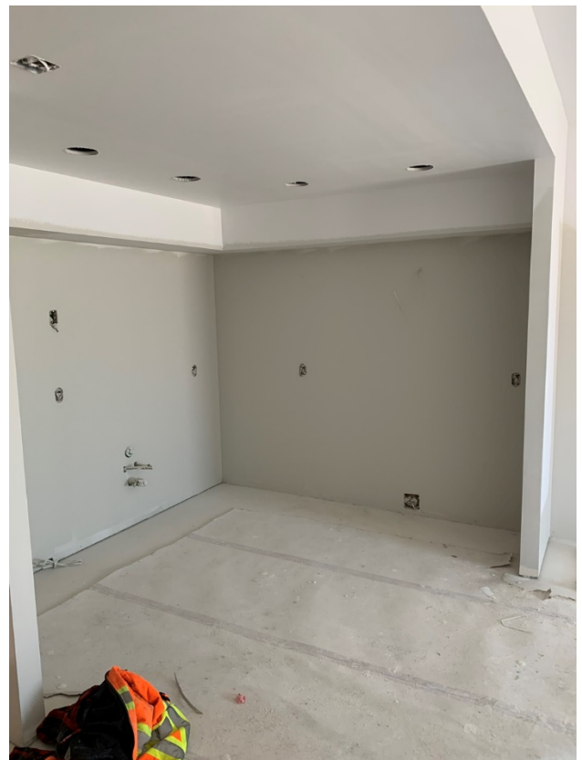
Prime/Paint Progress – LVL 2
