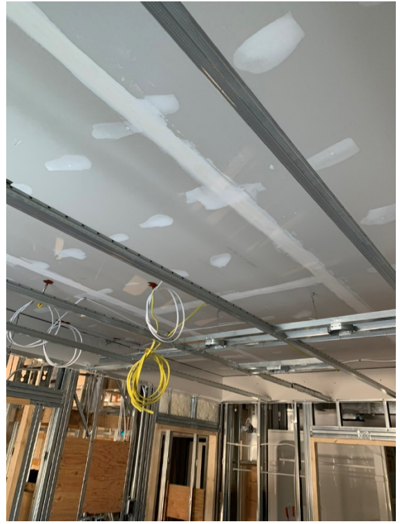
Suspended Ceiling Framing – LVL 1
