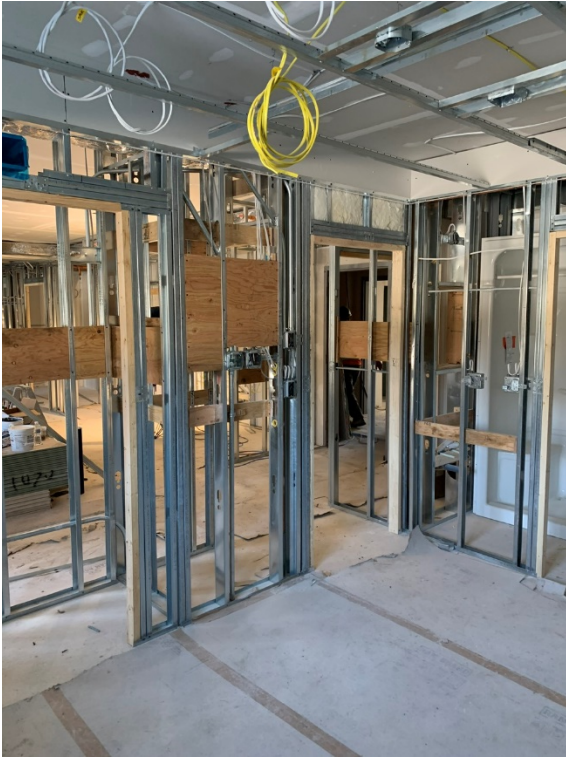
Suspended Ceiling Framing – LVL 1
