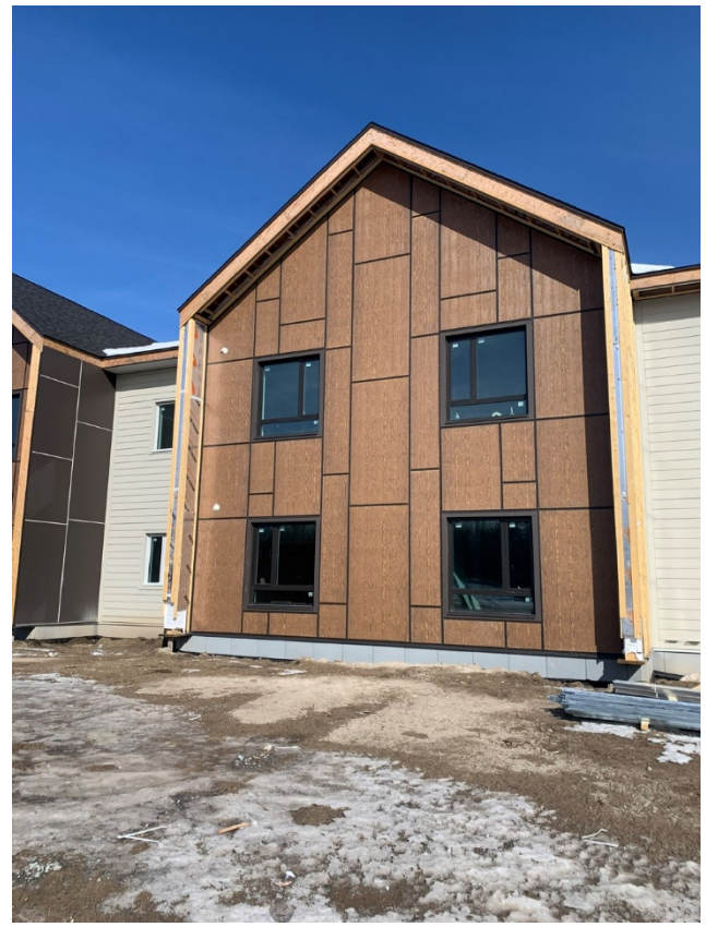
EZ Trim Install – South
