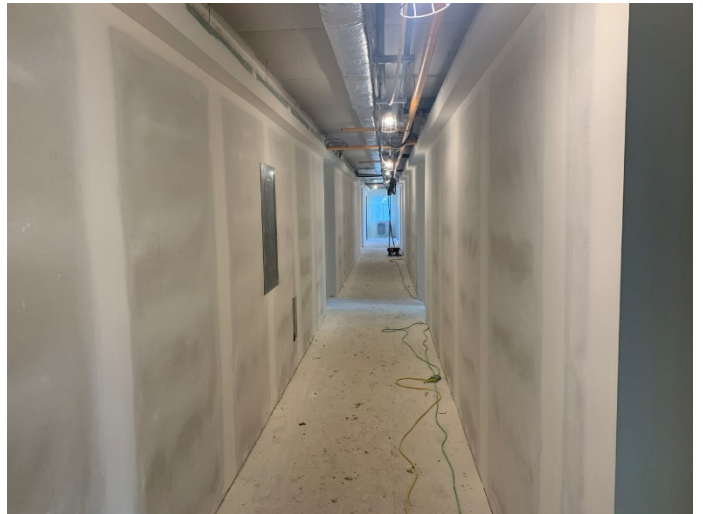
LVL 2 Corridor Progress
