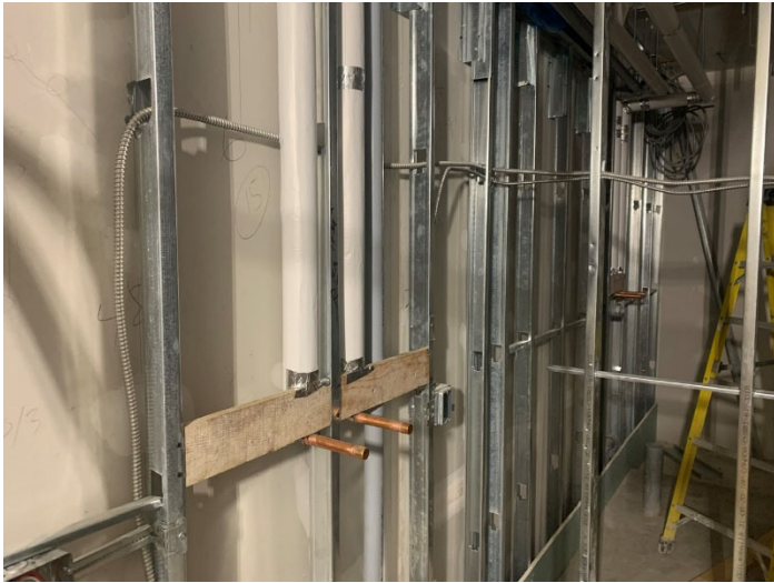
LVL 1 Laundry Domestic Water Rough In
