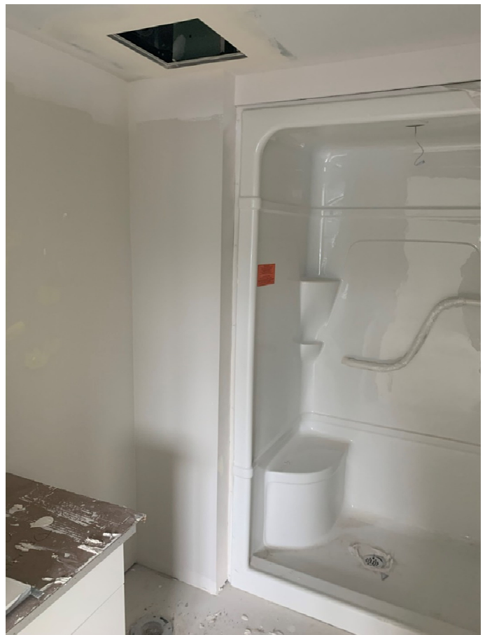
LVL 2 Access Hatch Install Progress
