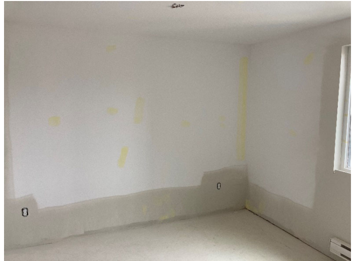
LVL 2 Touch-Up Progress
