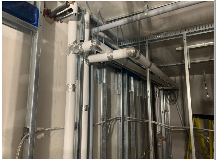
LVL 1 Laundry Domestic Water Rough In
