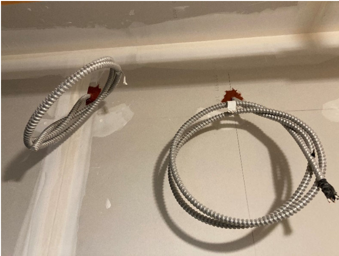
LVL 2 Corridor Electrical Firestopping
