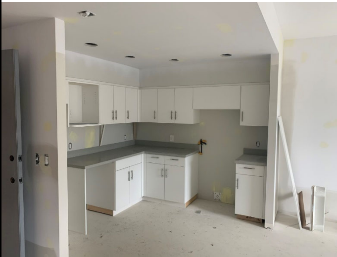
LVL 2 1 BR Millwork Install Progress
