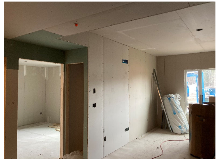
LVL 1 Wall/Ceiling Board Progress
