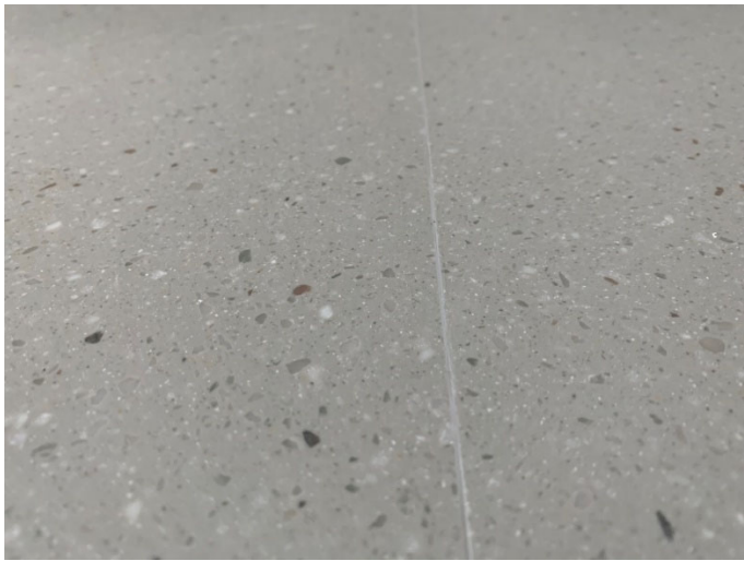
LVL 2 Countertop Seam
