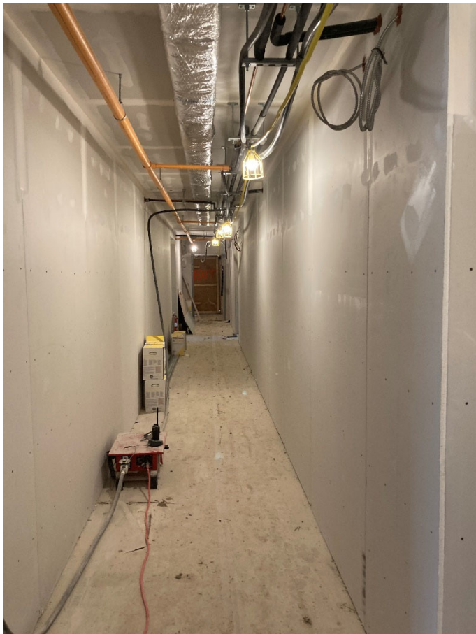
LVL 1 Corridor Progress
