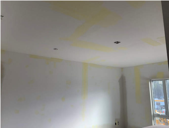
LVL 2 Touch-Up Progress
