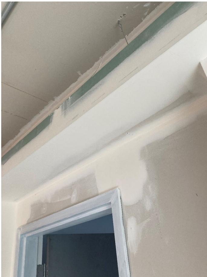
LVL 1 Corridor Bulkhead Progress
