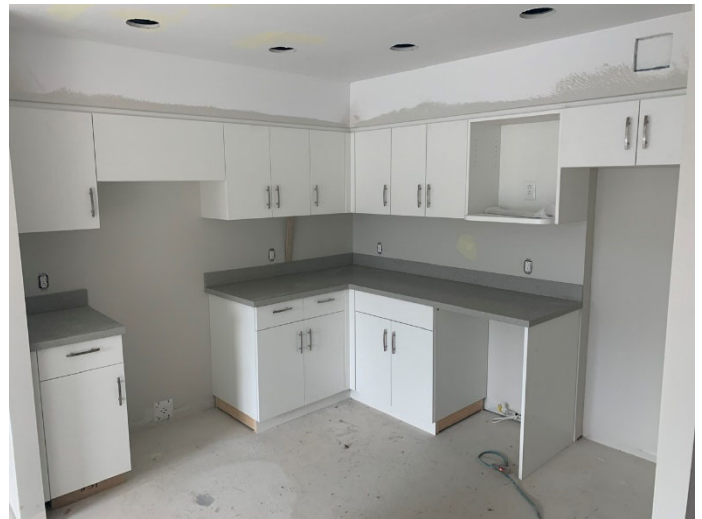
LVL 2 2 BR Millwork Install Progress
