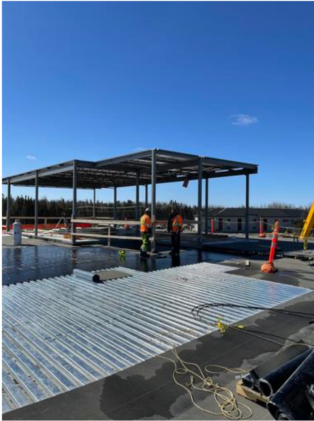
B1- Installing vapor barrier over primed deck
