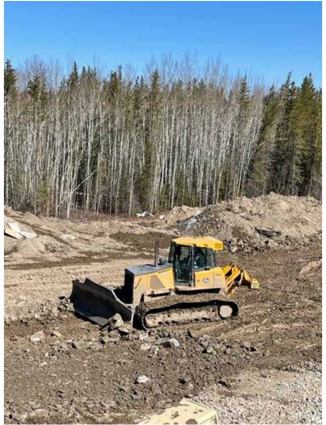
Dozer placing material for temporary access
