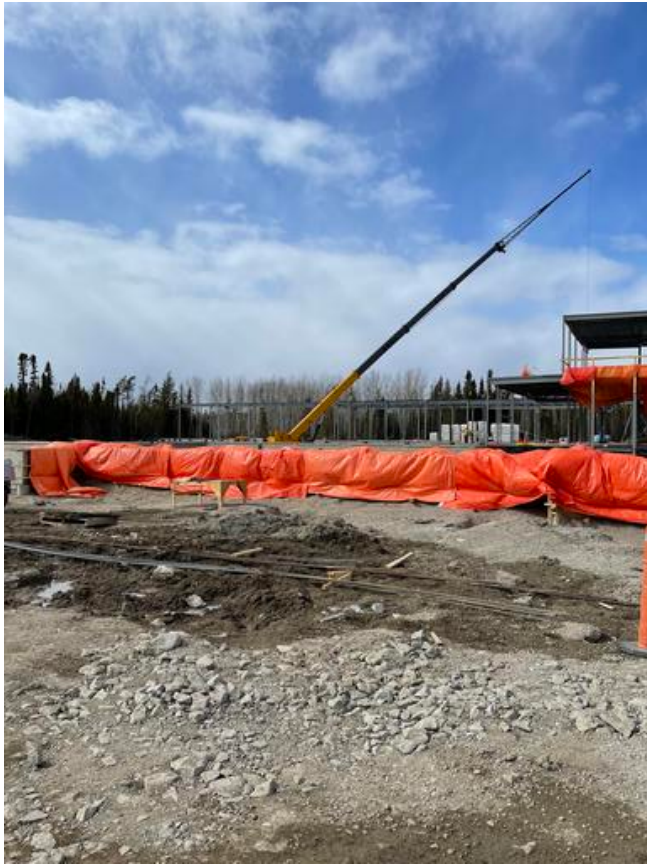
C1- Placing tarps over grade beam
