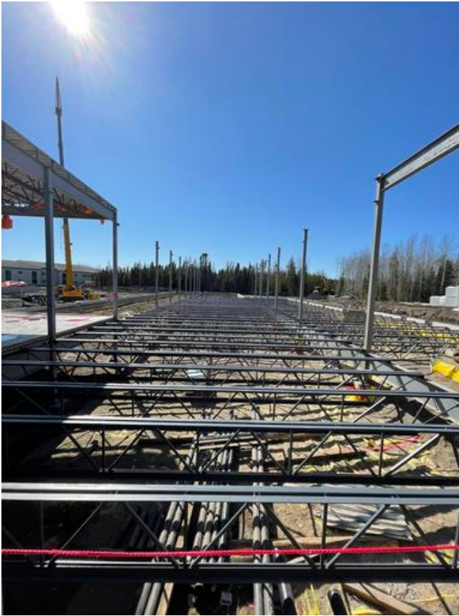
B2- Erection of floor structure
