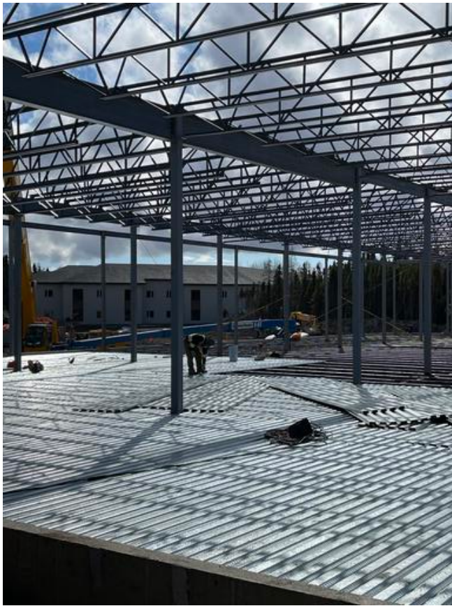
B2- Installing Q-Deck Arshdeep Grewal Apr 25, 2021 1:52 PM
