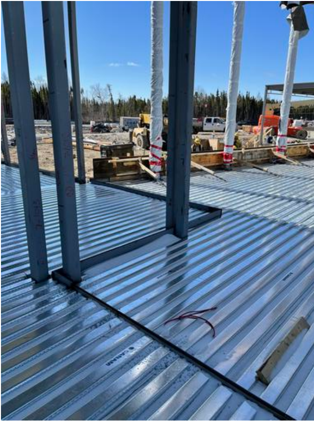
A3- Installed expansion joint Arshdeep Grewal Apr 24, 2021 8:52 AM
