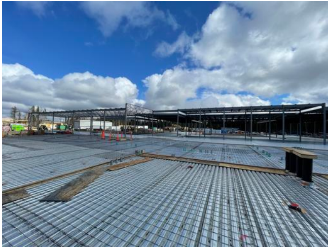
A1-Wire mesh over Q-Deck
