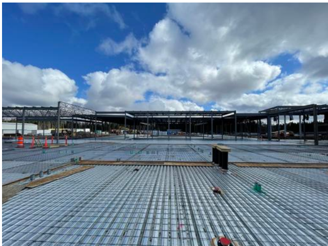
A1-Wire mesh over Q-Deck Arshdeep Grewal Apr 25, 2021 1:52 PM
