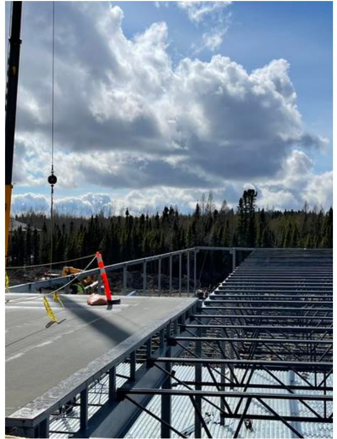
B2- Erection of roof structure Arshdeep Grewal Apr 25, 2021 1:52 PM
