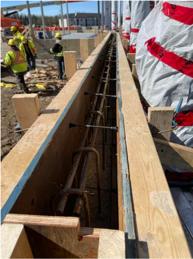
A3- Rebar close up for curtain wall Arshdeep Grewal Apr 24, 2021 8:52 AM
