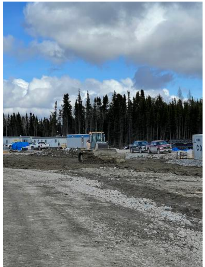
Dozer placing material for laydown areas
