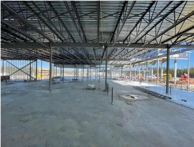
B1-1 - Concrete slab-on-deck
