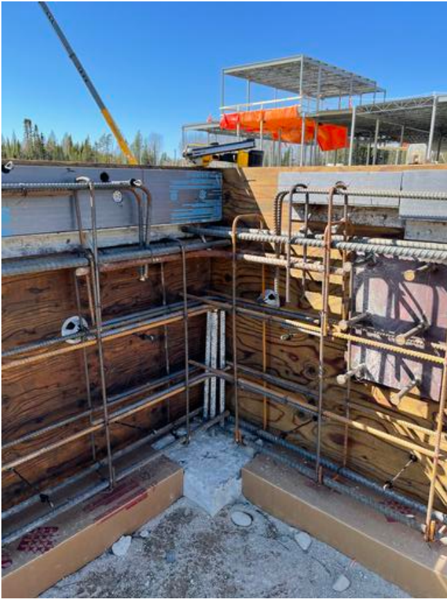
C1- Grade beam rebar closeup Arshdeep Grewal Apr 21, 2021 4:10 PM
