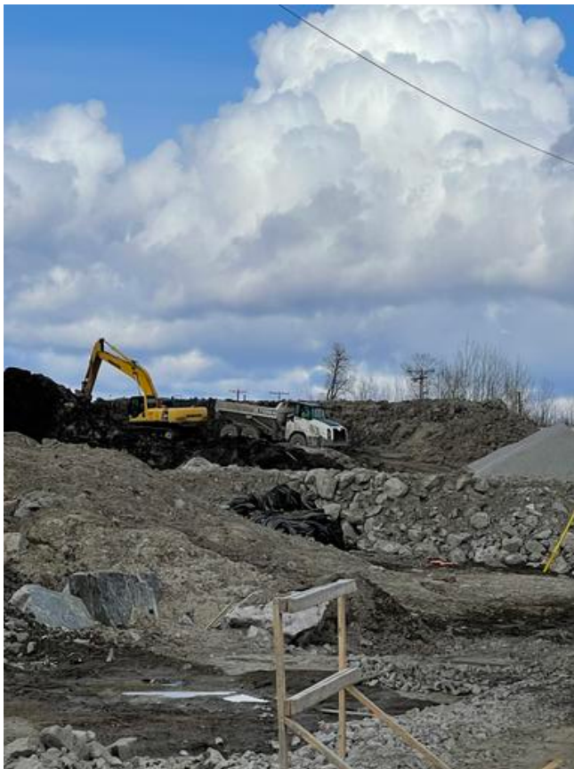
Excavator loading truck with material
