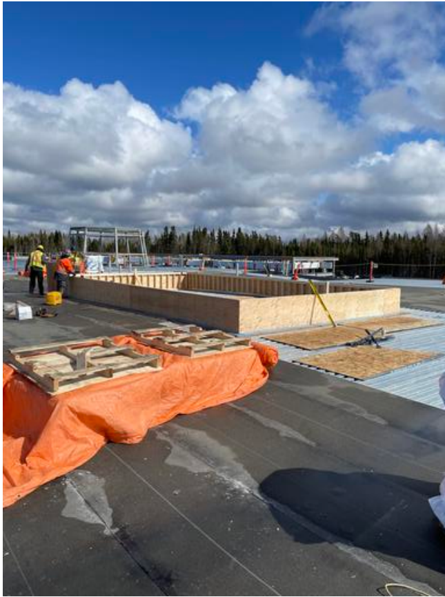
A3- Building roof curbs for RTU Arshdeep Grewal Apr 25, 2021 1:52 PM
