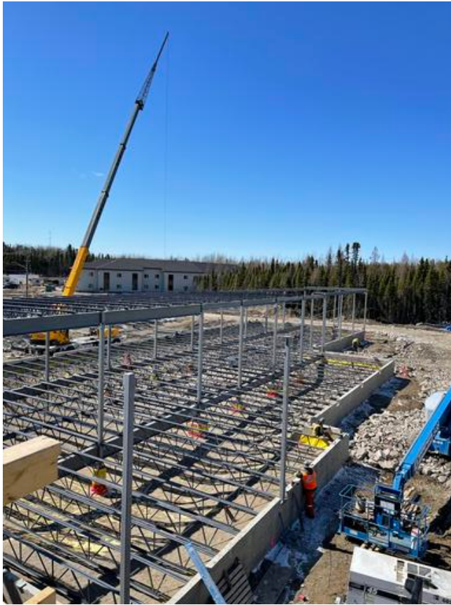
B2- Erection of roof structure Arshdeep Grewal Apr 24, 2021 8:52 AM
