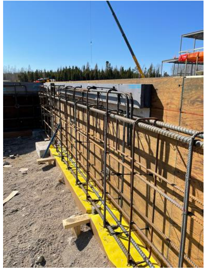
C1- Grade beam rebar closeup Arshdeep Grewal Apr 21, 2021 4:09 PM
