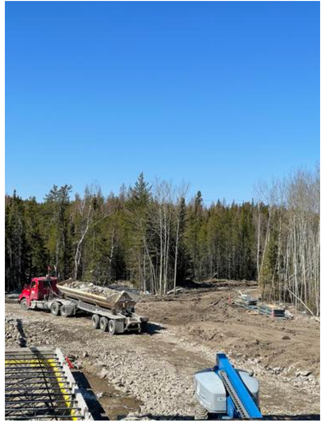
Truck hauling rock for building access to site Arshdeep Grewal Apr 24, 2021 8:52 AM
