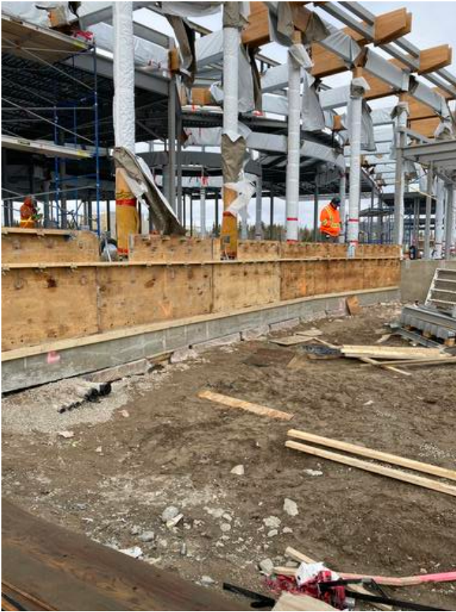
A3- Installing formwork for curtain wall
