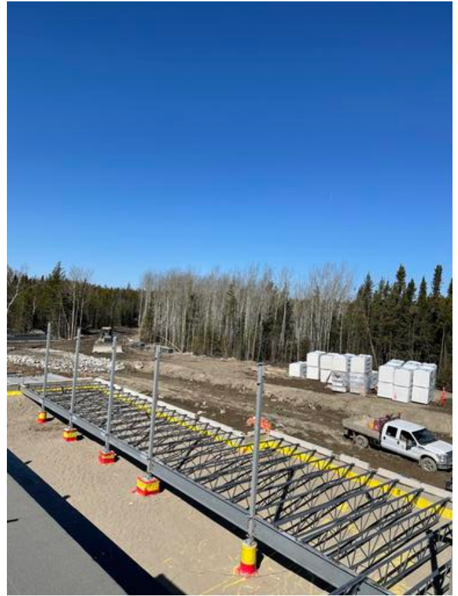
B2- Erection of floor structure Arshdeep Grewal Apr 21, 2021 4:52 PM
