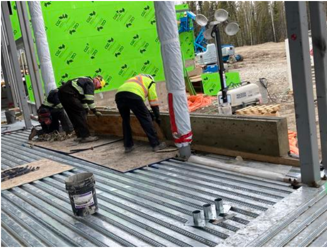
Removing form work from curbs A3
