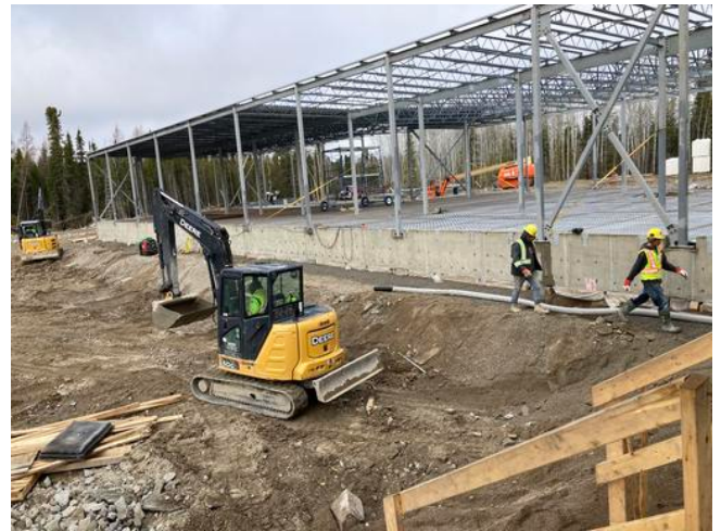
Installing weeping tile along GB (B2)
