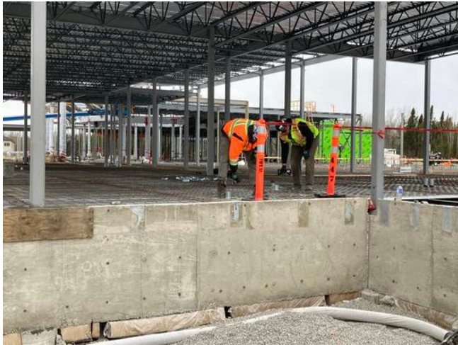
Drilling holes in deck A2 for installing hangers
