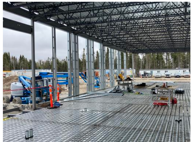
Steel stud framing along GL 16e (A2)
