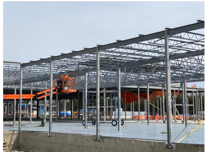
Straightening and torquing B2 roof level
