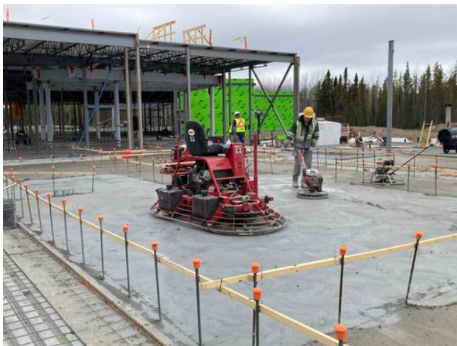
Working on finishing of concrete (A1-1)
