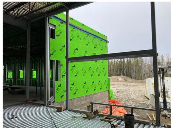
Exterior sheathing B1 along GL 4W
