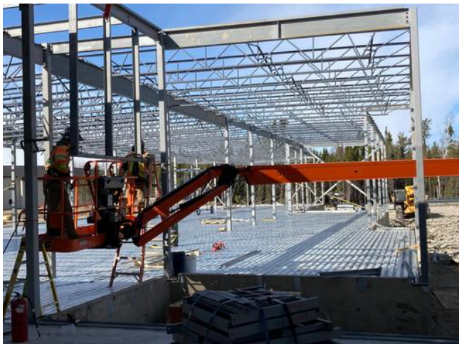
Working on C-channels in B2 Anmol Kang Apr 29, 2021 7:47 AM
