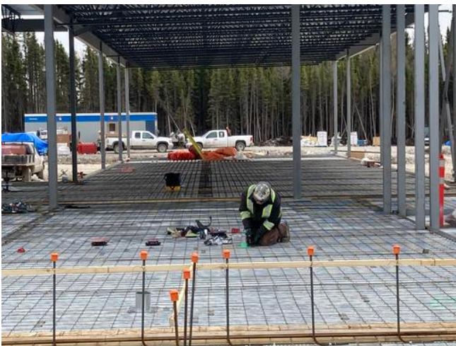
Installing sleeves in A2
