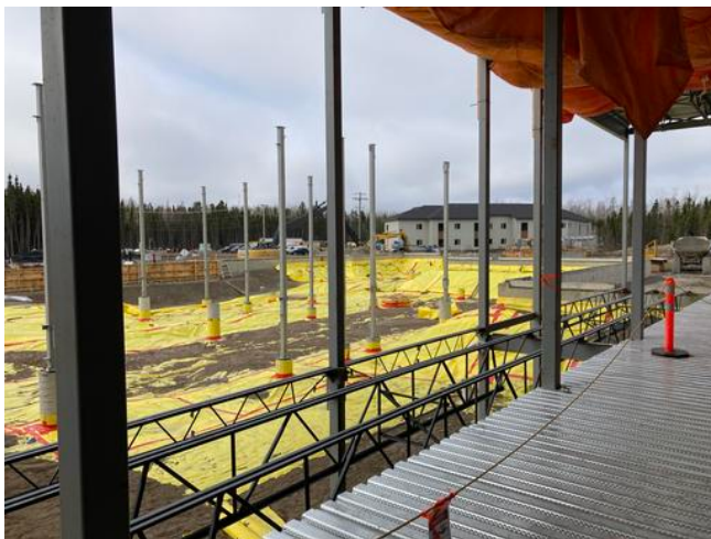
Poly in C1, C2 and steel columns in C1
