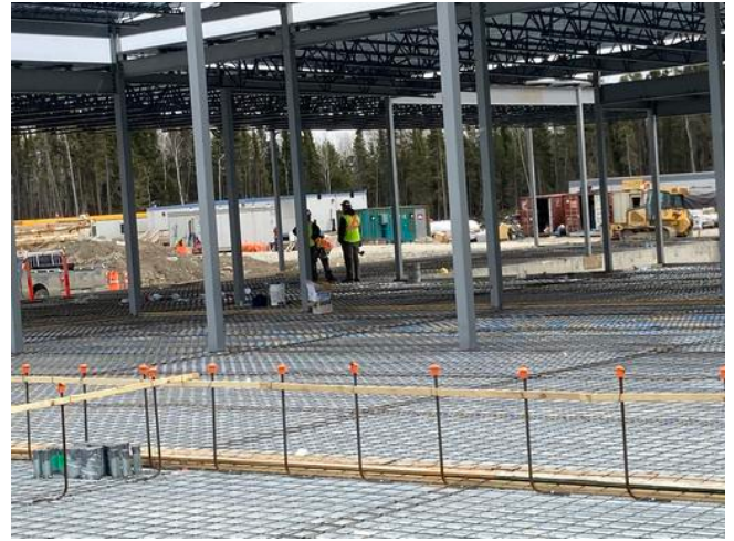
Mesh over deck in A2
