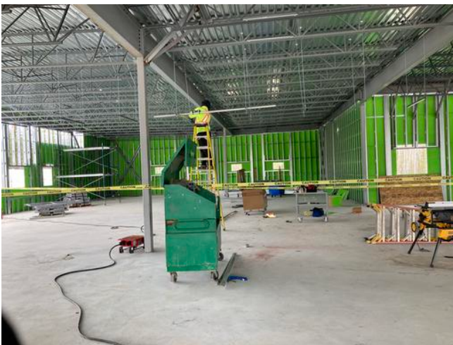
Working on hangers B1 roof level
