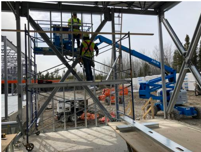
Stud framing along GL 15W
