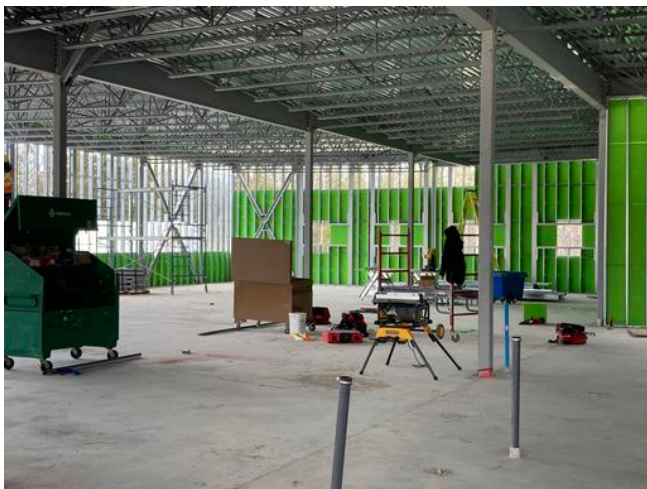
B1 exterior sheathing work in progress
