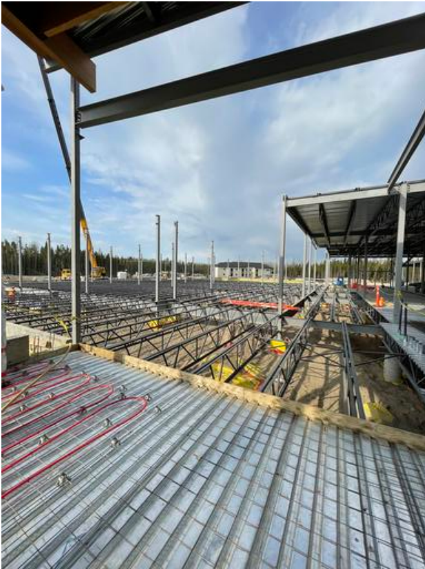
C1- Erection of floor structure Arshdeep Grewal May 14, 2021 7:52 AM
