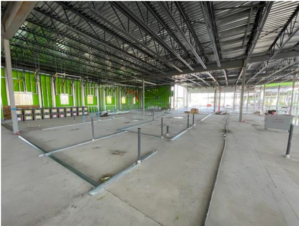
B1- Installing track for interior walls
