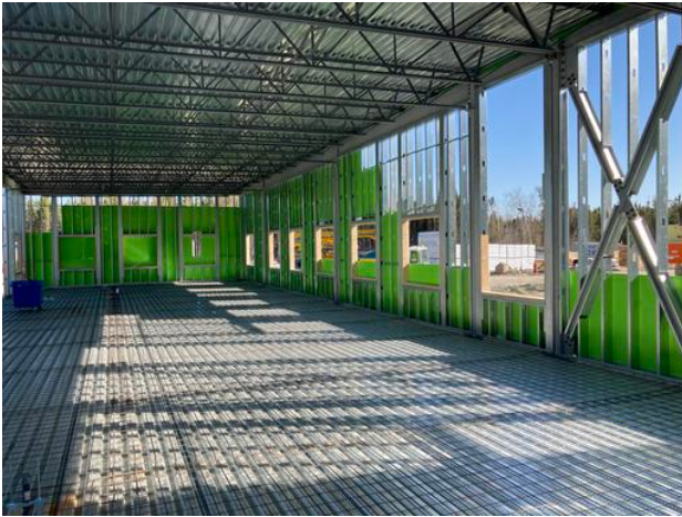
Exterior sheathing work in progress A2
