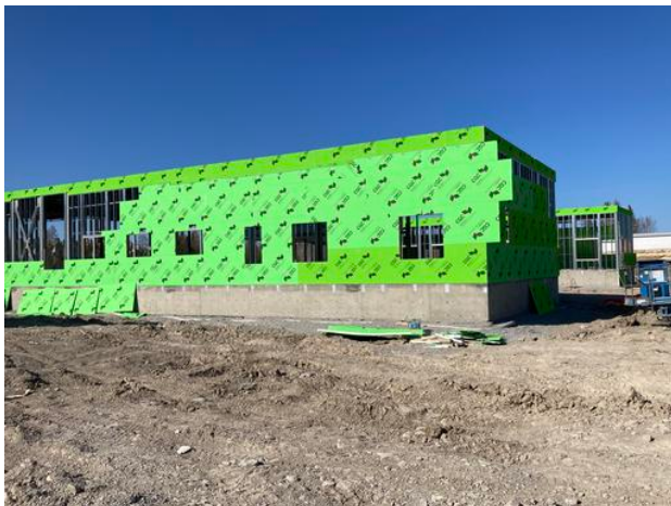
Exterior sheathing A2 along GL 6e
