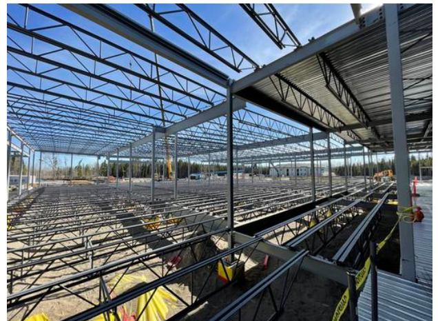
C1- Erection of roof structure
