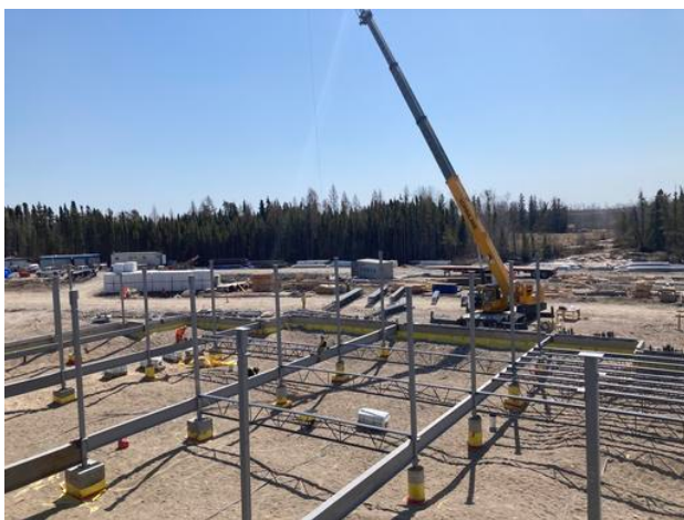
C1- Erection of main floor structure
