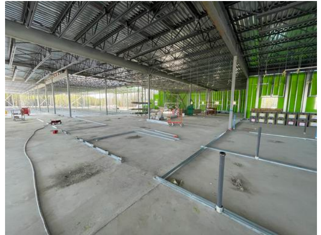
B1- Installing track for interior walls
