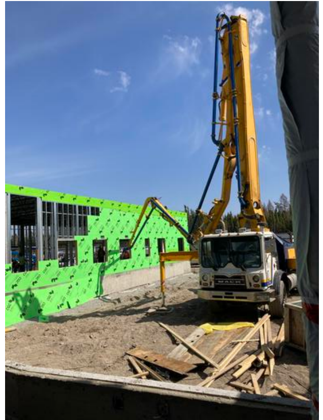
Pouring concrete with Concrete Pump Truck Anmol Kang May 13, 2021 5:41 PM
