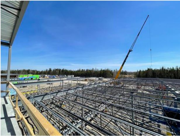
C1- Erection of roof structure
