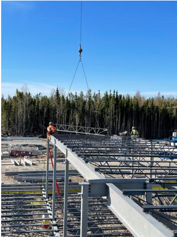
C1- Erection of roof structure
