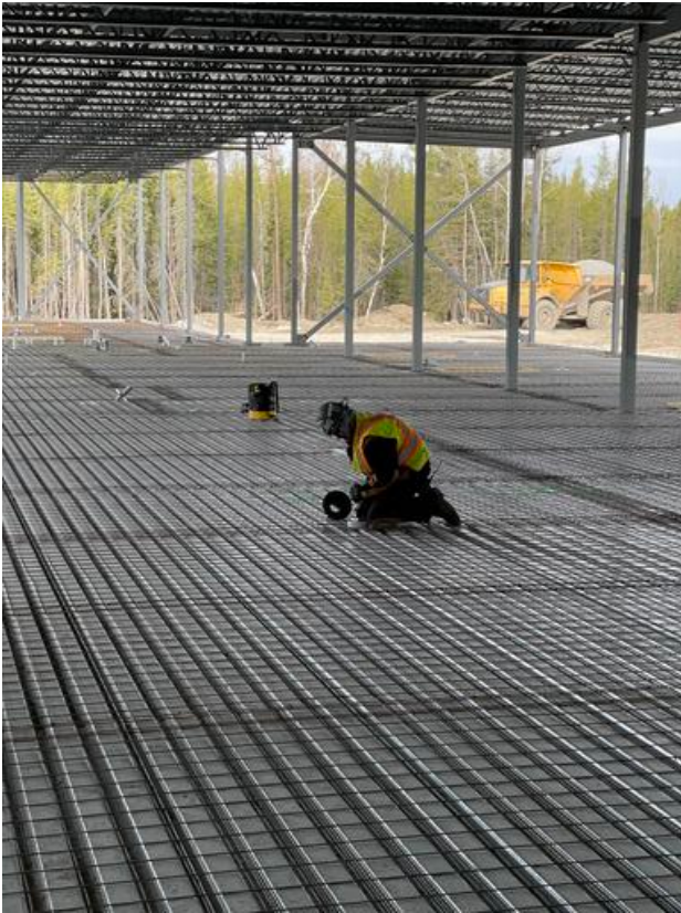
B2- Installing floor drains Arshdeep Grewal May 14, 2021 7:52 AM
