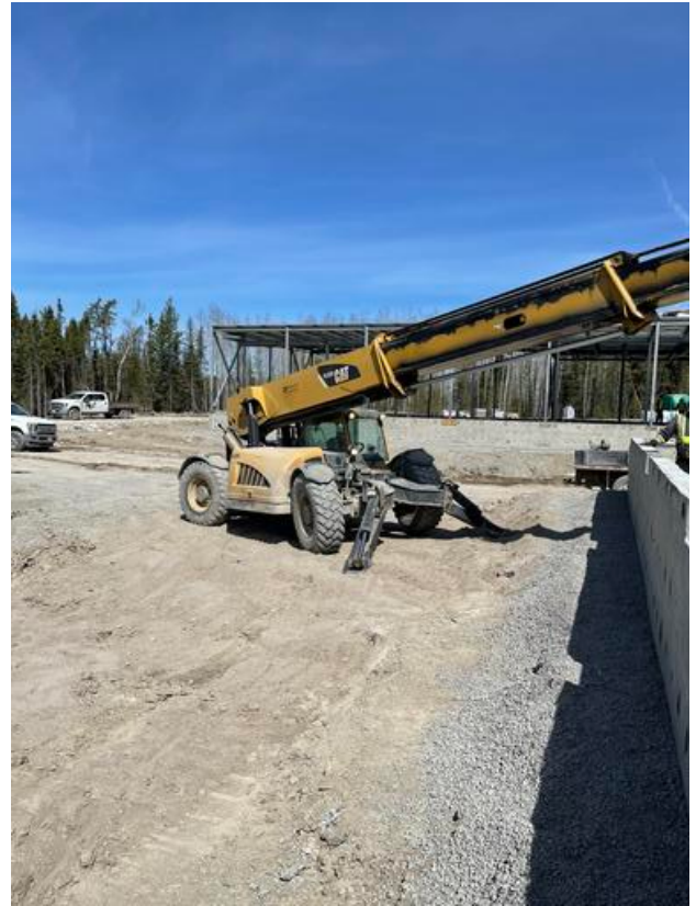
Telehandler being used for bucket pour
