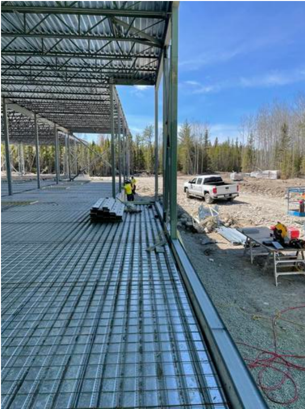
B2- Installing tracks along grade beam for framing
