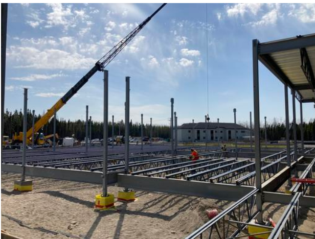
C1- Erection of floor structure Anmol Kang May 13, 2021 5:41 PM
