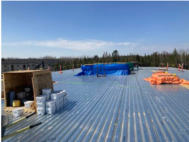
B2- Material covered and stored over dunnage
