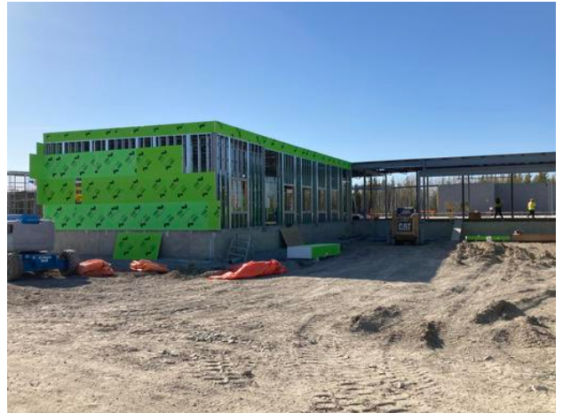
Exterior sheathing work in progress A2
