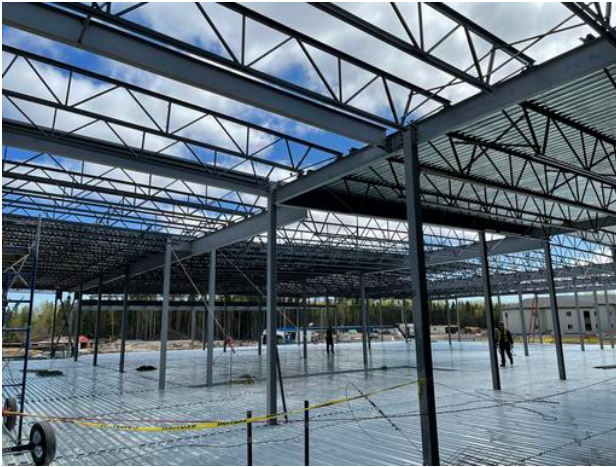
C1- Straightening structural steel
