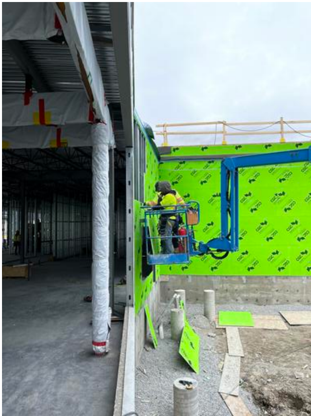
A3- Sheathing exterior north side Arshdeep Grewal May 21, 2021 7:59 AM
