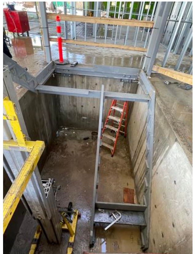
B1- Installing stairs
