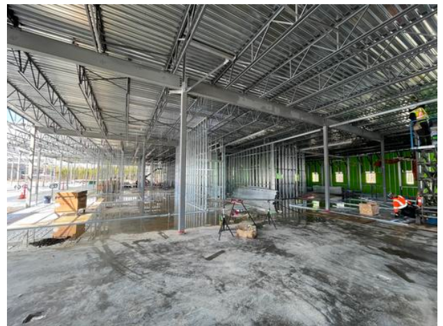
B1- Framing interior walls
