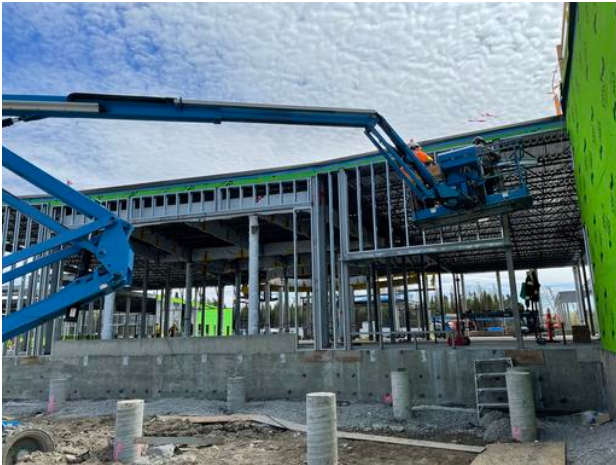
A3- Framing exterior wall
