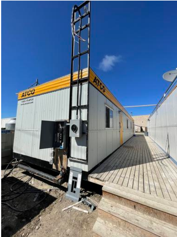
Electrical panel installed for upper office
