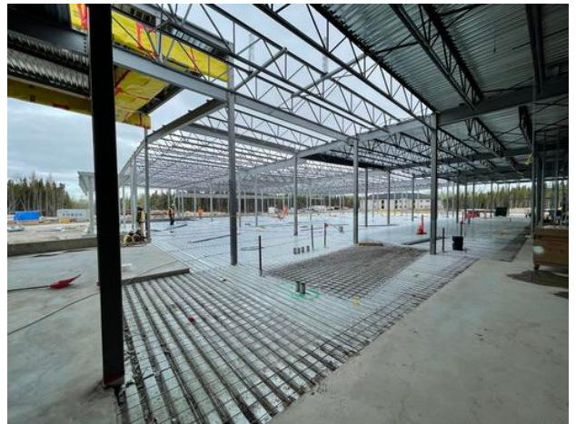
C1- Installing Q-Deck Arshdeep Grewal May 21, 2021 7:59 AM
