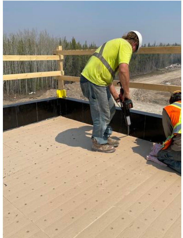
B1- Sealing insulation around ends
