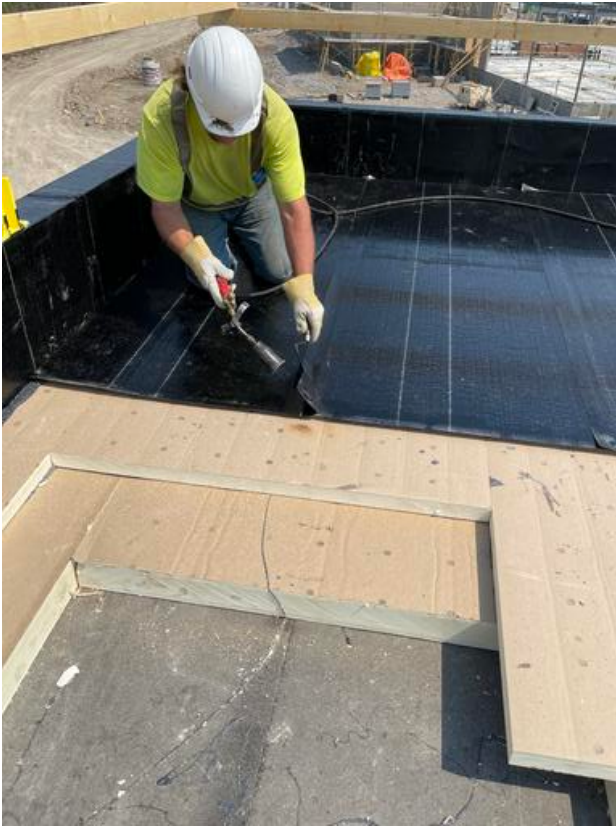
B1- Torching base sheet over insulation Arshdeep Grewal May 19, 2021 5:12 PM
