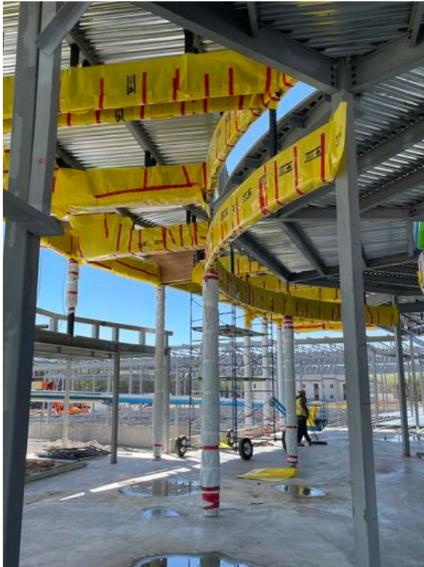
A3- Wrapping glulam Arshdeep Grewal May 20, 2021 9:02 AM
