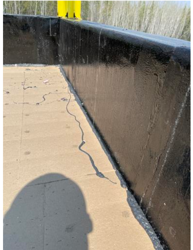
B1- Insulation sealed around ends Arshdeep Grewal May 19, 2021 5:12 PM
