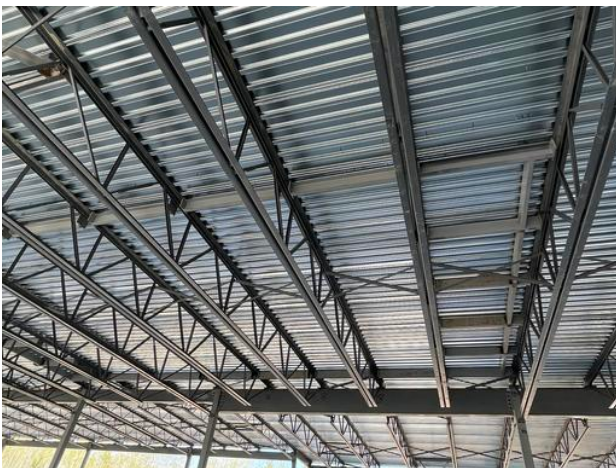
B2- Structural support underneath RTU
