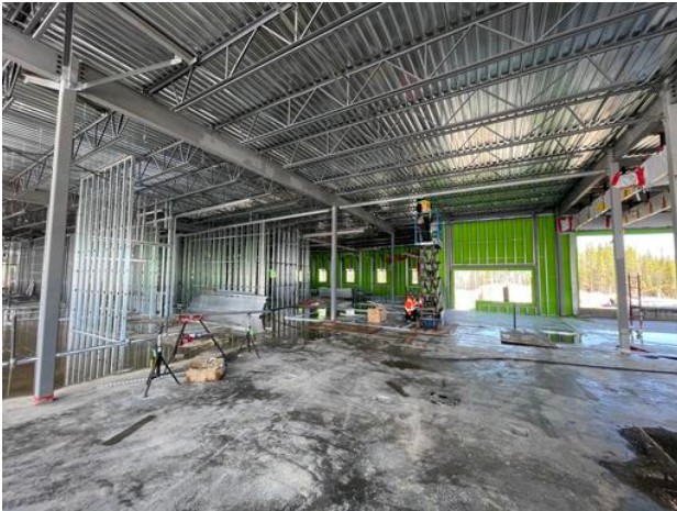
B1- Installing tracks for interior walls
