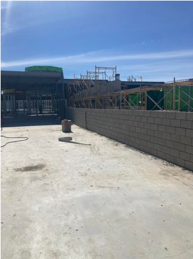
Masonry wall work in progress
