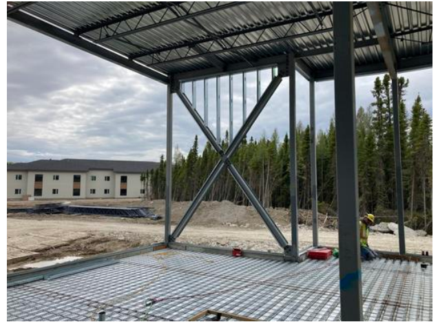
Installing exterior studs in B2
