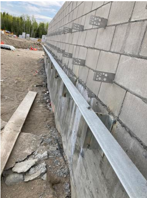
Installing exterior angle
