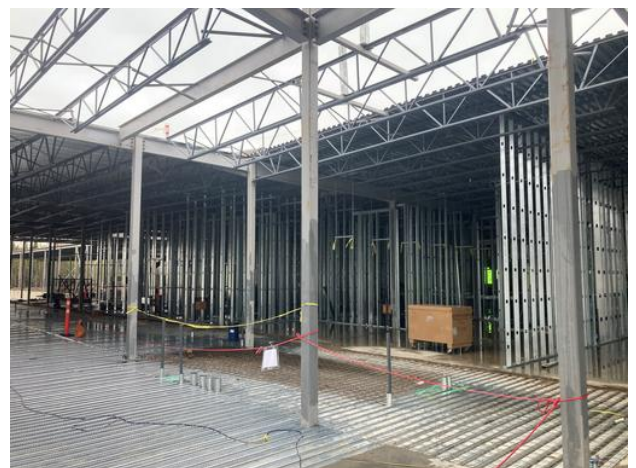
B1- Interior stud framing Arshdeep Grewal May 26, 2021 10:16 AM
