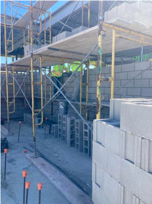
Laying masonry blocks in A1 along GL Ge
