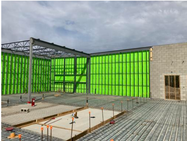
Exterior sheathing in A1
