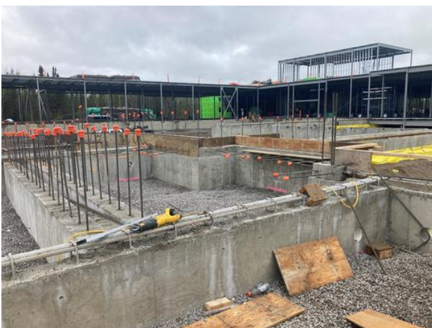
C2- Building formwork for curbs Arshdeep Grewal May 26, 2021 10:16 AM
