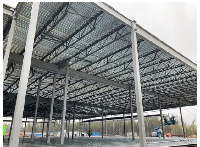
C1- Installing Q-Deck at roof level
