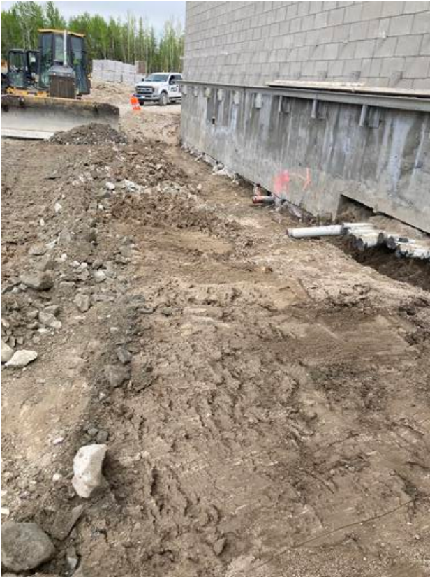
Clearing area for weeping tile and priming GB
