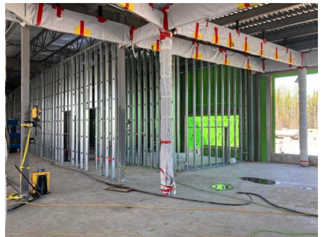
Stud framing in west figure A1 Anmol Kang Jun 3, 2021 4:59 PM
