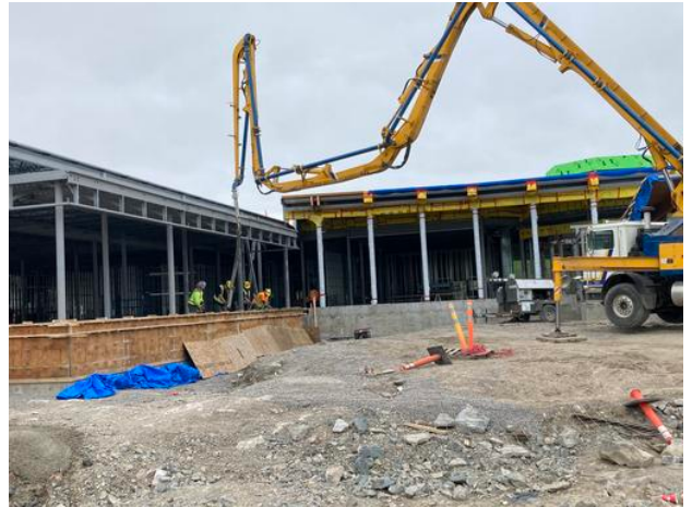
Pouring concrete in C1 curb
