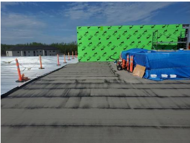
Vapour barrier installed
