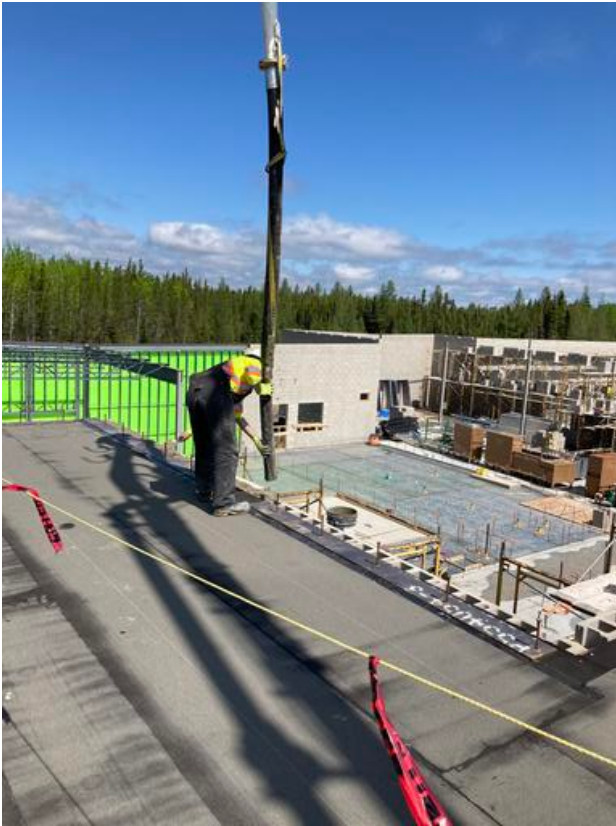
Pouring concrete into masonry wall
