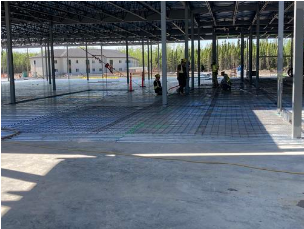
Laying mesh in C1
