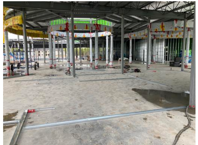
A3 bottom tracks installed
