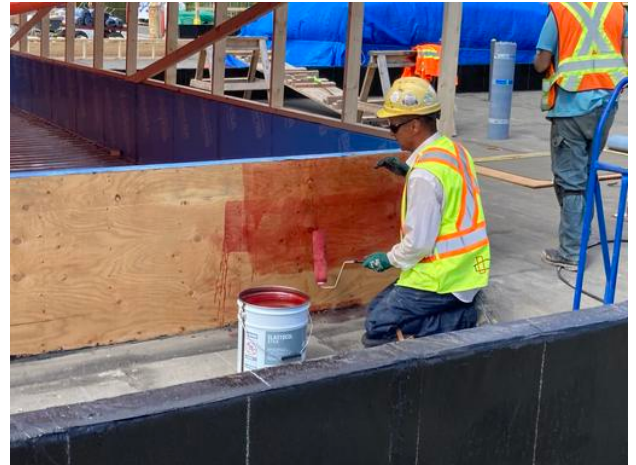
Priming roof curb B1
