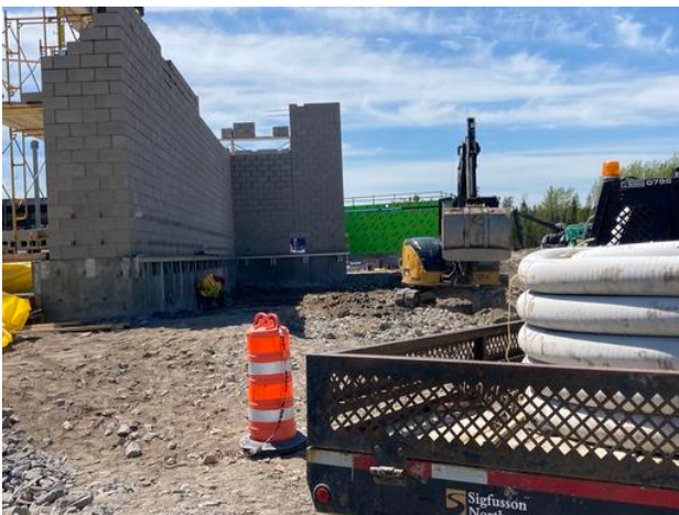
Clearing area for weeping tile A1 Anmol Kang Jun 3, 2021 4:59 PM
