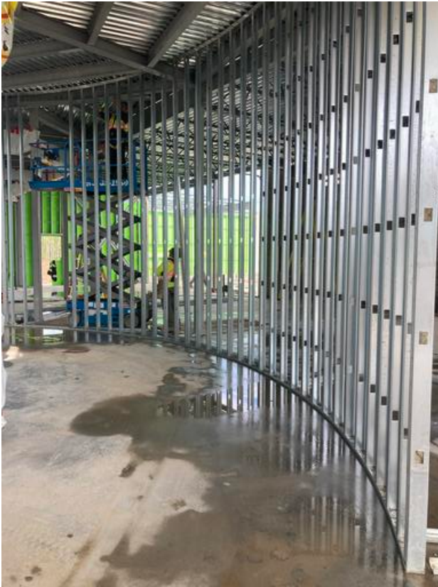
Interior stud framing in A3
