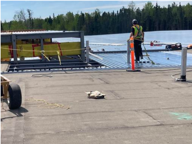
Installing Q deck C1
