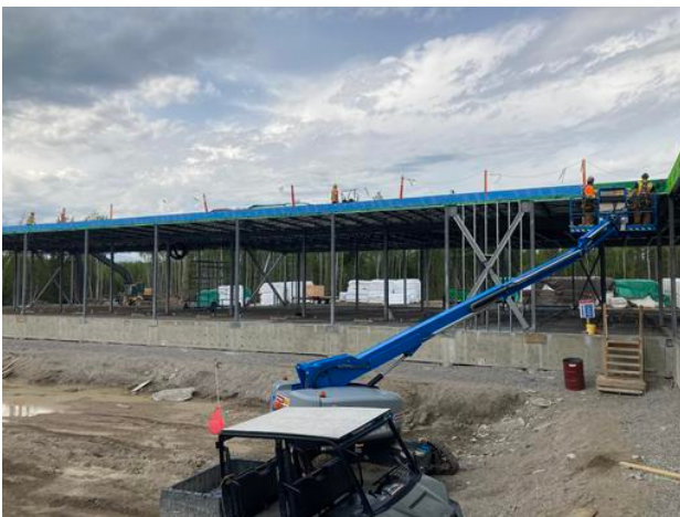
Installing blue skin and flashing around B2
