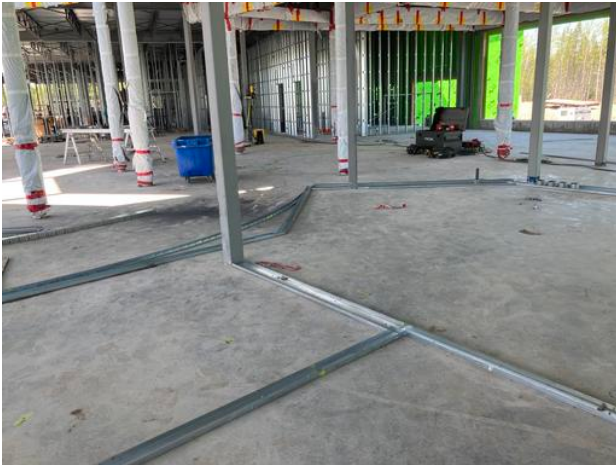
Bottom tracks laid in A3 Anmol Kang Jun 3, 2021 5:04 PM
