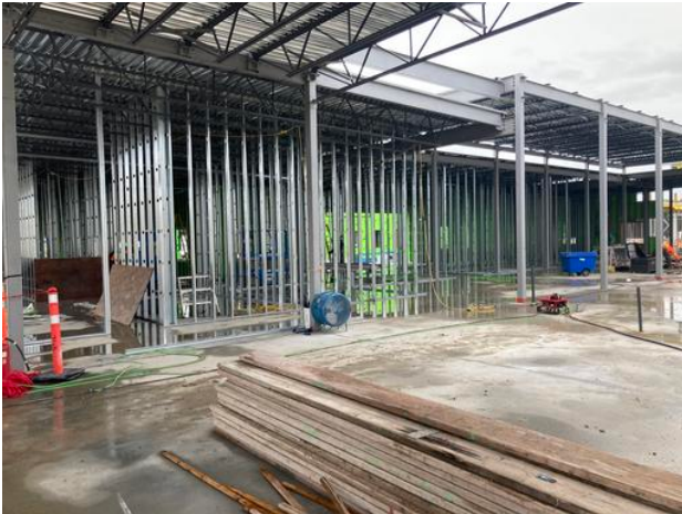
Interior stud framing in A2 Anmol Kang Jun 8, 2021 5:20 PM
