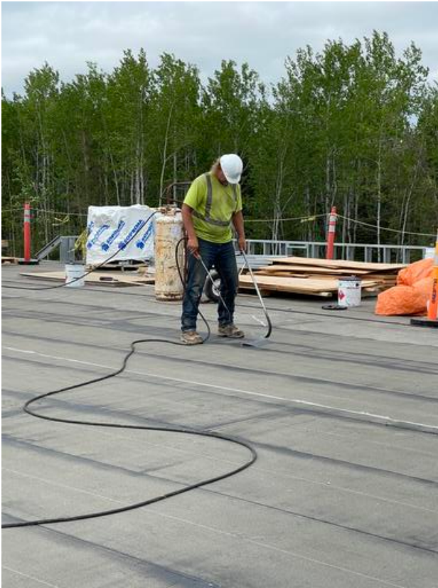
Torching vapor barrier B2 roof Arshdeep Grewal Jun 11, 2021 8:20 AM
