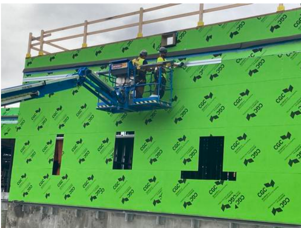
Installing bent flashing Anmol Kang Jun 8, 2021 5:20 PM
