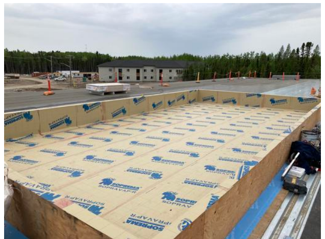
Interior curb B2 roof
