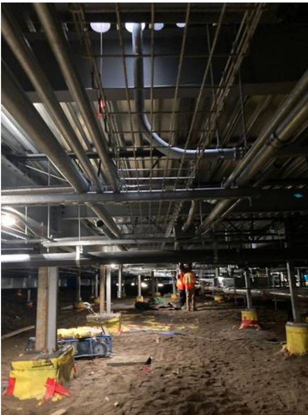
Cable tray installed A1 crawlspace
