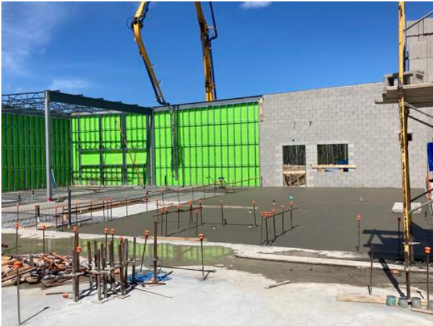
Pouring concrete in A1 kitchen area
