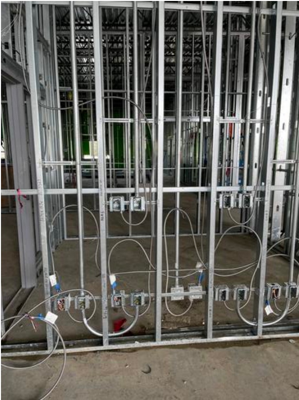
Electrical rough in in stud walls
