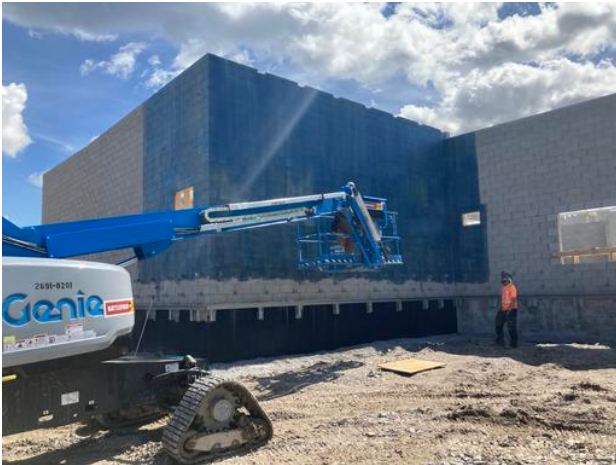
Priming A1 North Wall
