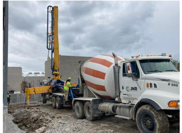
Pumping concrete into masonry walls.
