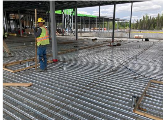
Installing plywood for pour break in B2 Anmol Kang Jun 8, 2021 5:20 PM
