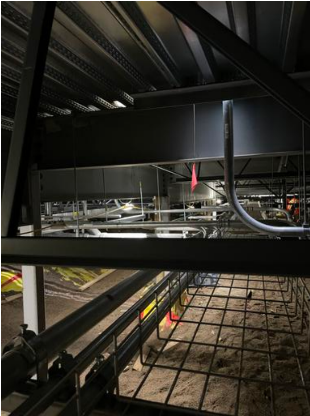
A1- Cable trays installed in crawlspace
