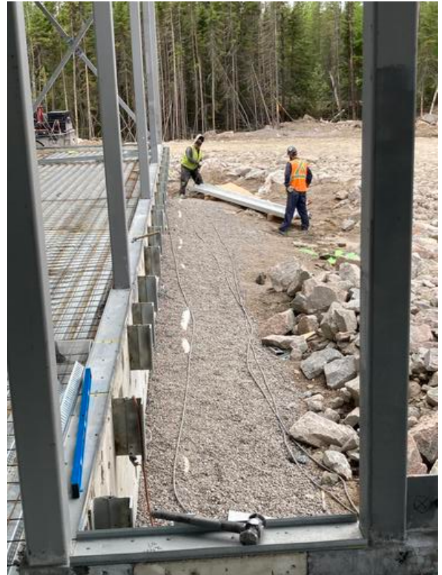
Installing exterior angle
