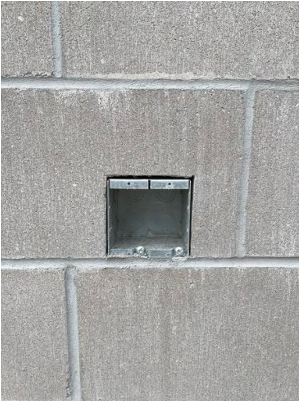
A1- Rough-in (Masonry wall) Arshdeep Grewal Jun 12, 2021 2:02 PM
