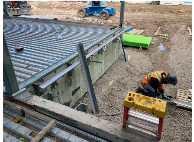
Installing exterior angle Anmol Kang Jun 9, 2021 2:47 PM
