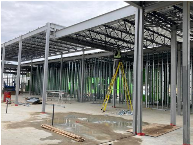
Installing hangers in A2
