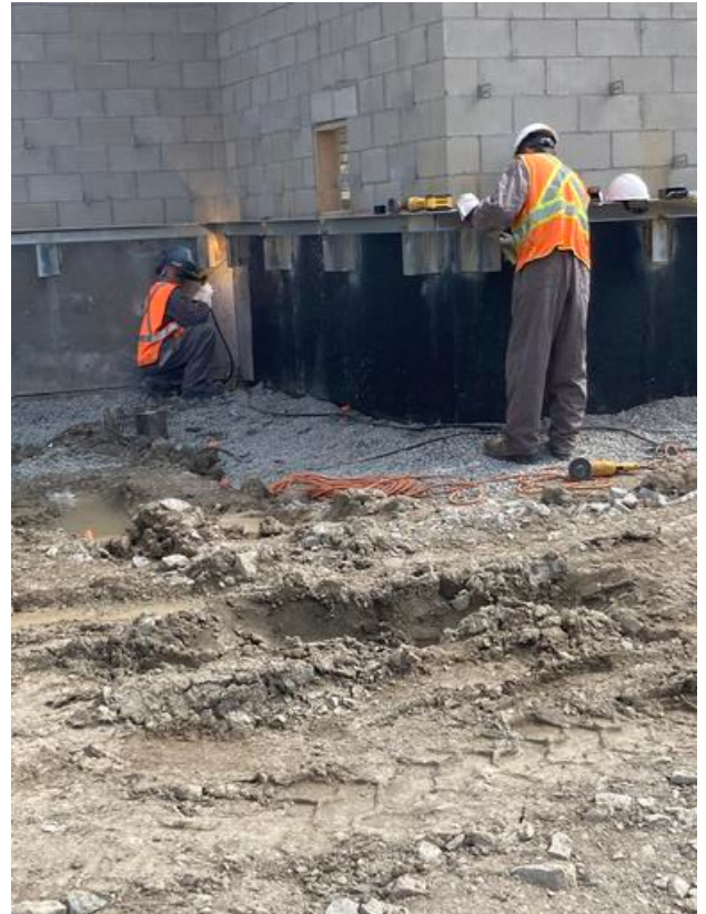
Welding angle on exterior
