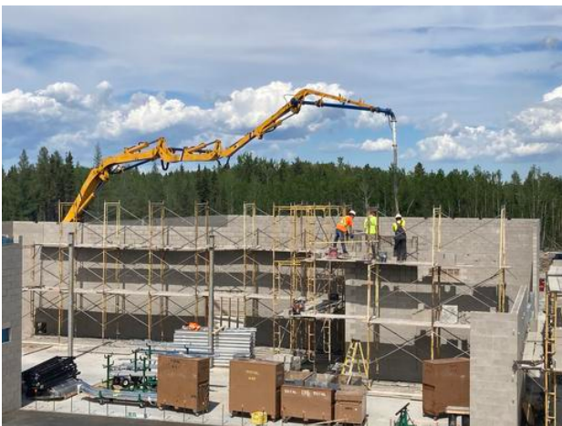
Pouring concrete in masonry wall A1
