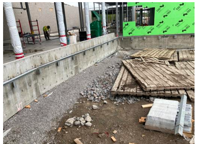
Exterior angle installed in A3 Anmol Kang Jun 8, 2021 5:20 PM
