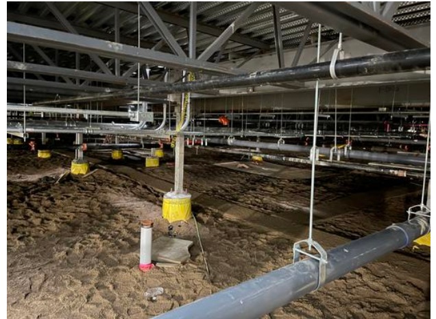
A1- Sanitary, water, sprinkler & conduit lines
