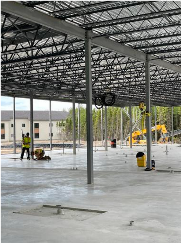
B2- Surveyor laying out M/E rough ins
