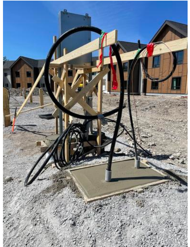
Distribution panel base poured Arshdeep Grewal Jun 23, 2021 8:58 AM
