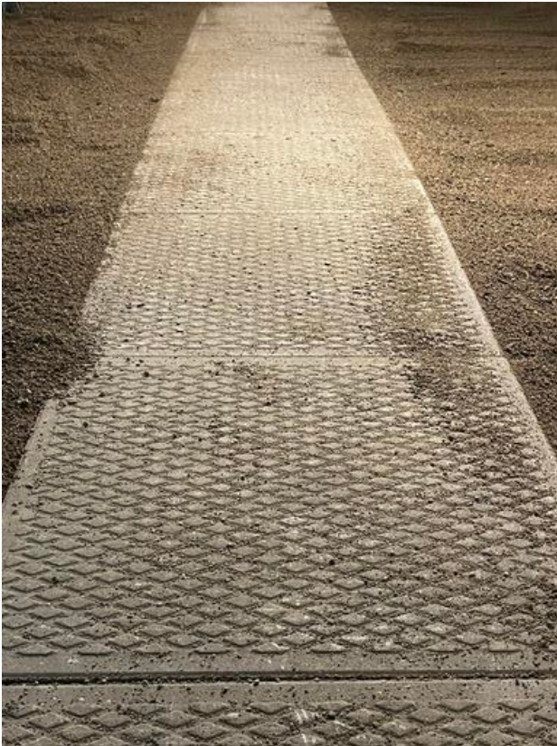
B1- Installing concrete pavers in crawlspace
