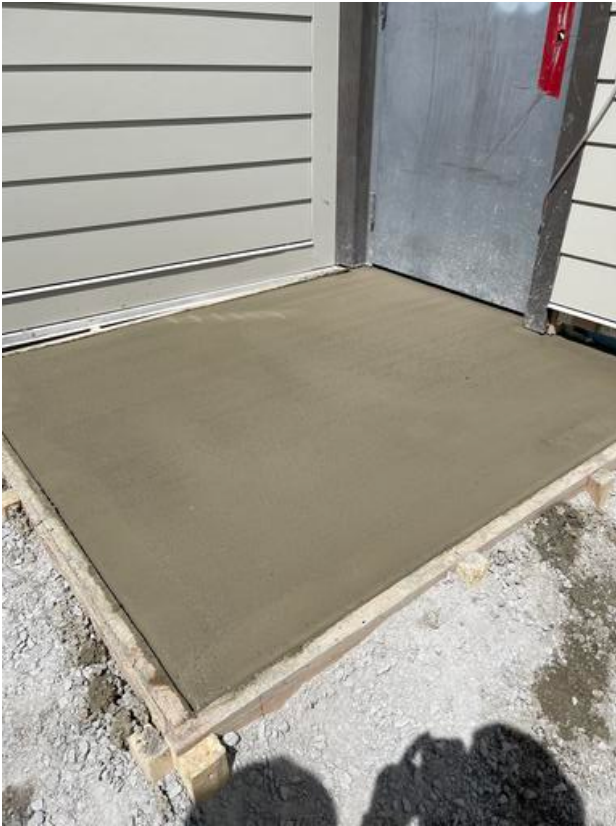
PA- Exterior Pad poured
