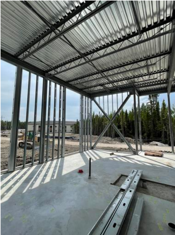
B2- Carlson framing exterior walls Arshdeep Grewal Jun 26, 2021 11:33 AM
