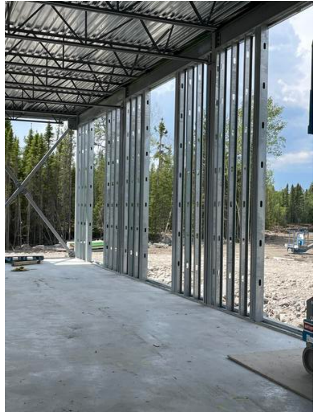
B2- Carlson framing exterior walls Arshdeep Grewal Jun 26, 2021 11:33 AM
