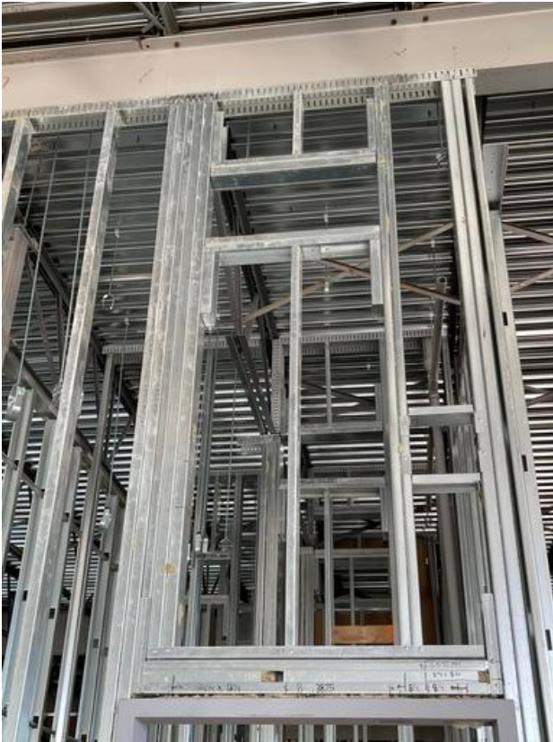
B1- Framing around openings in stud wall Arshdeep Grewal Jun 23, 2021 8:58 AM
