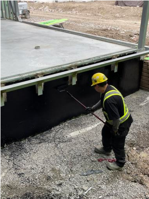
B2- Applying damp proofing coat over grade beam
