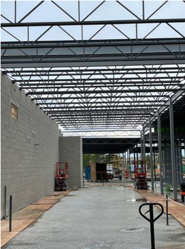
A1- Erection of roof structure
