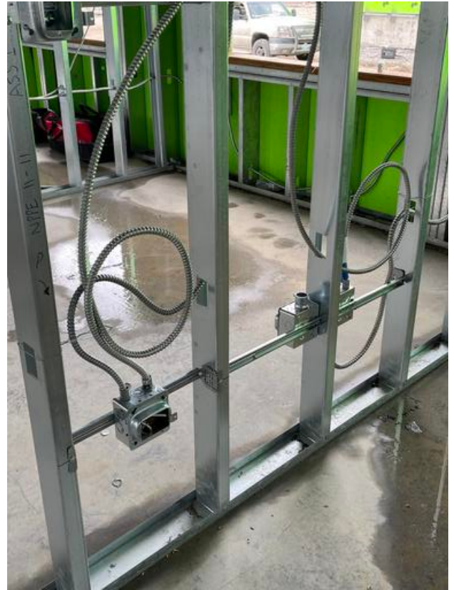
A2- Installing electrical rough ins
