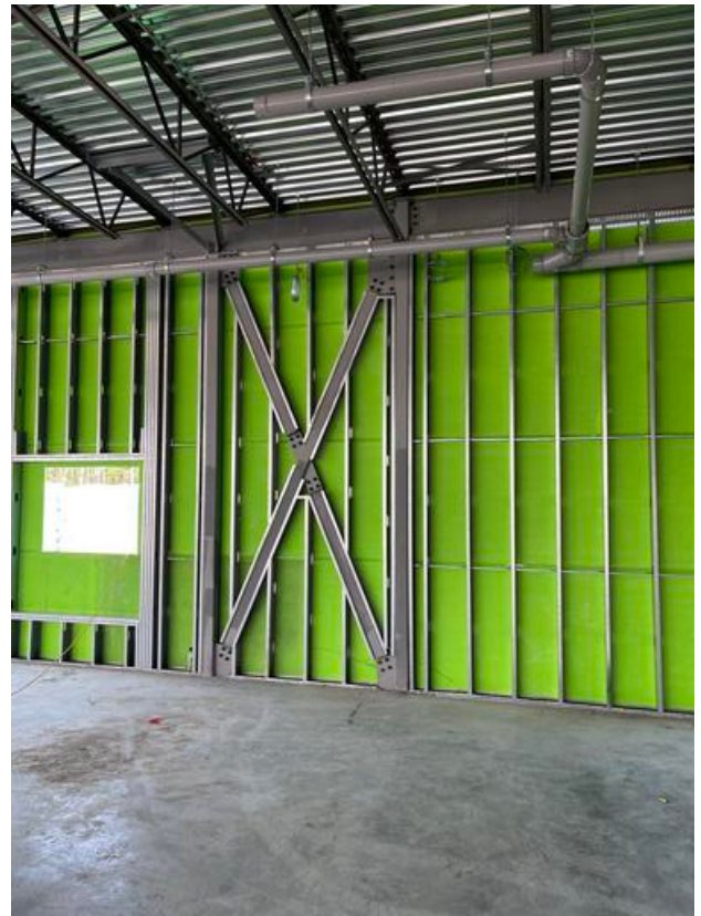
B2- Installing exterior wall sheathing
