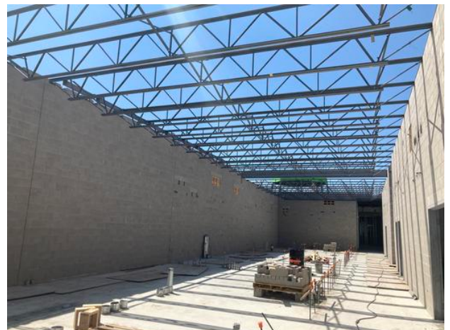
A1 steel structure over masonry Anmol Kang Jul 4, 2021 3:56 PM
