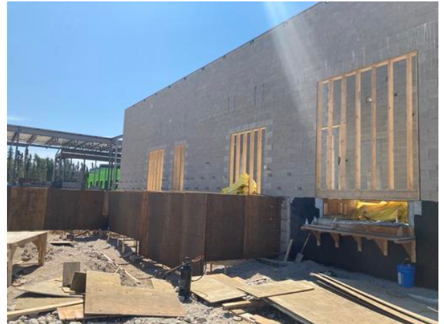
Formwork for exterior GB Loading dock
