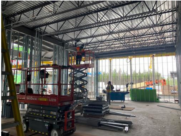
Working on conduit runs in A3
