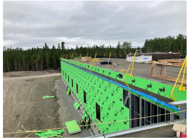
B2 exterior sheathing work in progress
