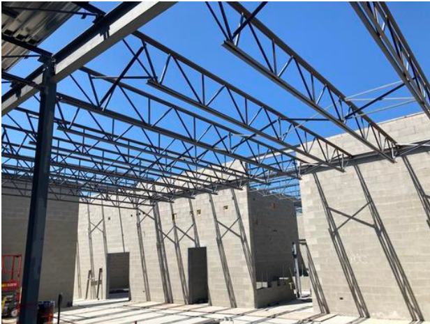
A1 steel structure over Masonry A1
