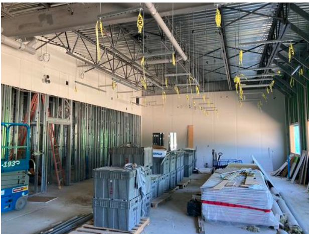
Dry wall installed in B1
