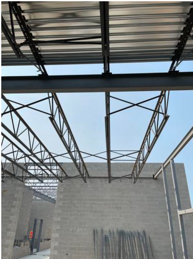
A1- Cross bracing between joist
