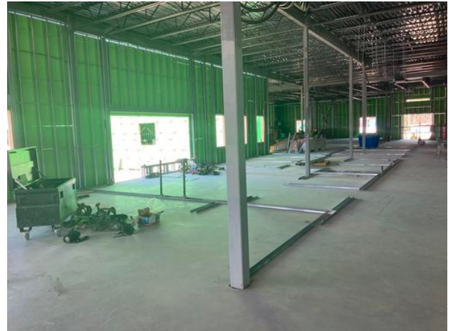
Bottom tracks laid in B1-3
