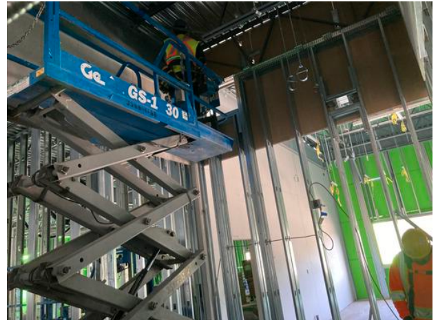
Installing drywall B1
