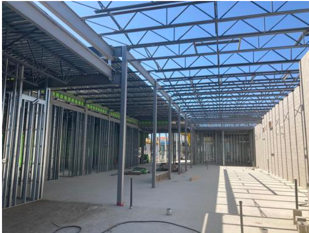
Joist over masonry wall A1
