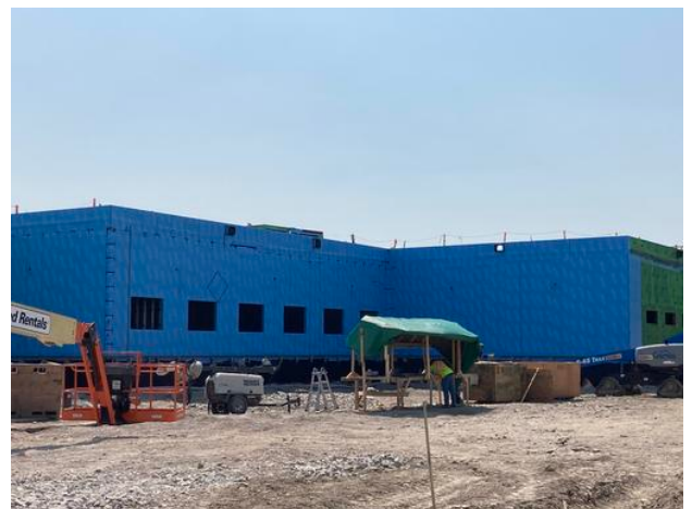
AVB installation B1 North wall Anmol Kang Jul 11, 2021 12:39 PM
