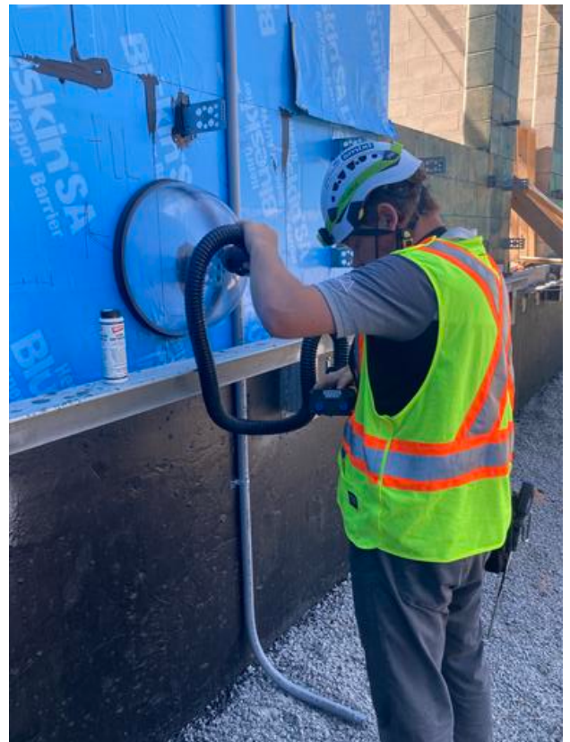
Bubble test on wall
