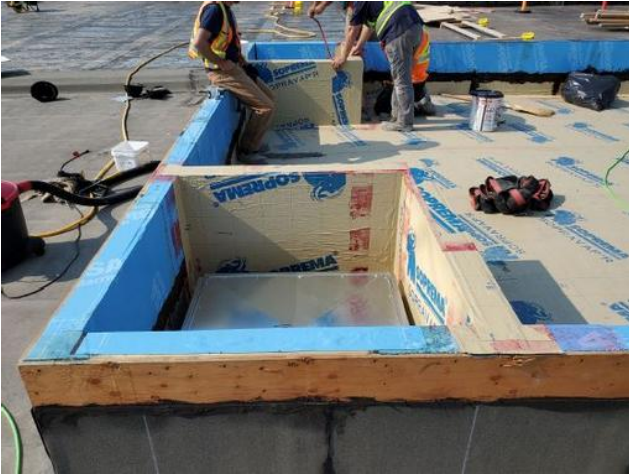
Duct work chase B1 RTU Anmol Kang Jul 15, 2021 2:42 PM
