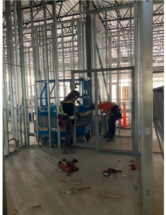
Installing door frames in B1 Anmol Kang Jul 15, 2021 2:40 PM
