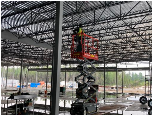
Installing hangers in C1 Anmol Kang Jul 19, 2021 4:56 PM
