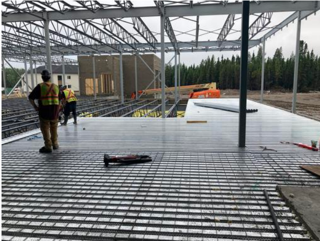
Laying deck sheets C2 main level
