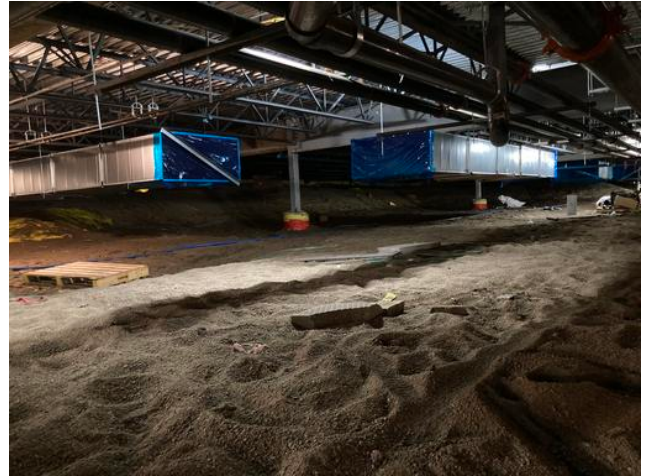
Crawlspace ducts sealed Anmol Kang Jul 17, 2021 2:23 PM
