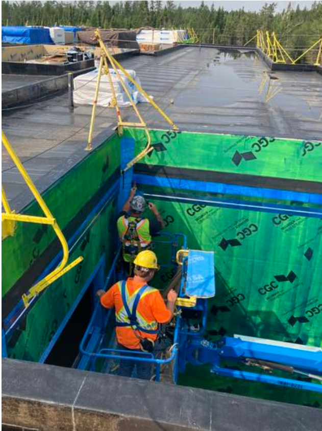
Installing AVB B2 North Anmol Kang Jul 15, 2021 2:41 PM
