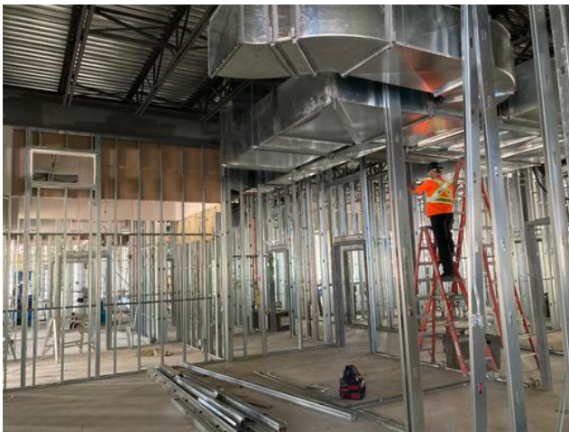
Ductwork installation in B1 Anmol Kang Jul 17, 2021 2:23 PM
