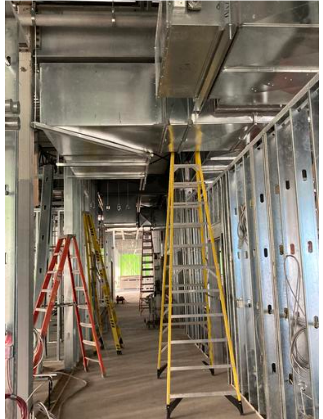
Ductwork in progress B1
