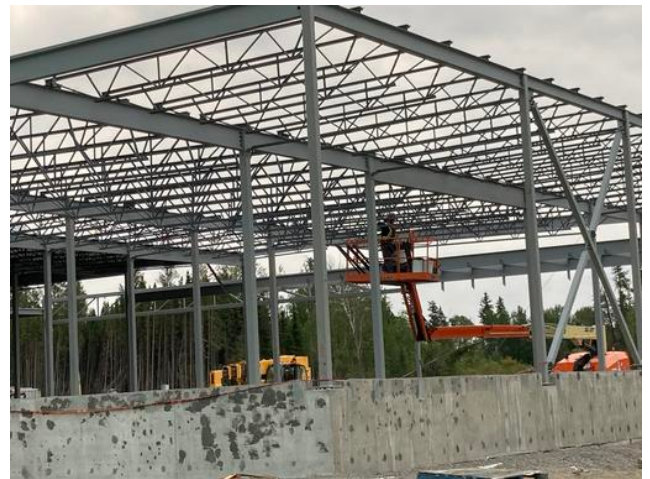
Cross bracing C2 roof level
