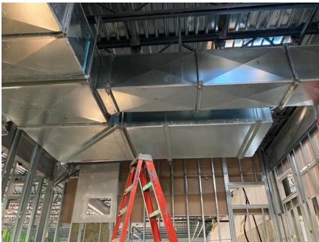
Working on ductwork in B1 Anmol Kang Jul 15, 2021 2:39 PM
