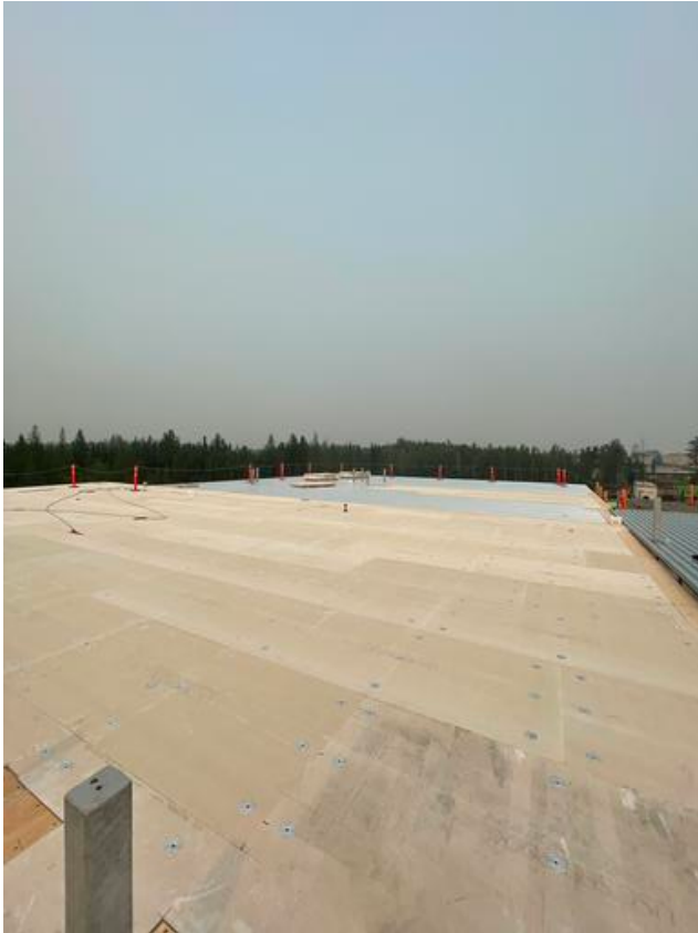
A1- Installing secure rock over Q-Deck
