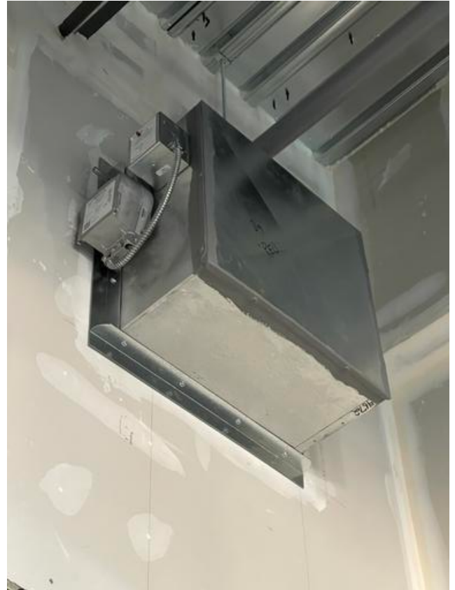
B1- Smoke dampers installed
