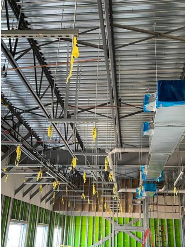
B1- Installing ductwork and water lines
