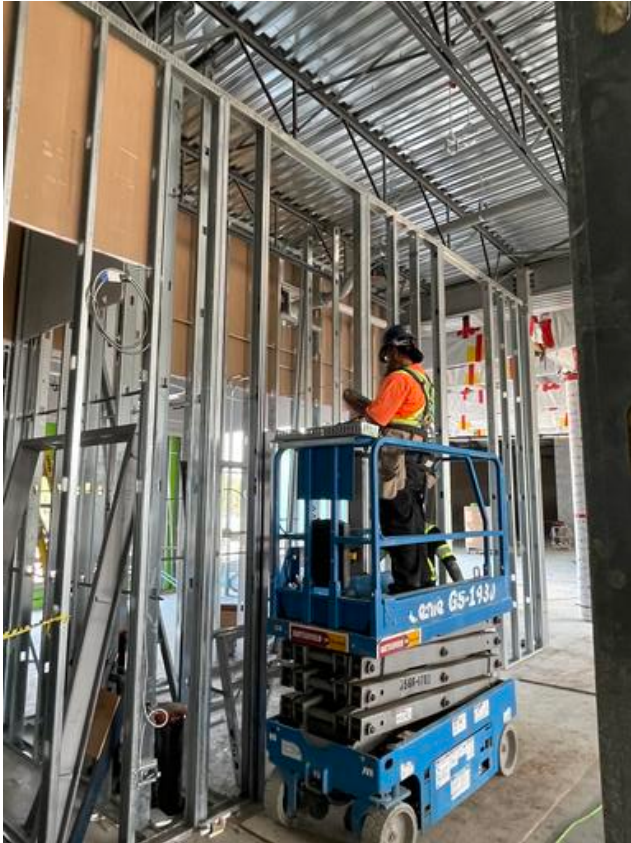
B1- Framing interior walls
