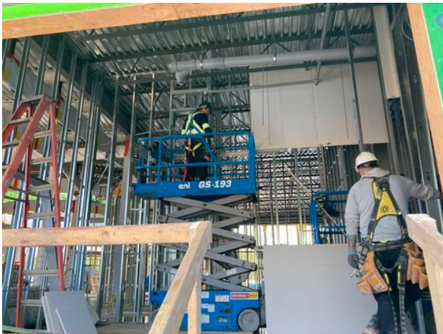
Installing drywall tops A3
