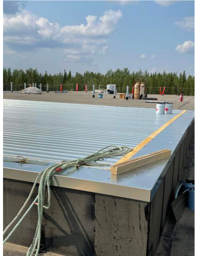
A1- Installing flashing at elevation change Arshdeep Grewal Jul 26, 2021 7:53 AM
