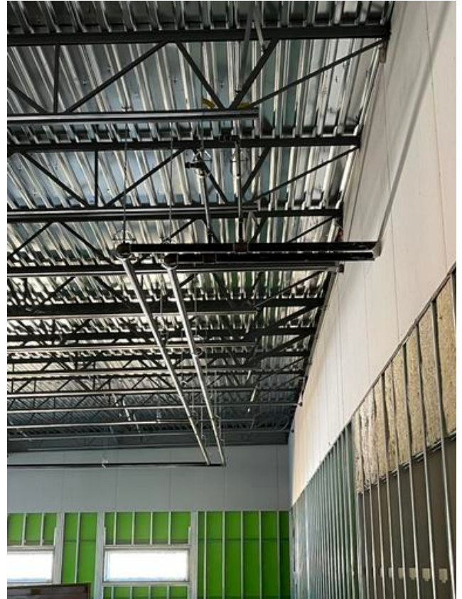
B1- Ongoing glycol lines installation
