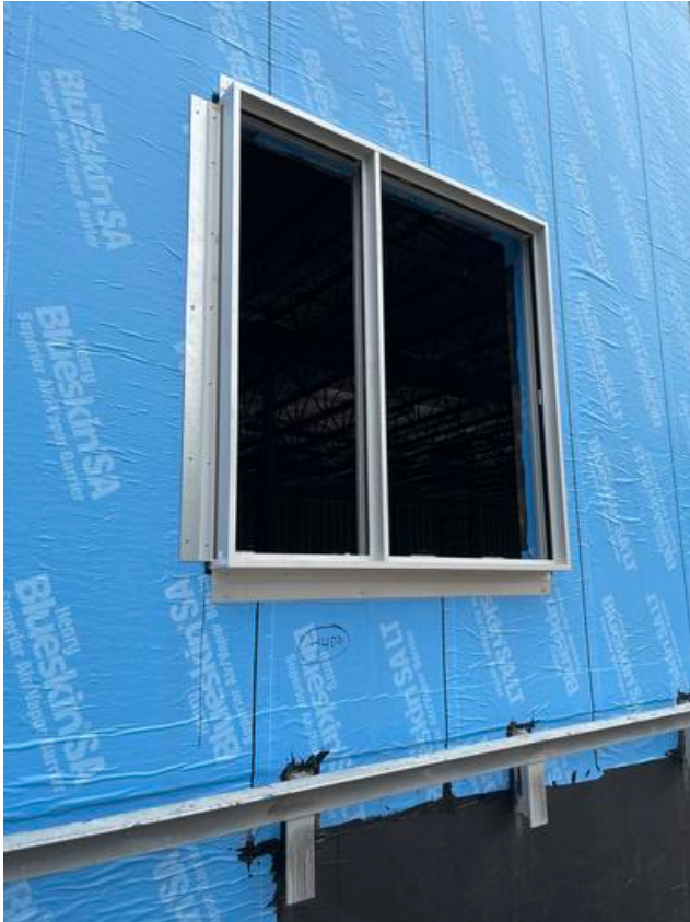
B2- Ongoing installation of window frames
