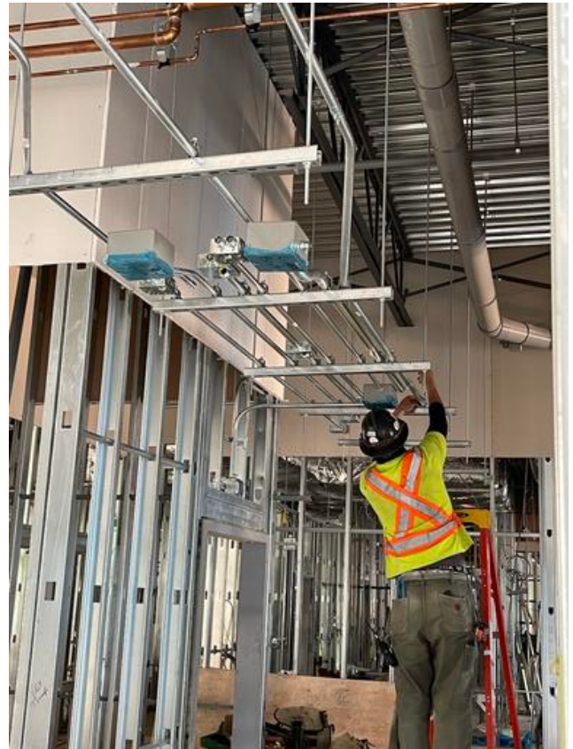
B1- Installing conduits and junction box
