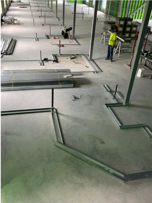
B2= Laying out interior wall Arshdeep Grewal Jul 26, 2021 7:53 AM
