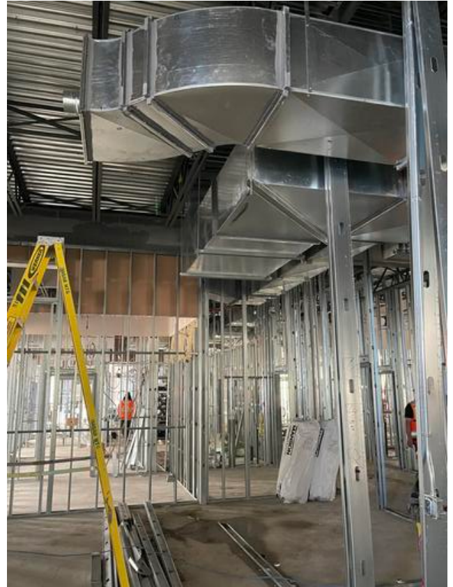
B1- Ductwork installation ongoing
