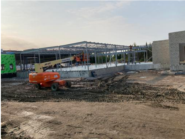
Cross bracing C2 roof level
