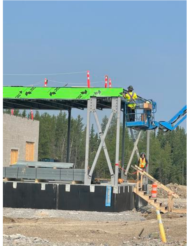
A1- Doing beam in-fills Arshdeep Grewal Jul 23, 2021 11:58 AM
