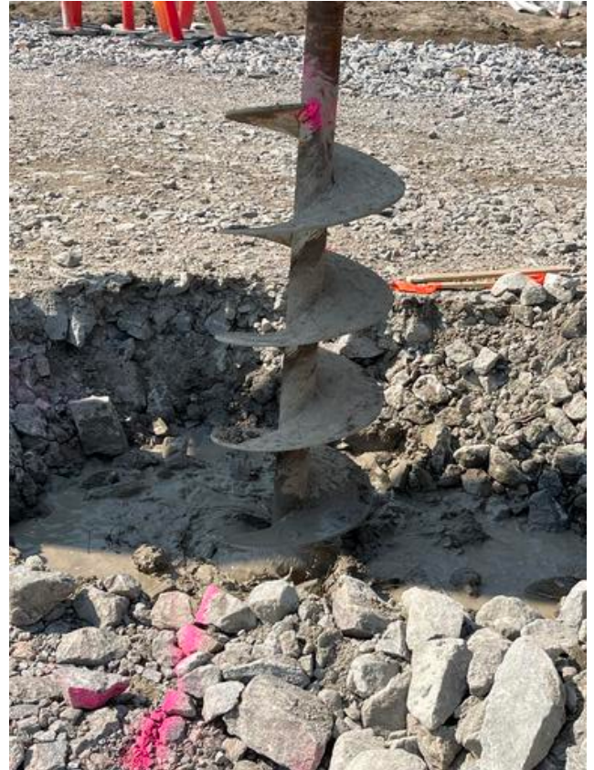
Drilling for light standards
