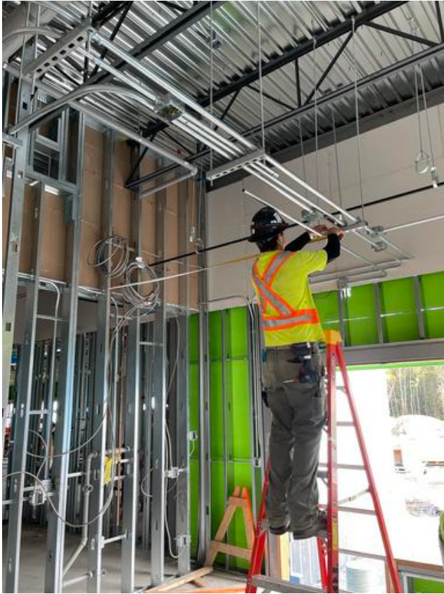
B1- Installing conduits and junction boxes
