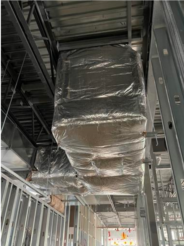
B1- Insulated ductwork Arshdeep Grewal Jul 21, 2021 2:21 PM
