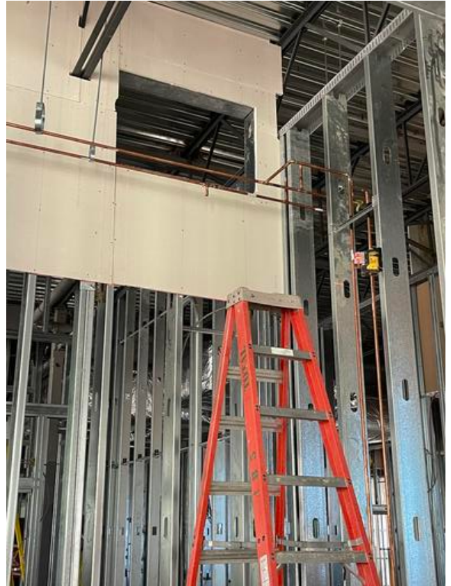
B1- Ongoing water line installation
