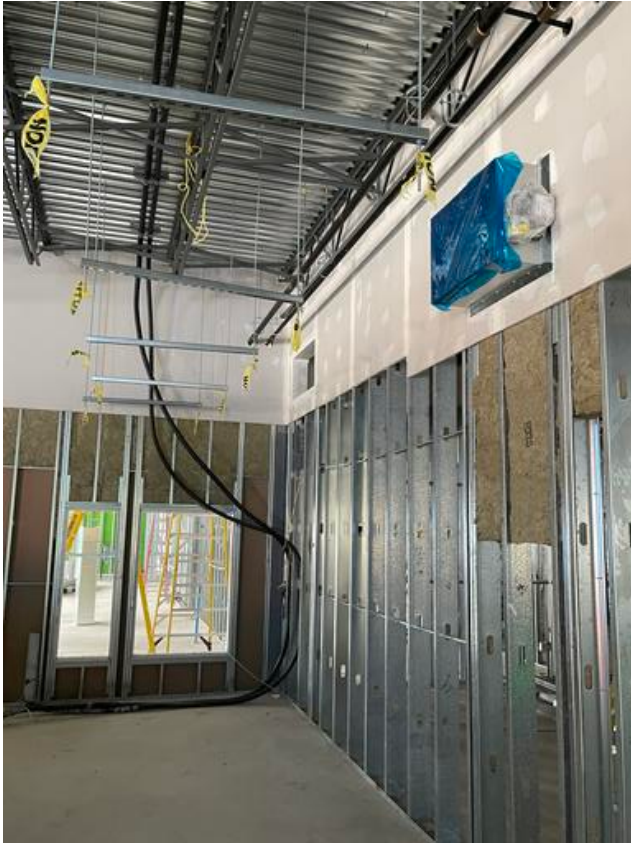
B1- Ongoing installation of drywall tops
