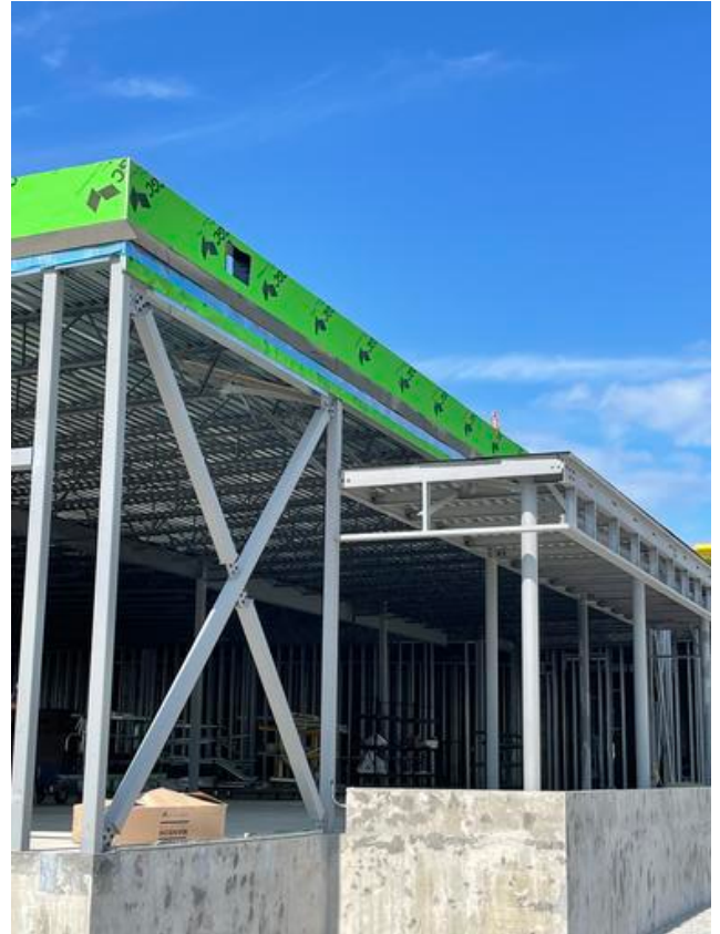
C1- Sheathing around parapet walls
