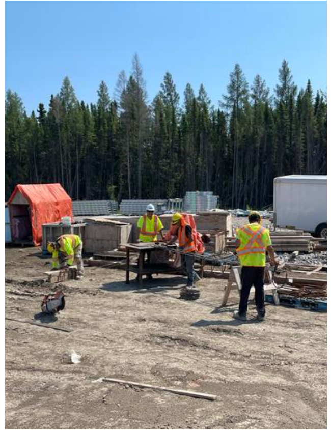
Making cages for light standard foundation
