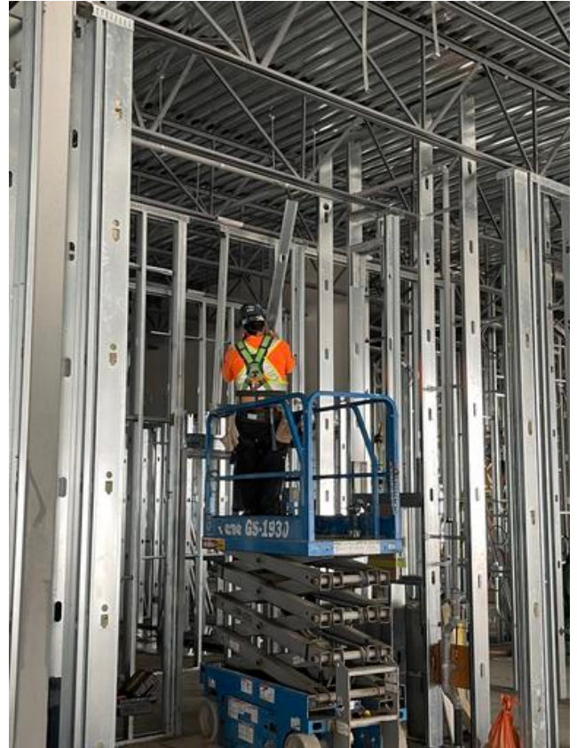
B1- Framing interior walls Arshdeep Grewal Jul 21, 2021 2:21 PM
