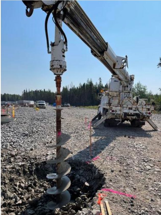
Drilling for light standards Arshdeep Grewal Jul 23, 2021 11:58 AM
