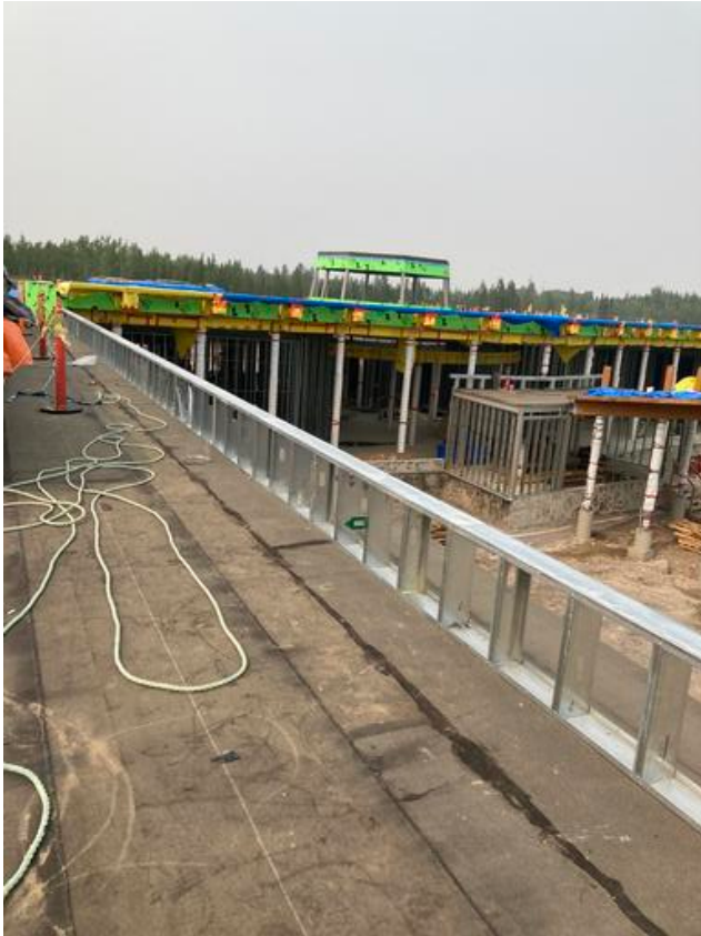
Parapet wall framing C1 roof
