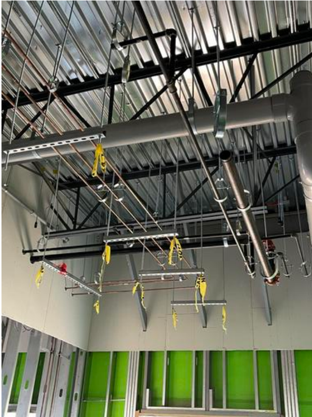
B1- Ongoing installation of plumbing systems
