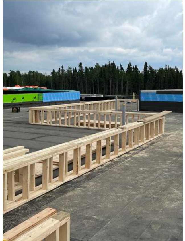
A3- Building curbs over expansion joint
