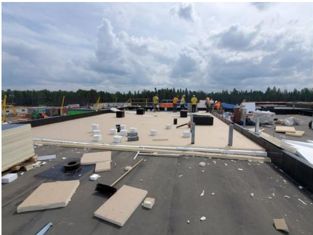
Roof insulation installation on-going
