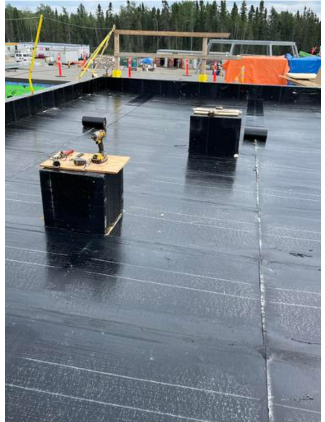
A1- Insulating around curbs
