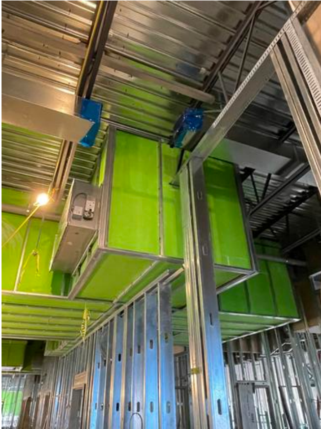
B1- Building shaft wall around ductwork Arshdeep Grewal Aug 9, 2021 3:39 PM
