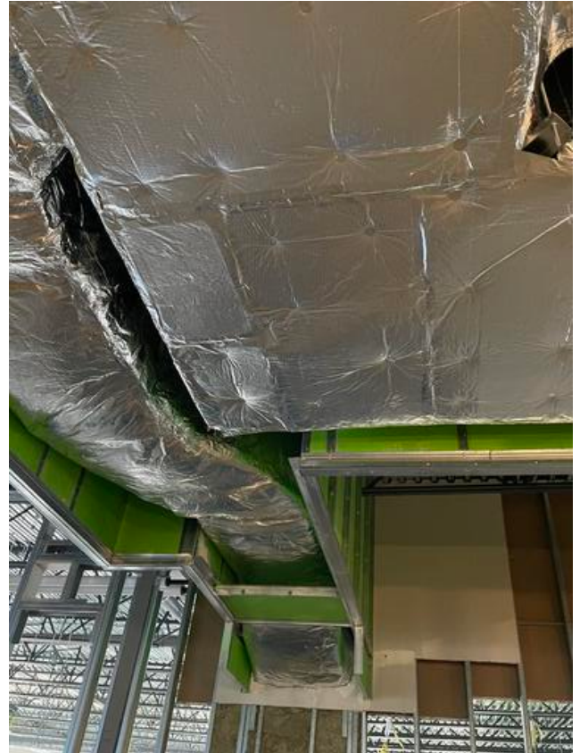
B1- Building shaft wall around ductwork Arshdeep Grewal Aug 9, 2021 3:39 PM
