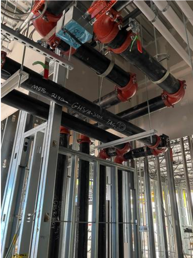
B1- Installed hydronic pipes
