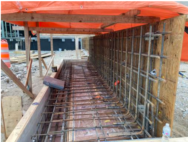
Rebar detail loading dock GB
