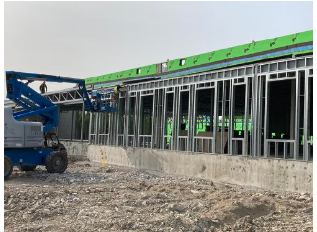
Working on exterior framing C1
