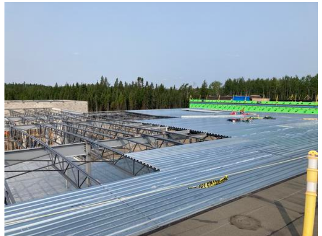
Installing deck C2 roof
