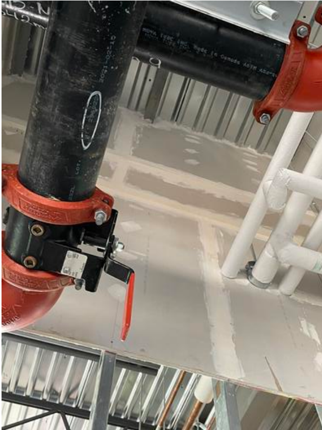
B1- Drywall installed to the flutes for rated wall Arshdeep Grewal Aug 9, 2021 3:39 PM
