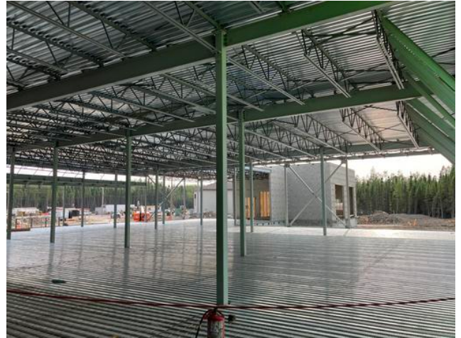
C2 roof deck complete
