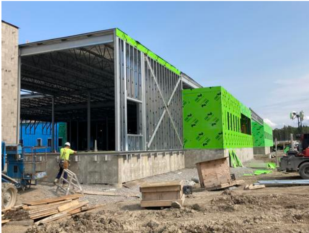
Exterior sheathing work on-going C2 Anmol Kang Sep 3, 2021 3:15 PM
