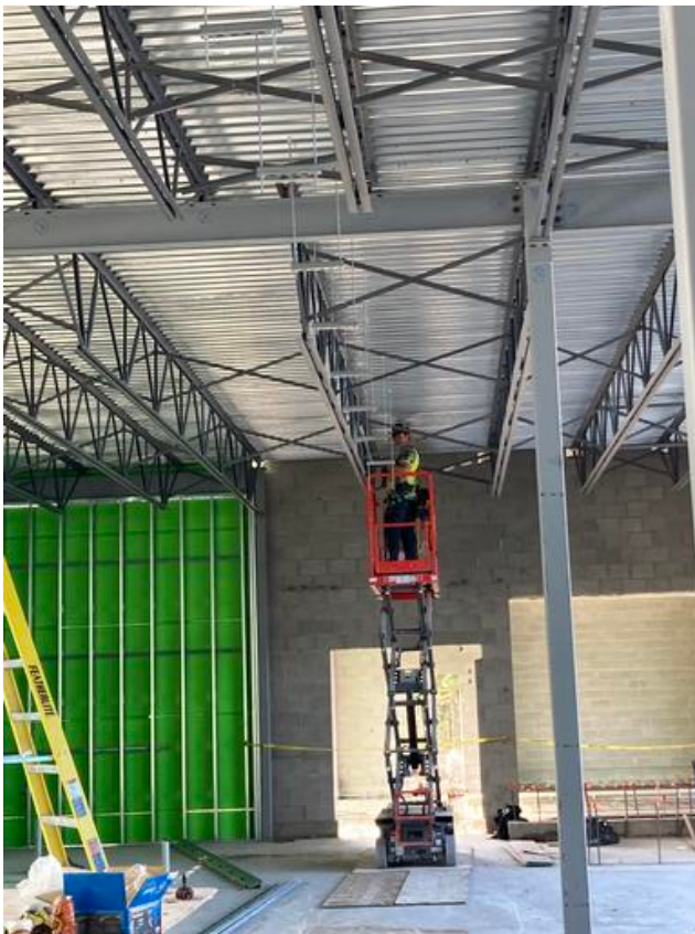
Installing hangers in C2
