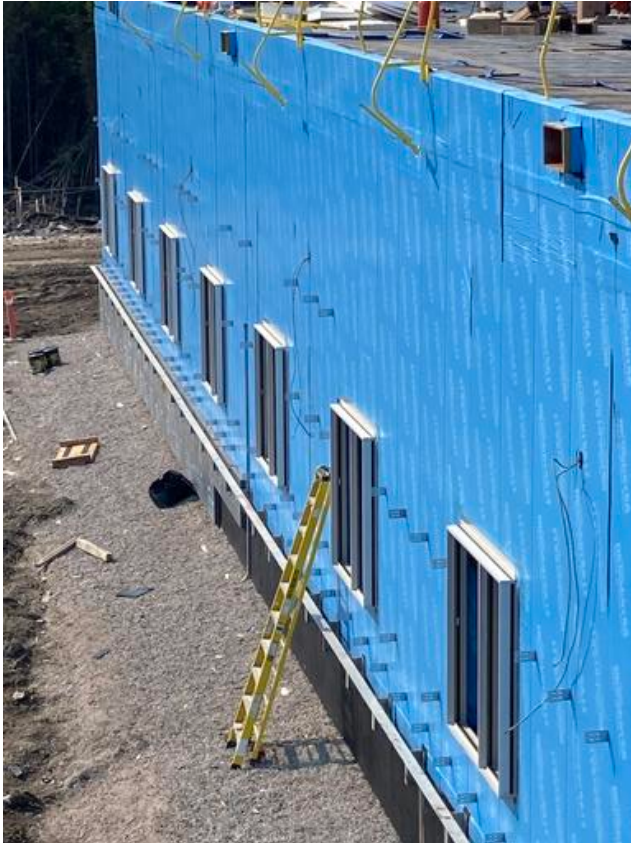
Brick clips installed B2 South wall
