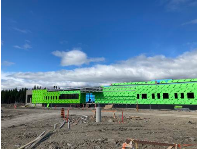
Exterior sheathing C1 and C2 Anmol Kang Sep 6, 2021 1:41 PM
