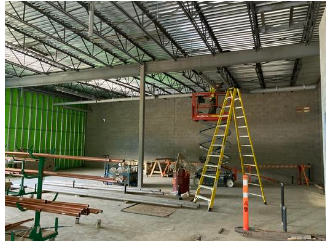
Installing hangers in A1
