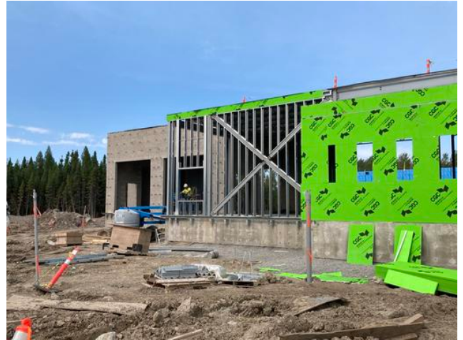
Exterior sheathing work on-going Anmol Kang Sep 3, 2021 3:15 PM
