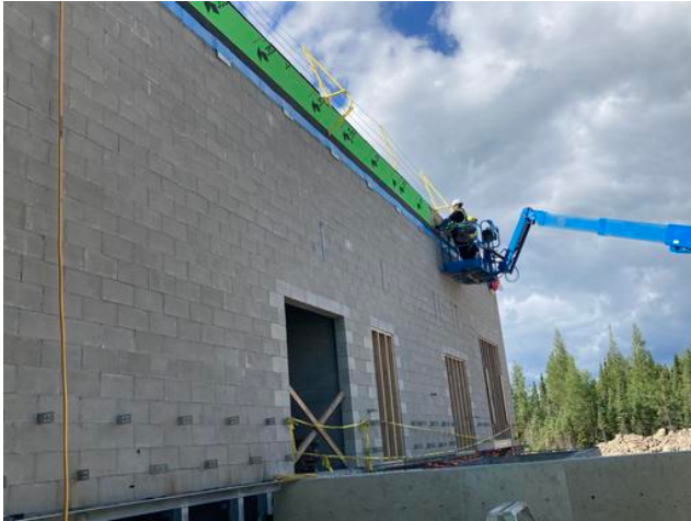
Exterior sheathing on parapet walls B1
