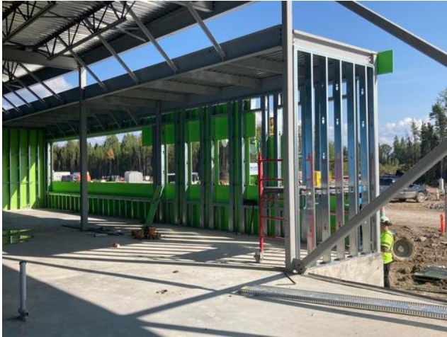
Exterior sheathing work on going C2
