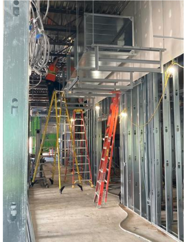
Ductwork on going B1
