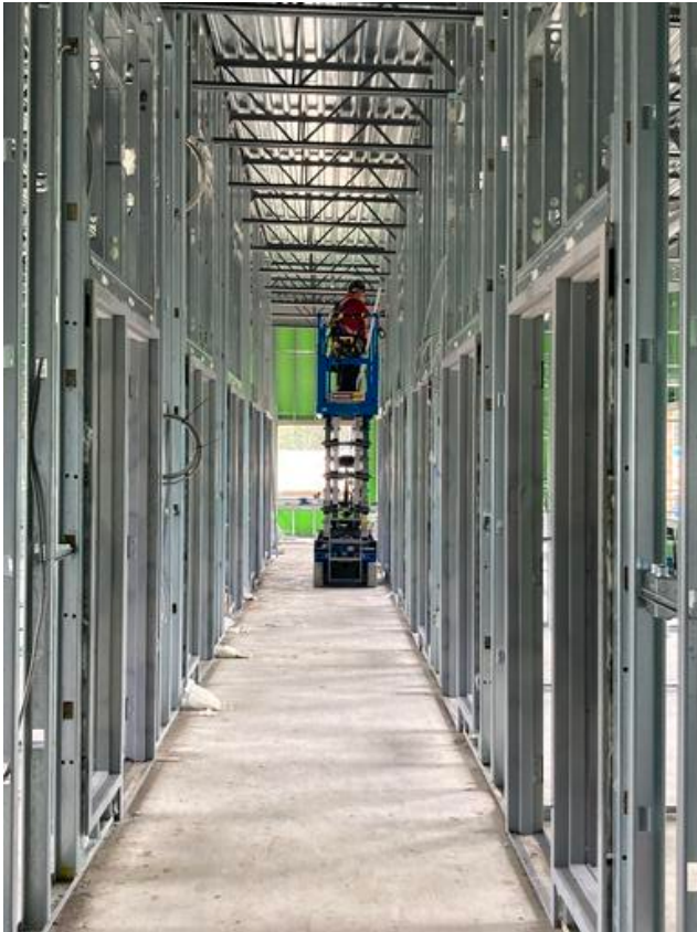
Installing door headers in A2
