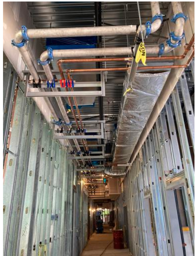
Water mains installed B1 corridor
