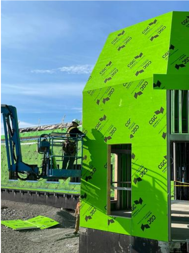
A2- Sheathing exterior wall on quiet room
