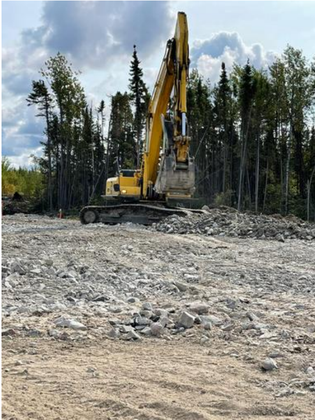
Spreading rock on southwest parking lot
