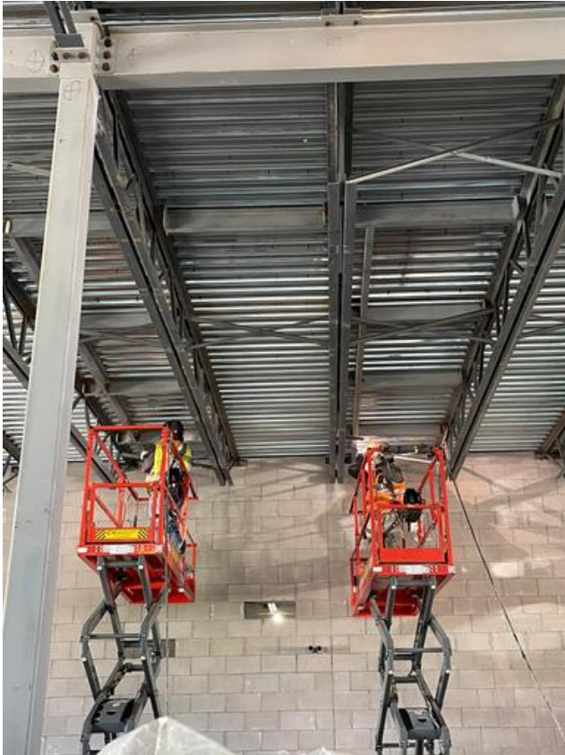
A1- Installing RTU supports
