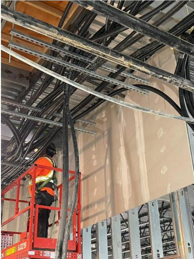
B1- Installing feeder cables
