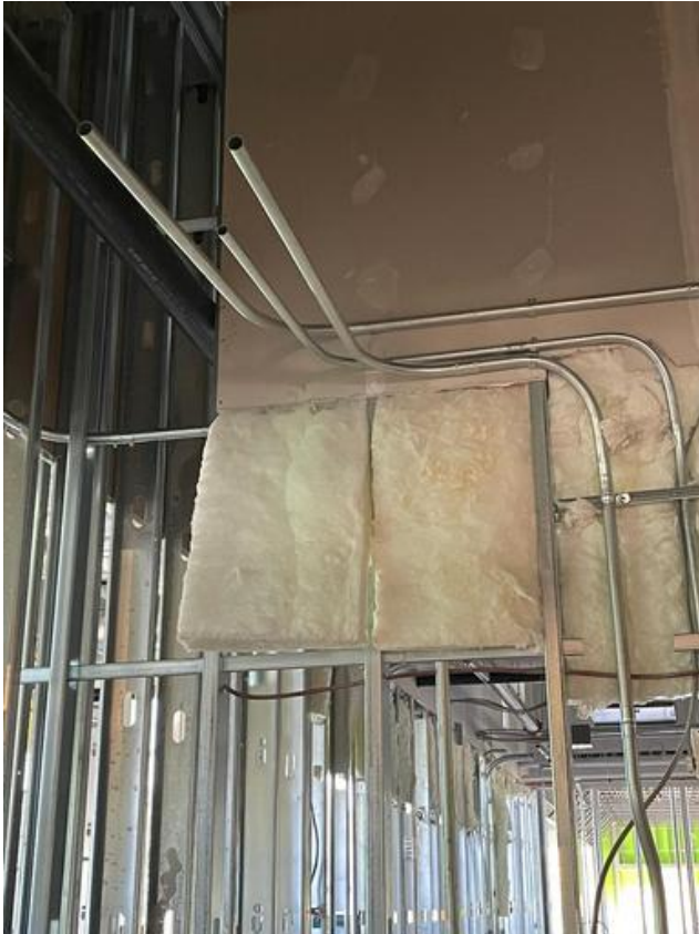
B1- Installing conduits Arshdeep Grewal Sep 12, 2021 5:39 PM
