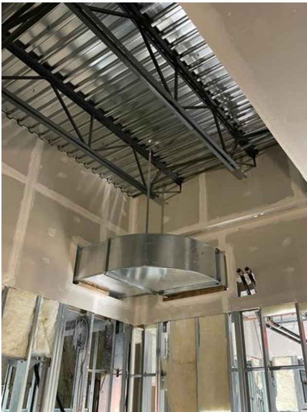
Mech Duct work install Arshdeep Grewal Sep 14, 2021 5:34 PM
