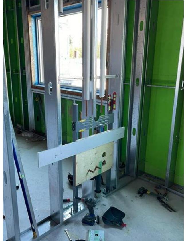
B1- Installing lav carrier Arshdeep Grewal Sep 12, 2021 5:39 PM
