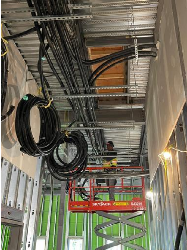
B1- Installing feeder cables Arshdeep Grewal Sep 13, 2021 4:37 PM
