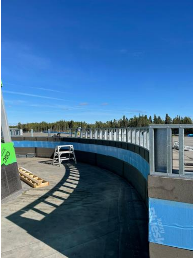
A3- Framing parapet walls Arshdeep Grewal Sep 12, 2021 5:39 PM
