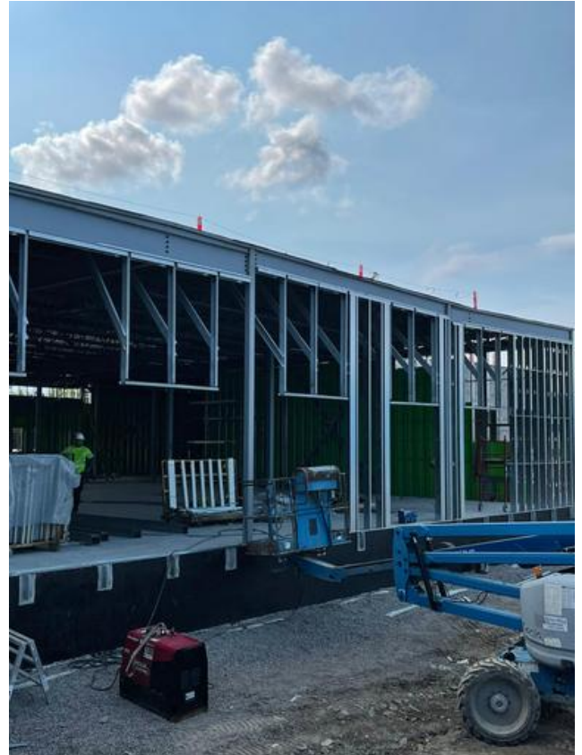
C2- Framing exterior wall
