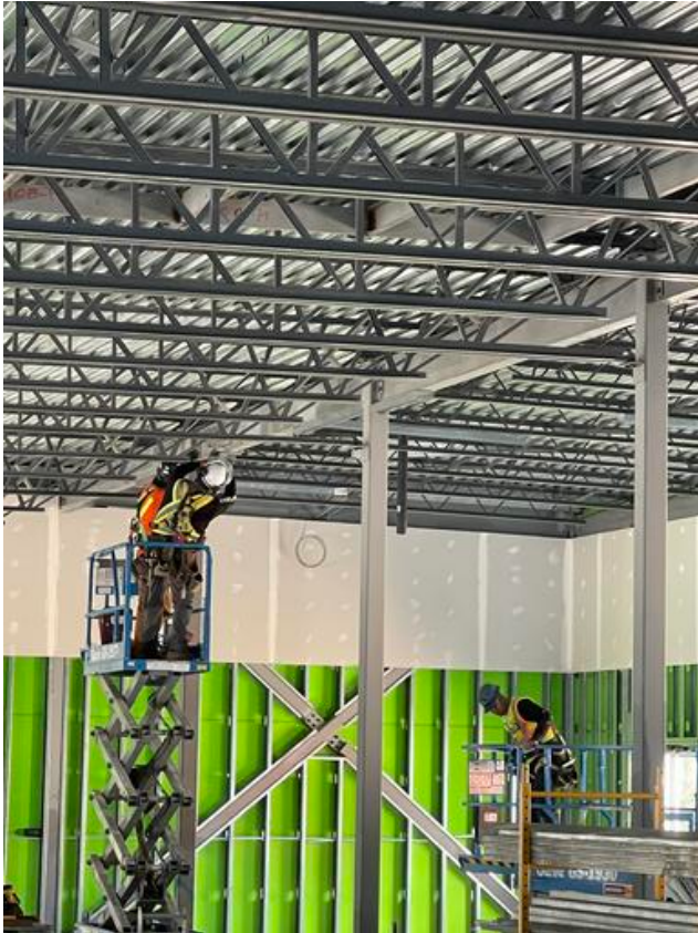
B2- Installing top tracks
