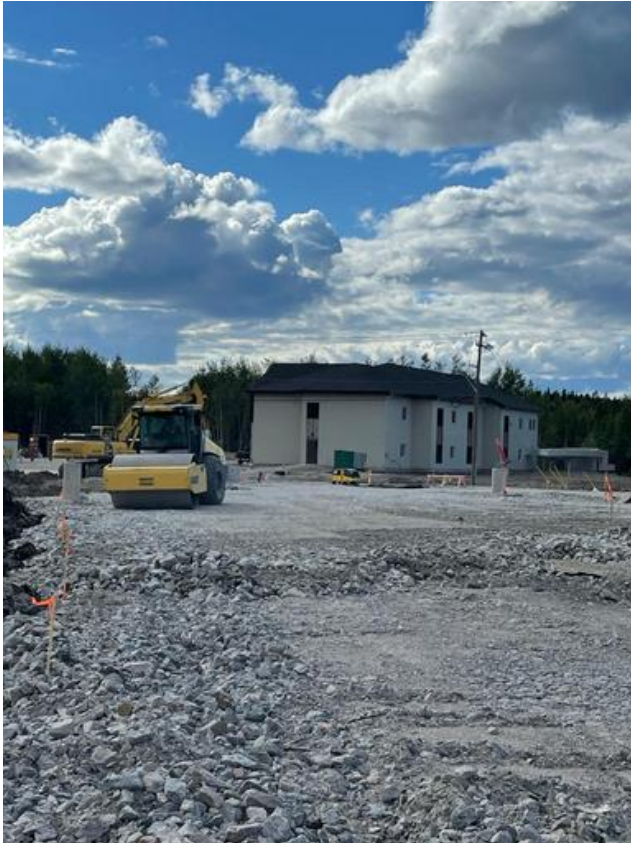
Placing & compacting rock @Southwest parking lot
