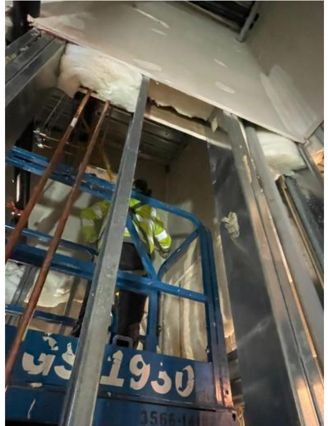
B1- Installing drywall tops
