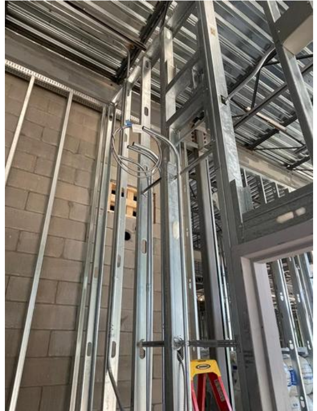
A3- Ongoing installation of electrical rough ins Arshdeep Grewal Sep 12, 2021 5:39 PM
