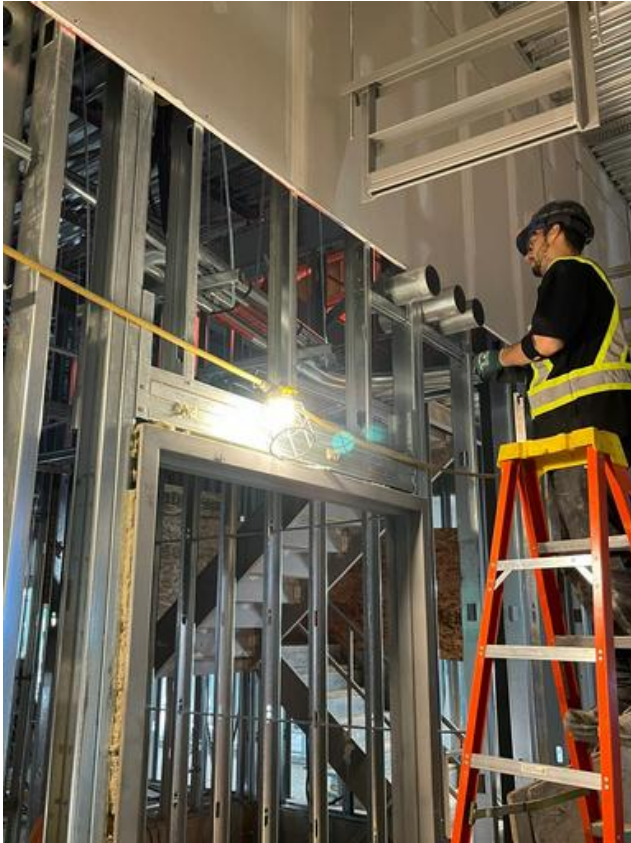
B1- Installing sleeves Arshdeep Grewal Sep 11, 2021 7:57 PM
