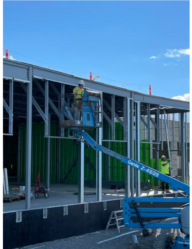
C2- Framing & sheathing exterior wall
