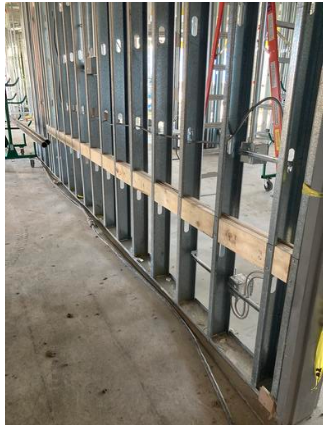
Hand rail backing in B1 Anmol Kang Oct 19, 2021 4:35 PM
