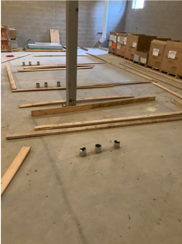
Working on housekeeping pads
