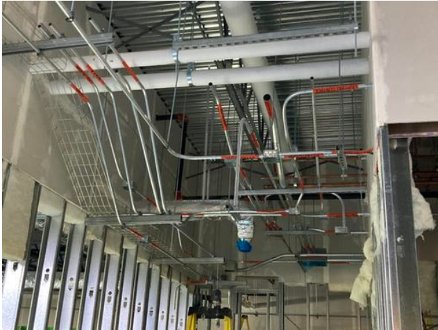
Installing electrical conduit in B1 Anmol Kang Oct 21, 2021 1:42 PM
