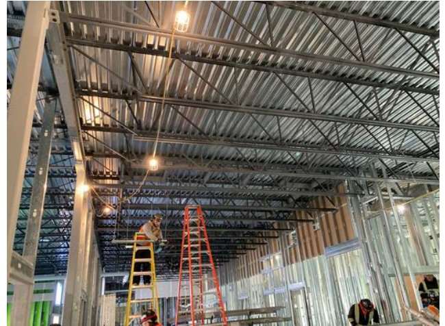
Installing hangers in B2 Anmol Kang Oct 20, 2021 1:22 PM
