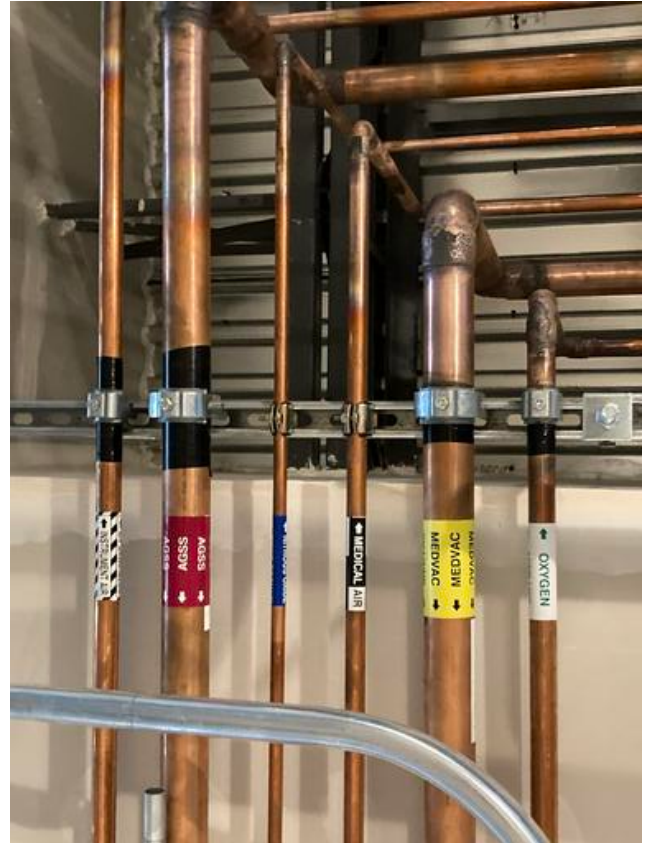
Pipes with marking B1 corridor
