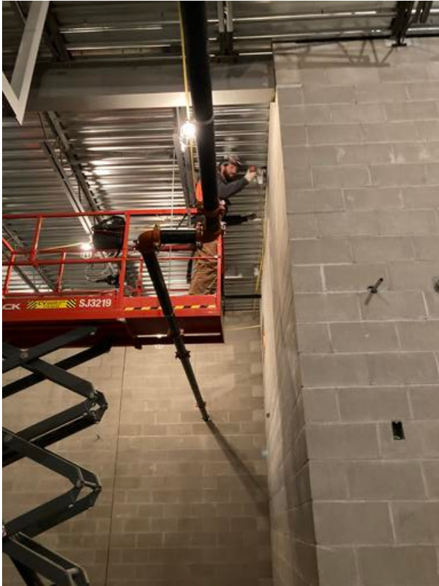
Installing sprinkler pipes in A1
