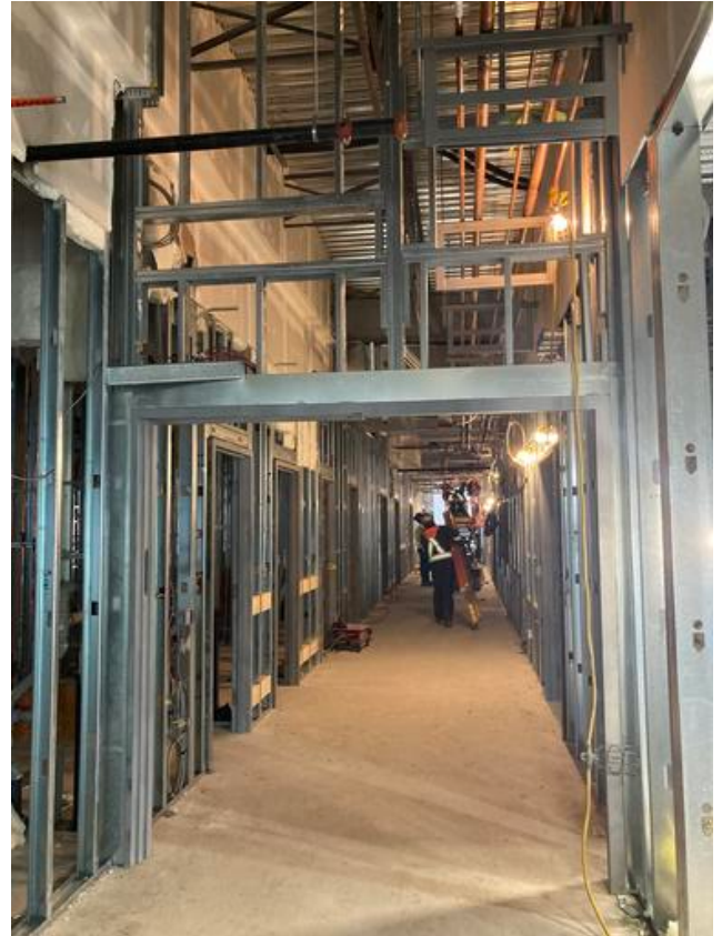
B1 corridor door frame installed
