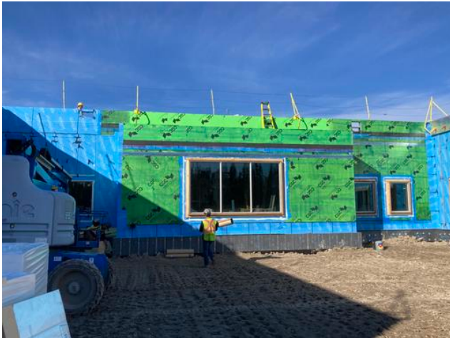
Installing AVB in A2 Anmol Kang Oct 19, 2021 4:45 PM
