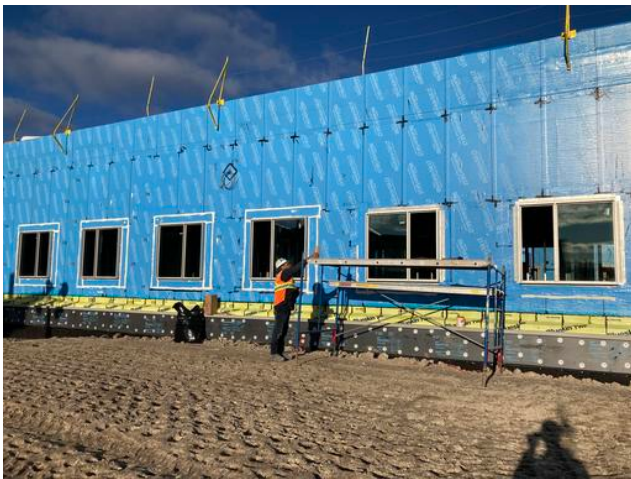
Installing blue skin around windows Anmol Kang Oct 20, 2021 1:13 PM
