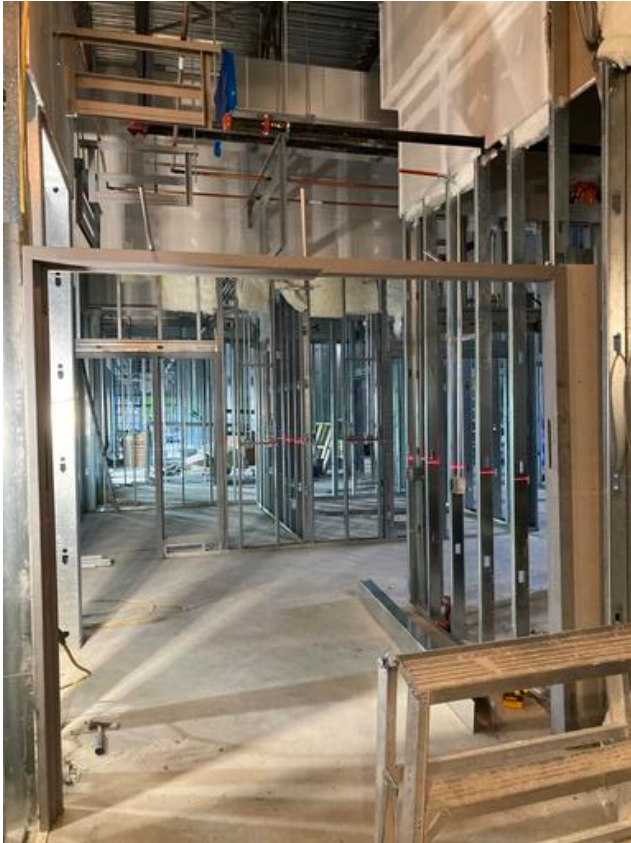
Door frame installed in B1
