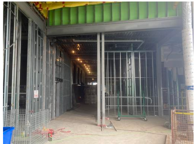
A1/A2- Interior steel stud progress Arshdeep Grewal Nov 2, 2021 7:04 AM
