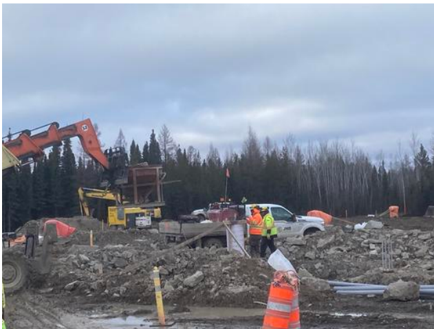
Pouring light standards in east parking lot Arshdeep Grewal Nov 2, 2021 7:04 AM
