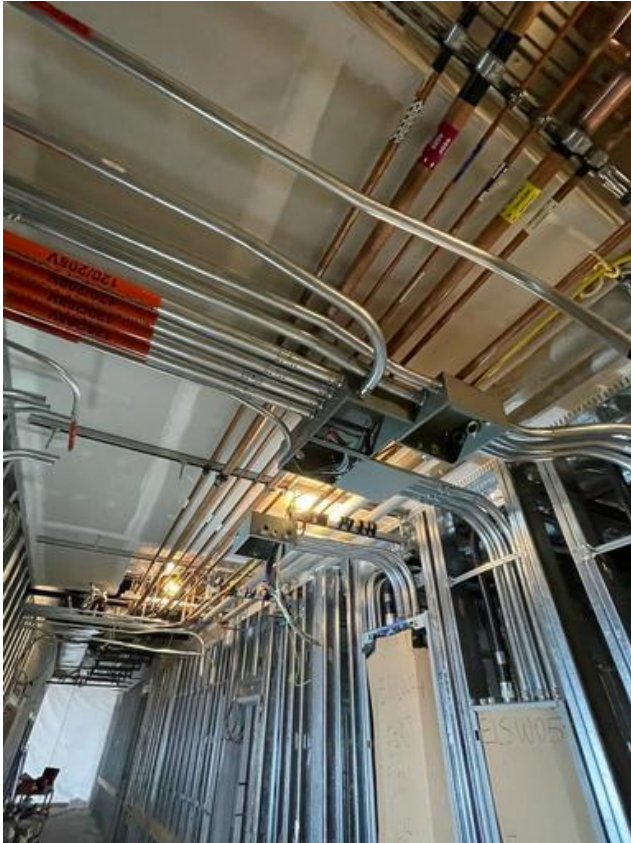
B1- Installing conduits & junction boxes
