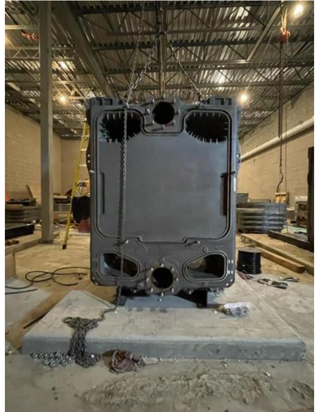
A1- Installing boilers in mechanical room
