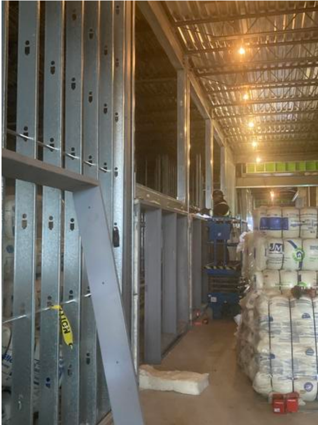
A1/A2 - Framing interior walls Arshdeep Grewal Nov 2, 2021 7:04 AM
