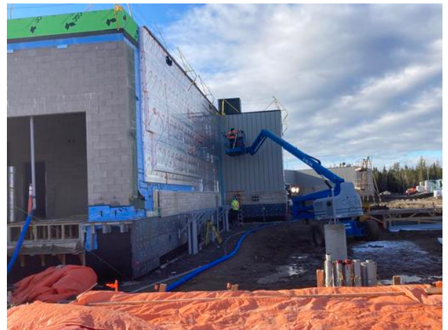
Installing cladding A1 North Anmol Kang Oct 31, 2021 6:47 AM
