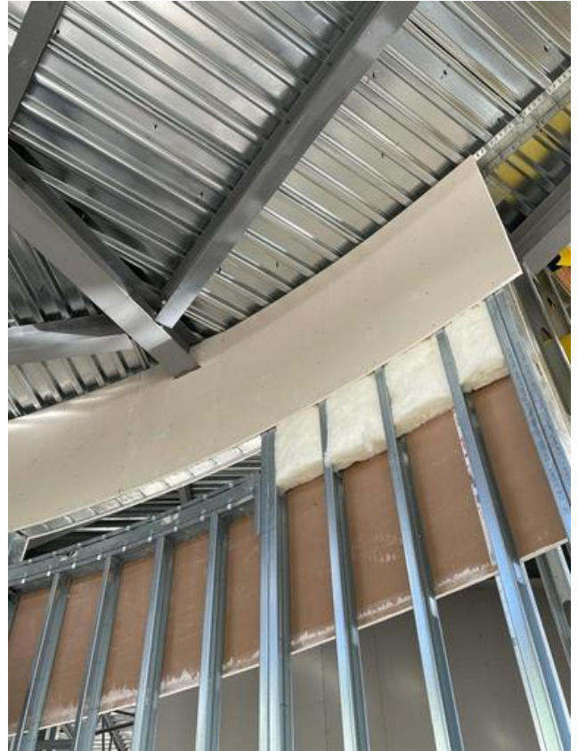
A3- Installing drywall tops Arshdeep Grewal Nov 4, 2021 4:46 PM
