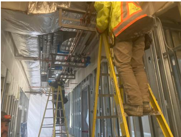
B1- Installing medical lines Arshdeep Grewal Nov 2, 2021 7:04 AM
