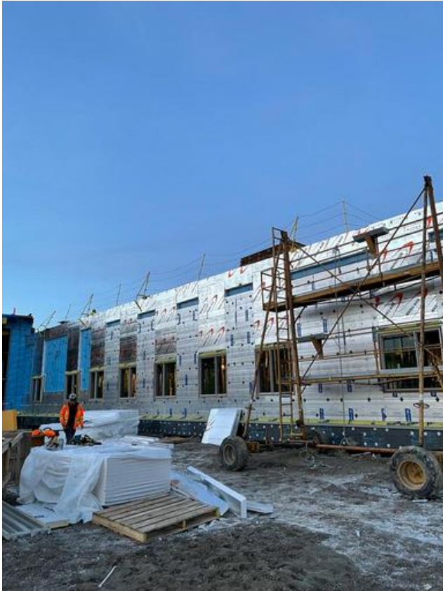
A2- Installing insulation over exterior wall
