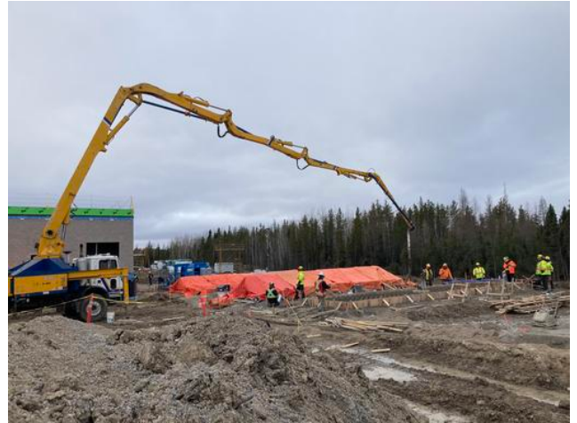
Pouring concrete pad in tank farm Arshdeep Grewal Nov 2, 2021 7:04 AM
