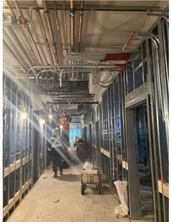
Working on domestic water mains
