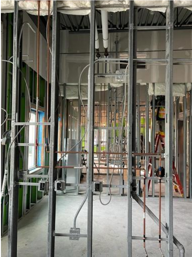
A2- Electrical in wall rough in Arshdeep Grewal Nov 2, 2021 4:14 PM
