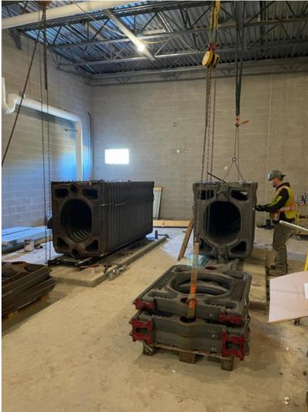
A1- Installing boilers in mech room Arshdeep Grewal Nov 3, 2021 4:19 PM
