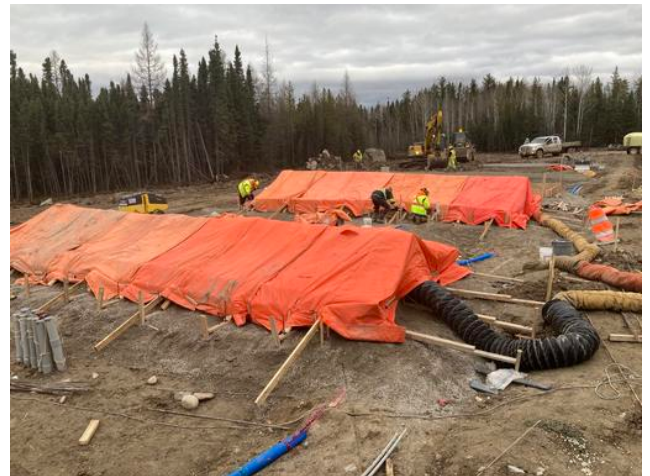
Generator pads hoarded after pour
