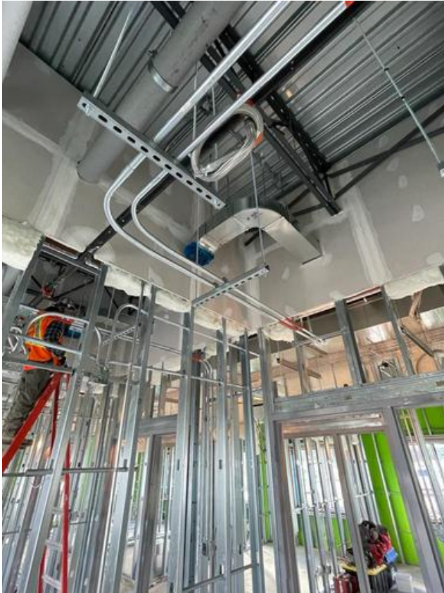
A2- Installing ductwork Arshdeep Grewal Nov 4, 2021 4:46 PM
