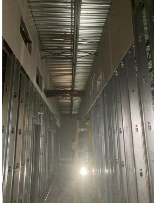
A1- Installing drywall tops Arshdeep Grewal Nov 2, 2021 7:04 AM
