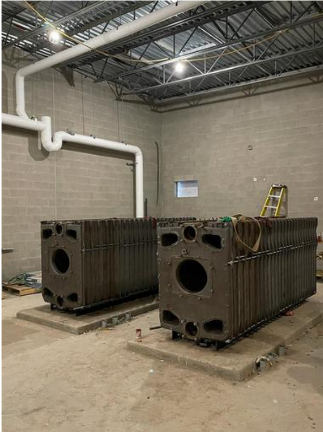
A1- Installing boilers in mech room Arshdeep Grewal Nov 4, 2021 4:46 PM
