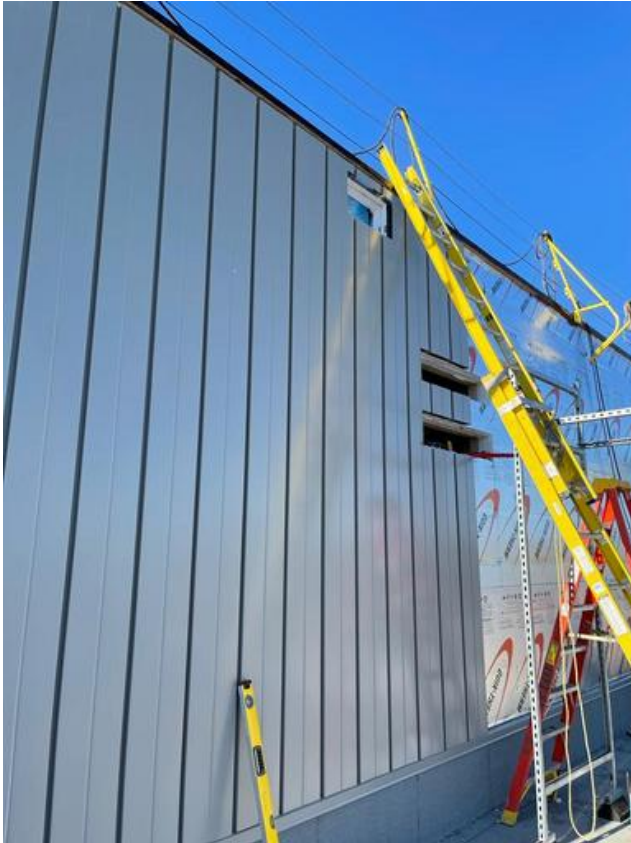
B1- Installing cladding around penthouse
