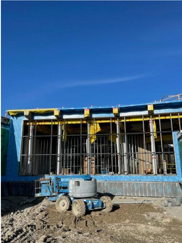
A3- Installing curtain wall
