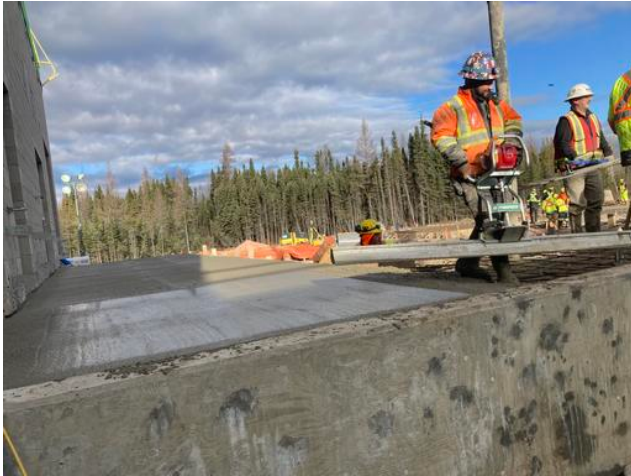
Loading dock area slab work in progress
