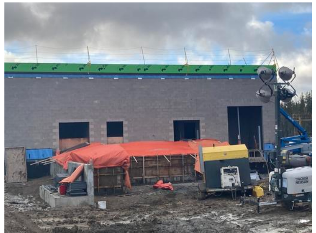
Loading dock slab hoarded and heated
