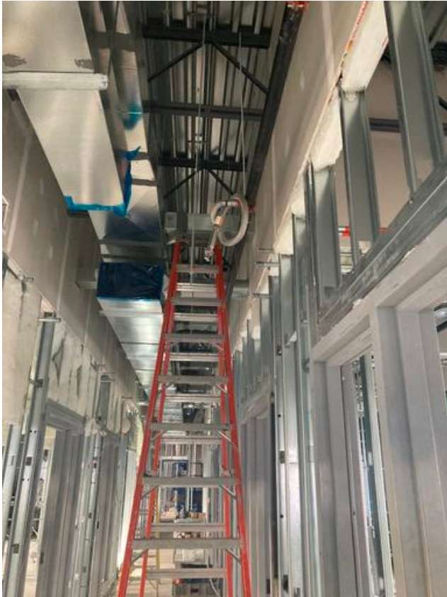
Ductwork installation on going A2
