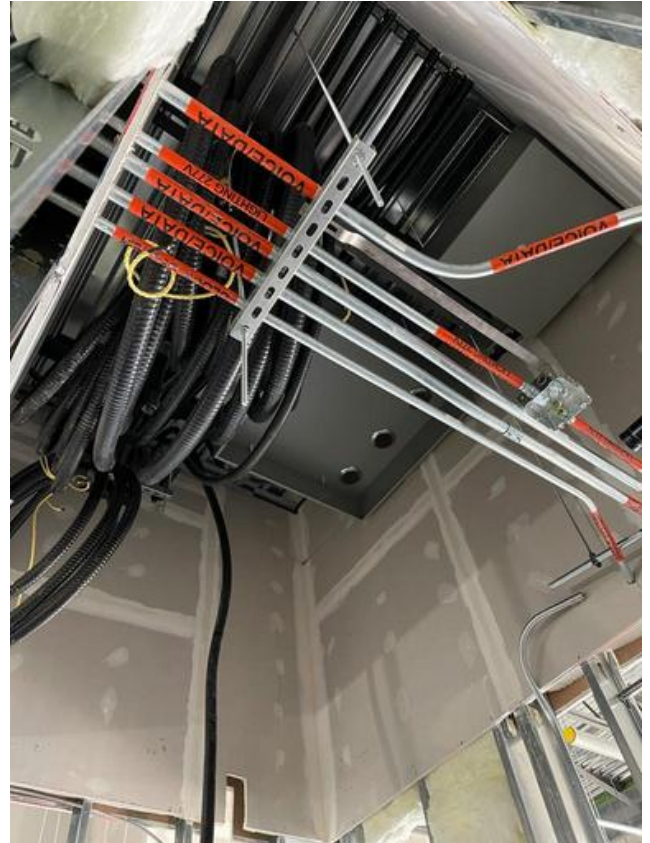
B1- Main floor panel feeders install Arshdeep Grewal Nov 3, 2021 4:19 PM
