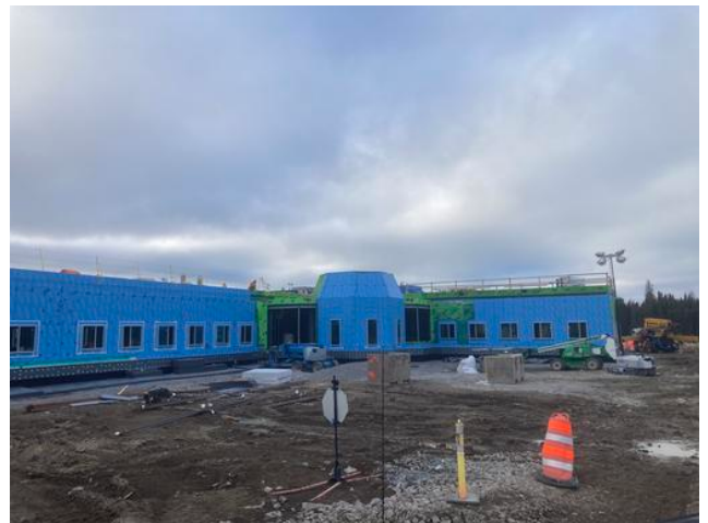
A1/A2- Installing AVB over exterior wall Arshdeep Grewal Nov 2, 2021 7:04 AM
