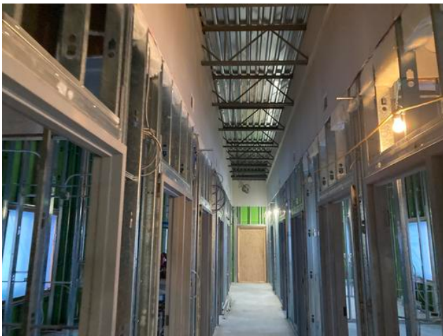
Dry wall tops installed in A1
