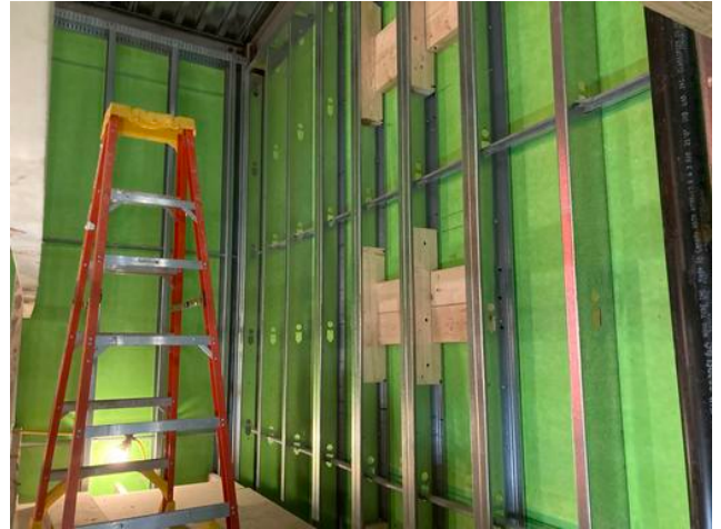
Backing done for stairs in B1
