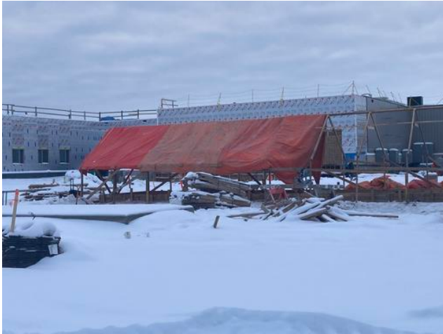
Hoarding setup for propane pad
