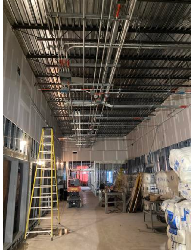
Rough in work on going A2
