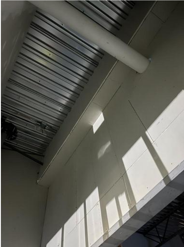
B2- Installing drywall tops Arshdeep Grewal Dec 6, 2021 5:26 PM
