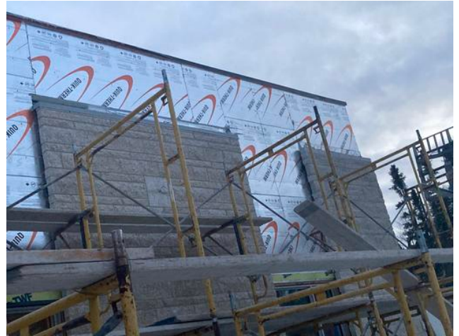
Flasing over masonry
