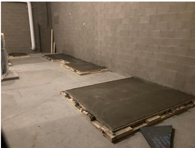
Pads poured in mech room A1 Anmol Kang Dec 2, 2021 5:12 PM
