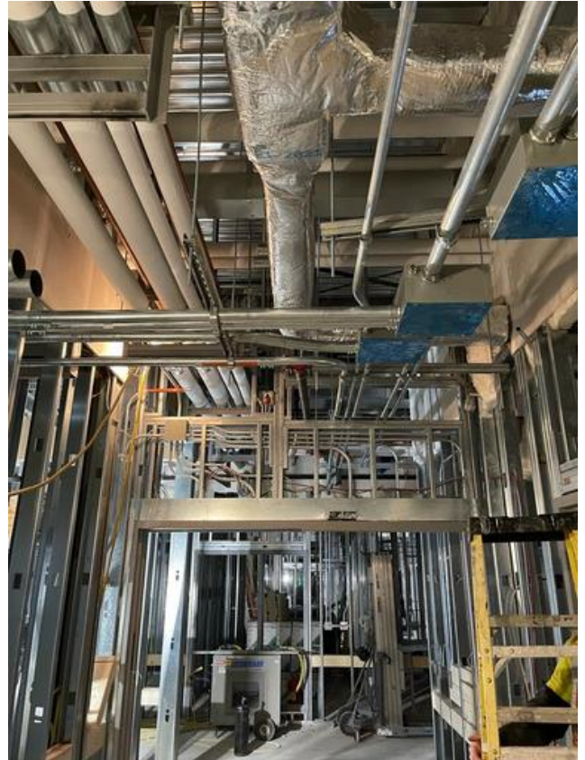
B1- Installing conduits & junction boxes Arshdeep Grewal Dec 6, 2021 5:26 PM
