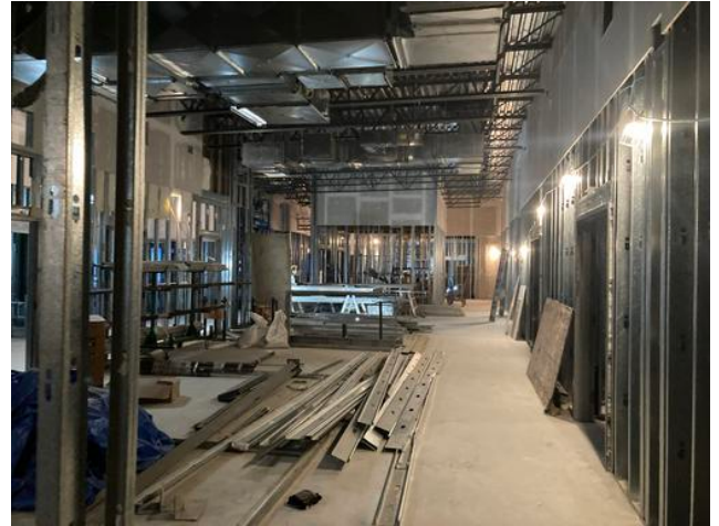
B2 interior framing Anmol Kang Dec 2, 2021 5:12 PM
