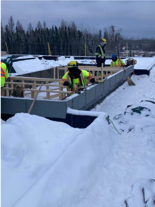
Working on RTU curb C1 roof Anmol Kang Dec 2, 2021 5:14 PM
