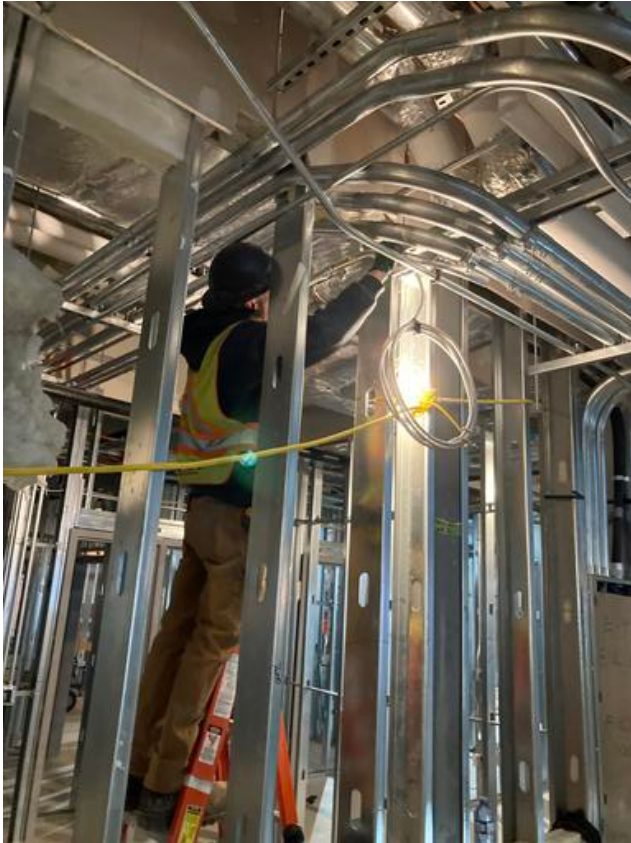
Rough in work on going in B1
