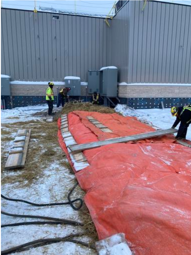
Heating ground for trenching
